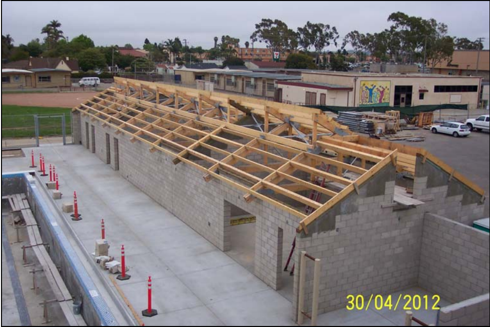
SMHS – Pool Equipment Room Roof Takes Shape
