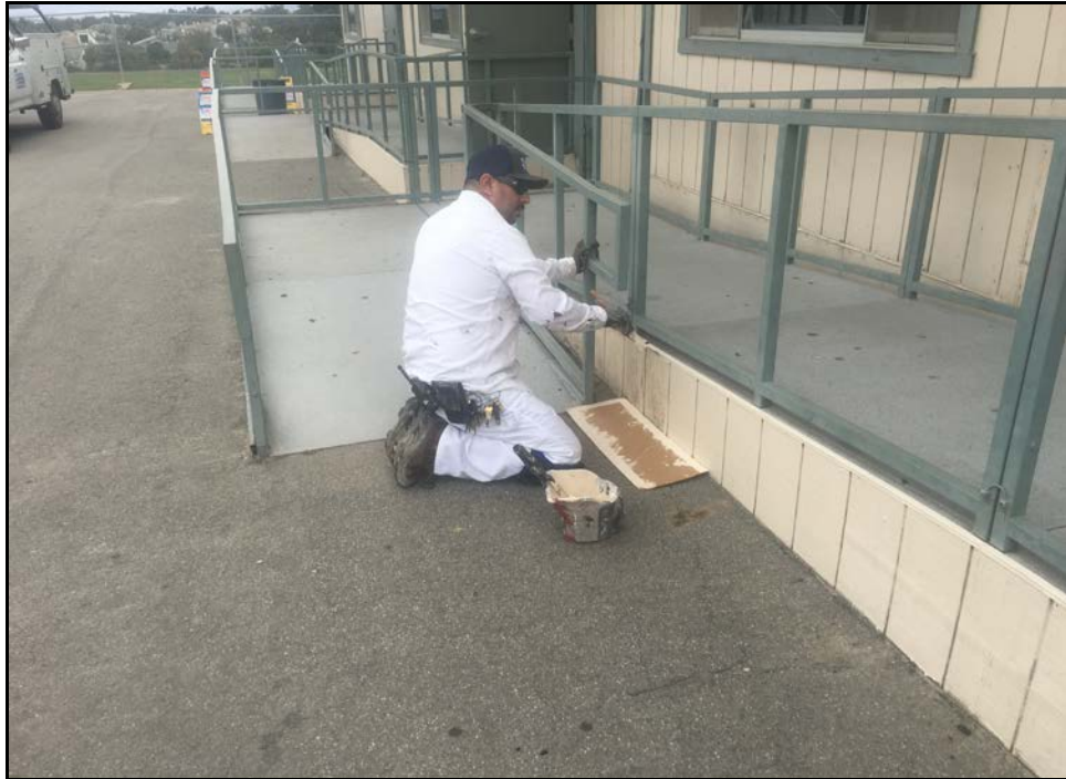
ERHS - Ernest Paz Freshens Up the Appearance of a Relocatable Classroom
