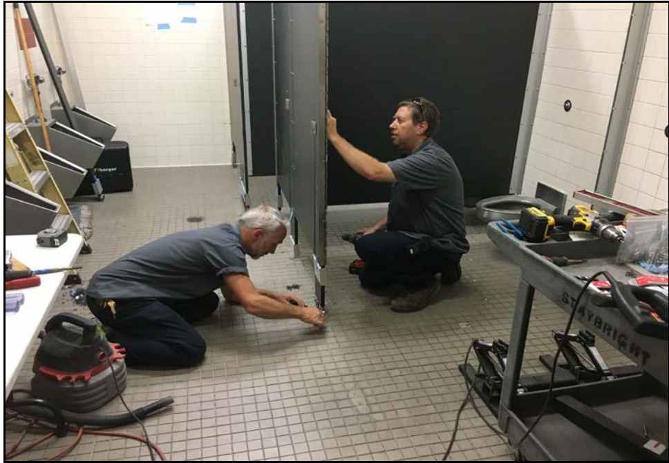
SMHS - Eric Fulton and Greg Parker Install New Partitions at the Wilson Gymnasium Boys' Locker Room Restroom....
