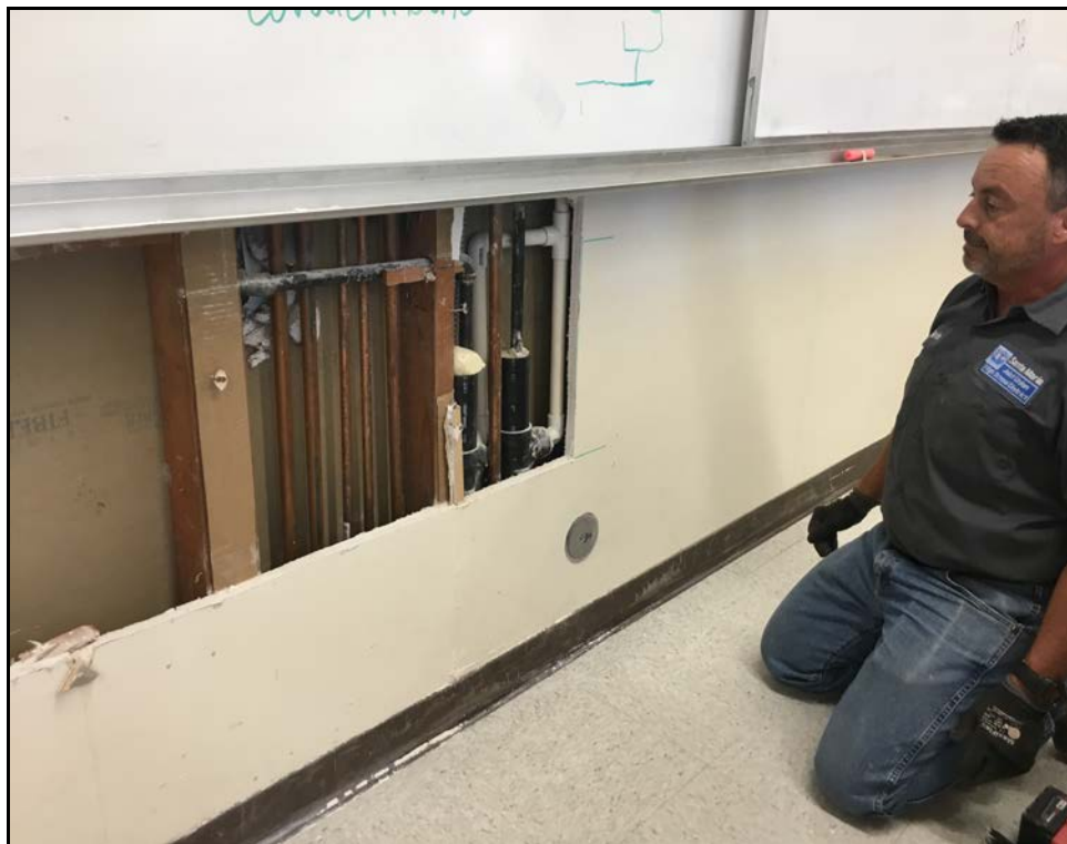
ERHS- Bernie Rayner Troubleshoots a Science Classroom Gas Line
