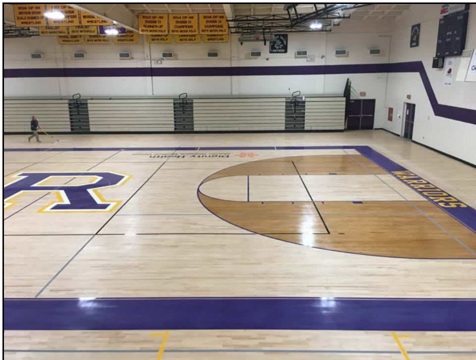
ERHS Gymnasium Floor - Sanded, Painted, and Floor Finish Applied; Ready for Action!
