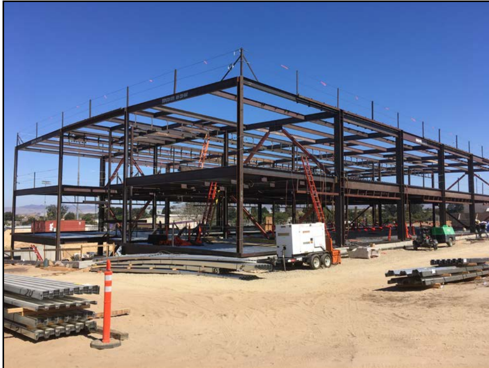
ERHS 38 Classroom Building – Second and Third Floor Steel is Set
