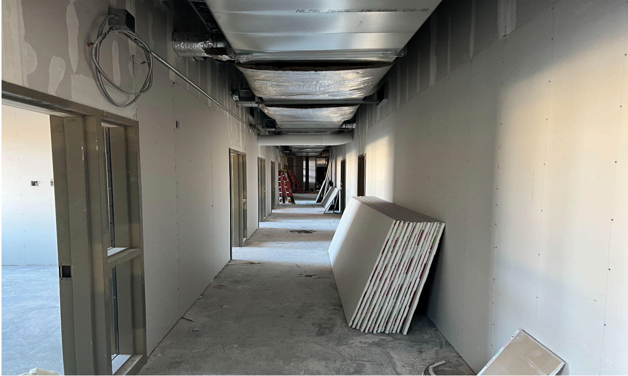
Office area corridor on the north side of the new addition.
