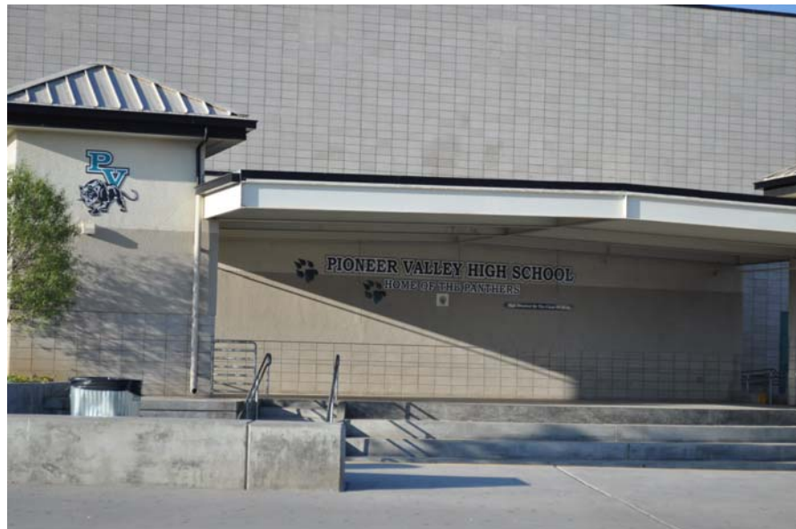
Pioneer Valley Gymnasium Remediation - Roof Repairs and Rain Gutters
