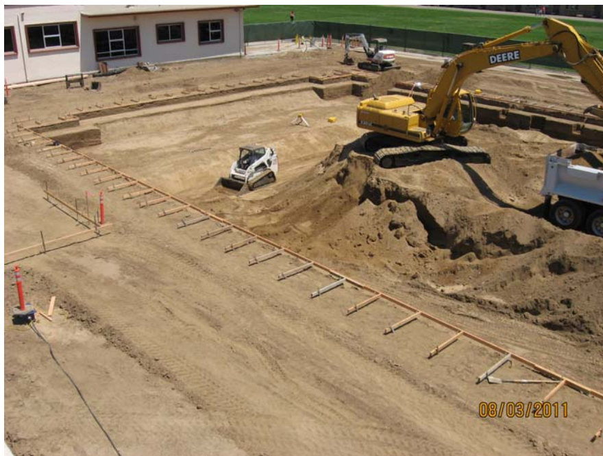
Santa Maria High Pool In-progress
