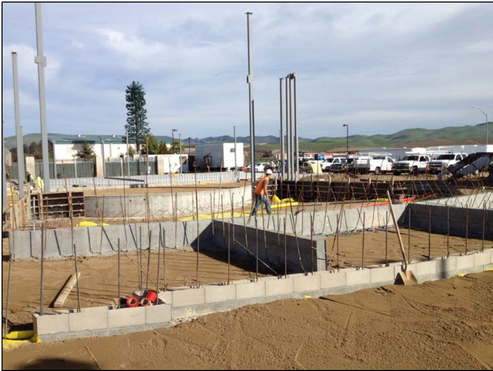
PVHS – Performing Arts Center Stage Begins to Take Shape
