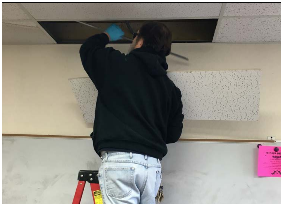
ERHS – David Burrill Replaces Damaged Ceiling Tiles in a Classroom
