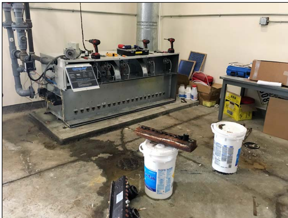
ERHS – Pool Heater Heat Exchanger Replacement In-progress
