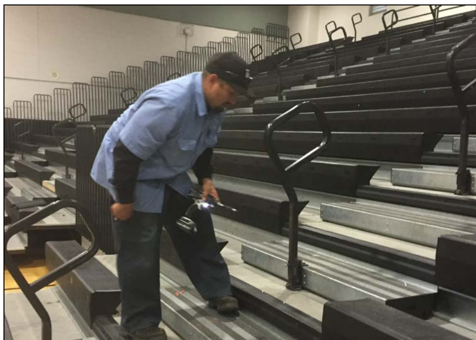
PVHS - Elias Comacho Replaces Gymnasium Bleacher Handrails
