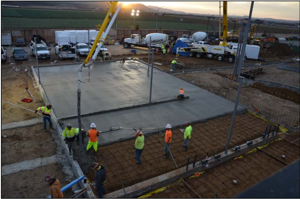
PVHS – Performing Arts Classroom Floors are Poured Early in the Morning
