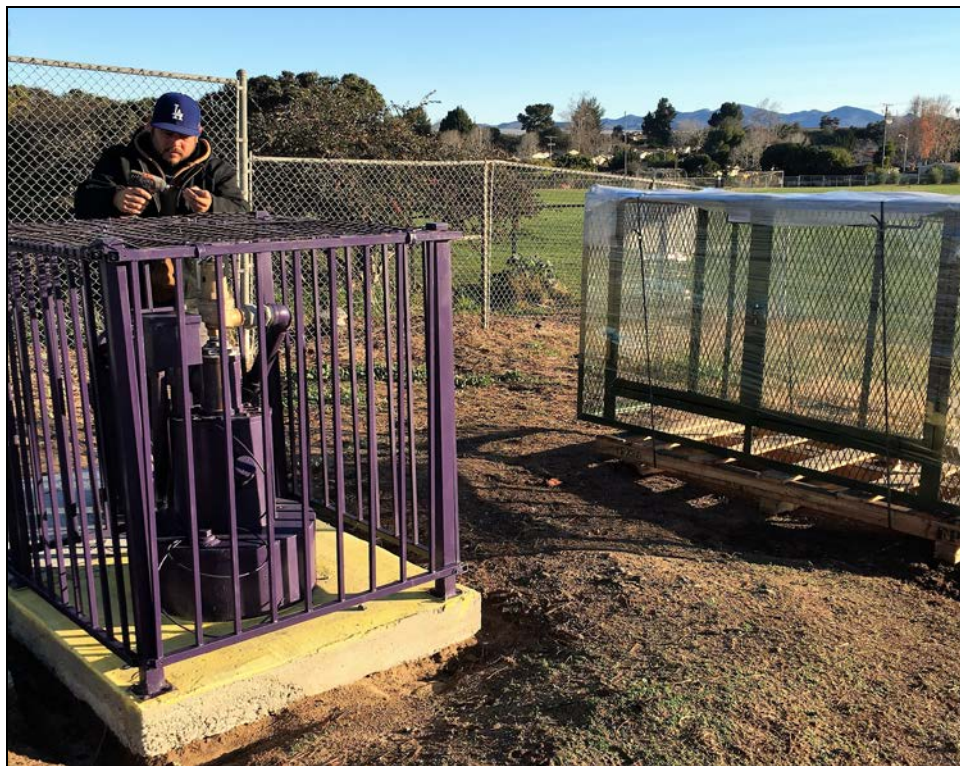
ERHS – Flavio Rodriguez Replaces the Access Cage for the Irrigation Well Head
