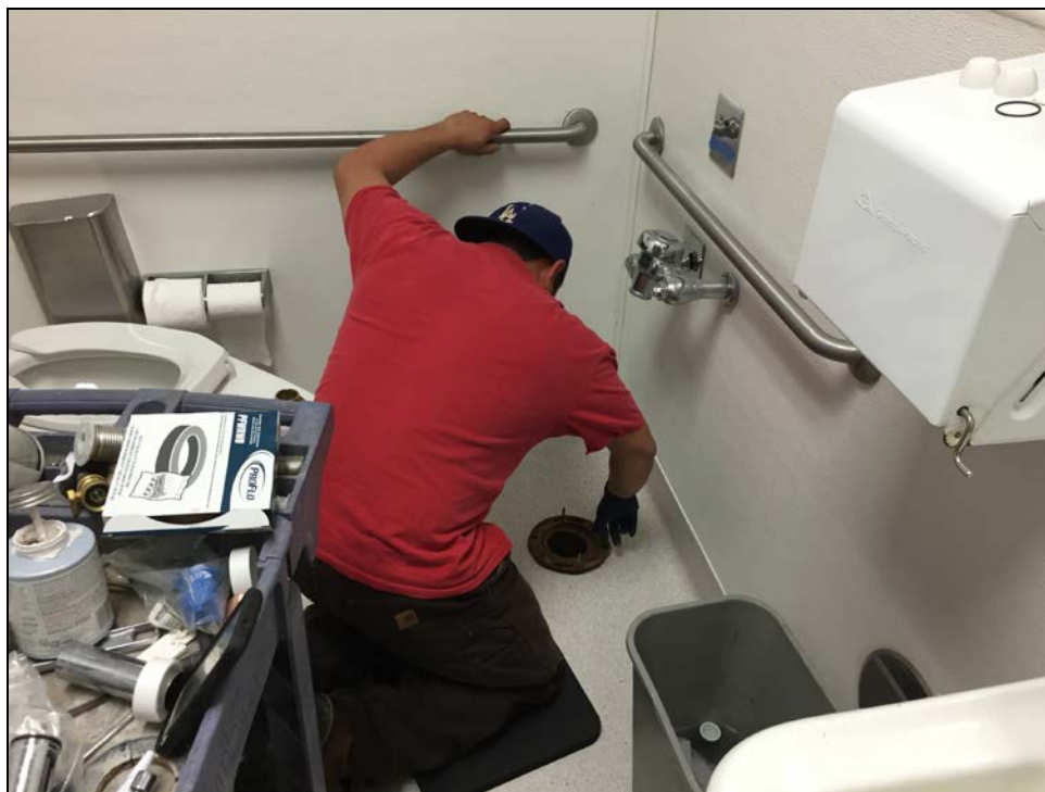
PVHS - Flavio Rodriguez Installs Low-Flow Fixtures after Replacing Staff Restroom Flooring
