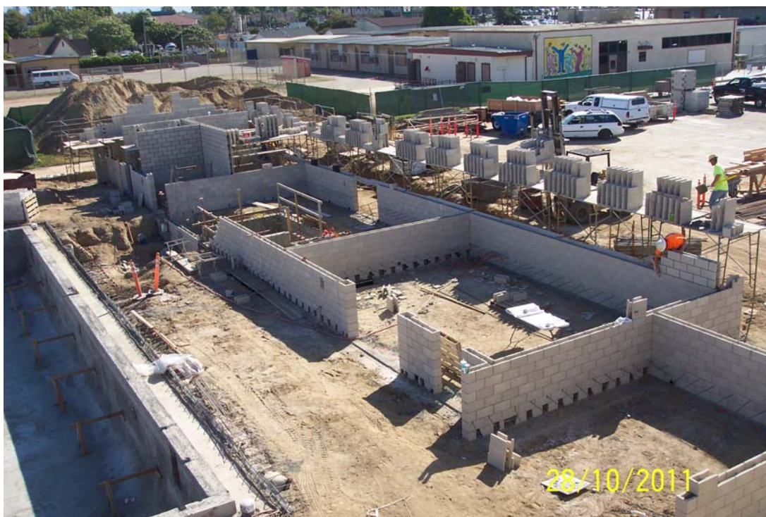
SMHS Pool Equipment Room Begins to Take Shape
