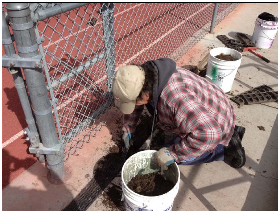
ERHS - Juan Rodriguez Cleaning Storm Drains at the Football Stadium
