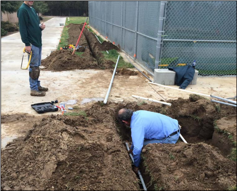
PVHS – Dell Ward and José Placencia Lay Conduit for Power at the Baseball Field
