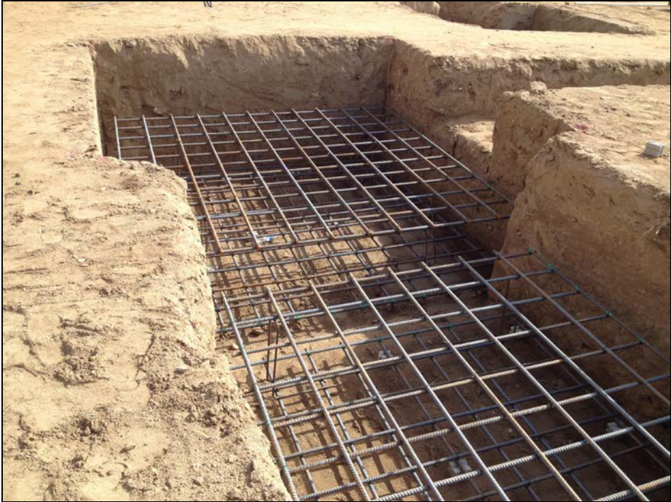
SMHS –Concrete Reinforcing Bars Installed for Footings
