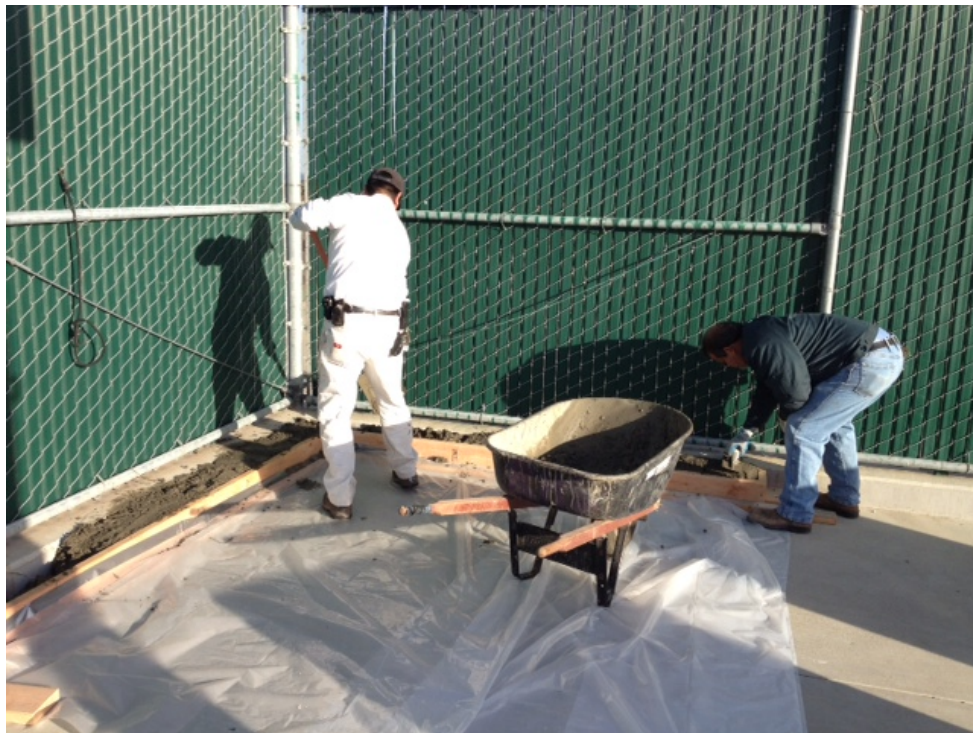
ERHS – Ernest Paz and José Placencia Pour Footings for new Lockers at the Pool
