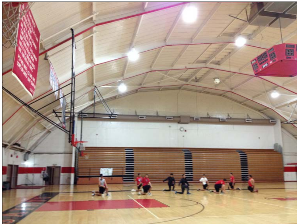
SMHS - Energy Conversion ... New Inductive Lights in Wilson Gymnasium
