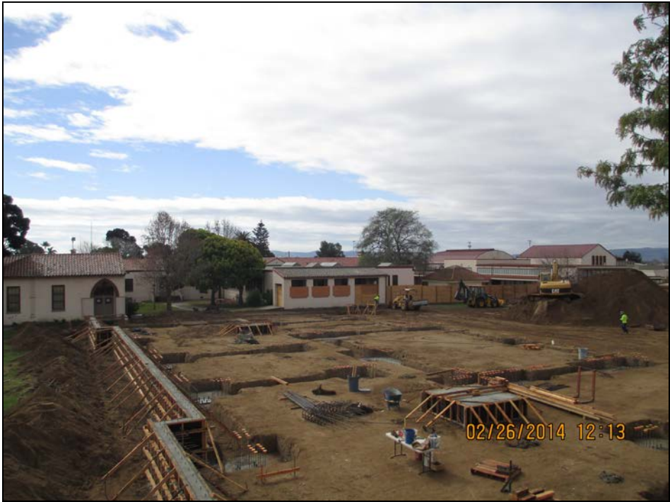
SMHS – 14-Classroom Building Footings in Place
