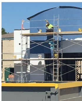
Workers paint the façade of the new Guardian Catholic School entrance
