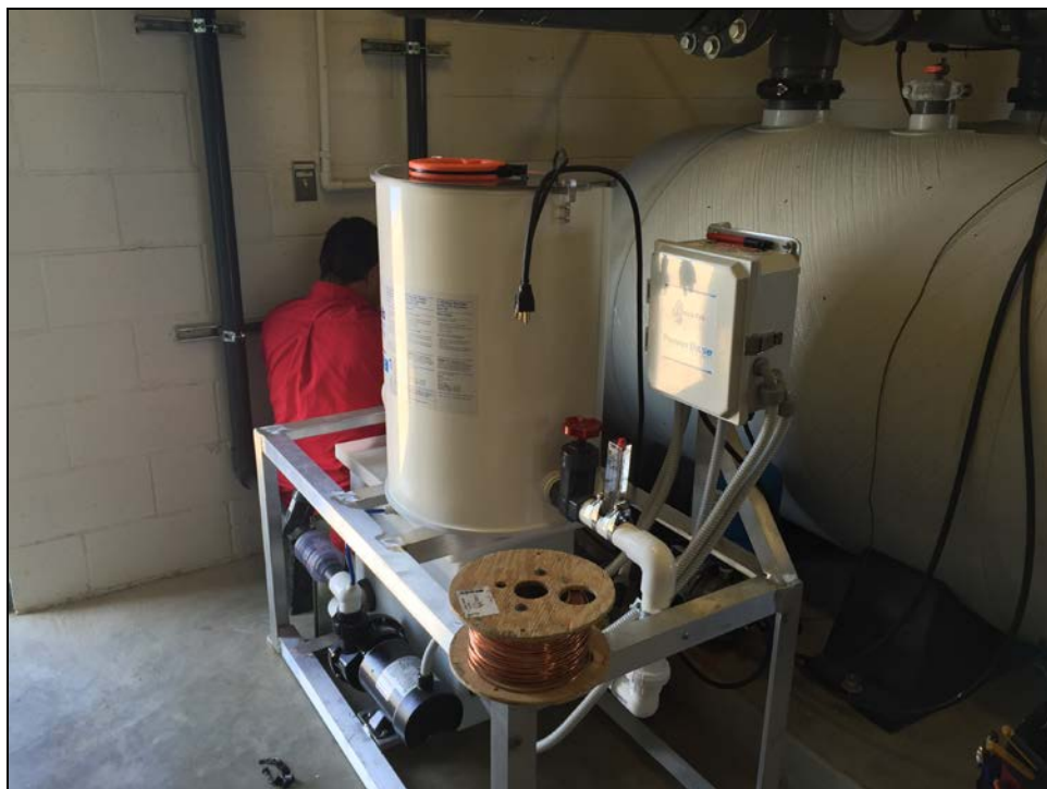
PVHS - Pool Chemical Dispensing Changed from Liquid Chlorine to Tablets
