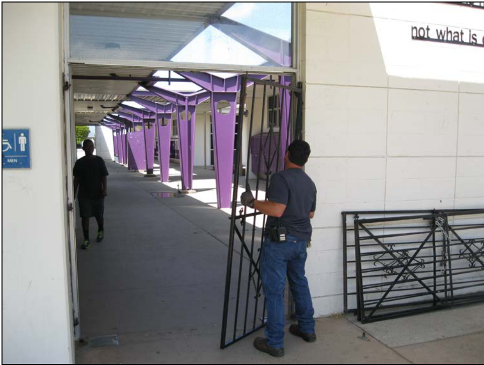
ERHS - Bernie Rayner Removes Gates to Open the Traffic Flow Between Classrooms
