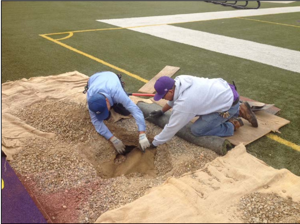
ERHS – Juan and Nelson Repair Gopher Damage at the Football Field
