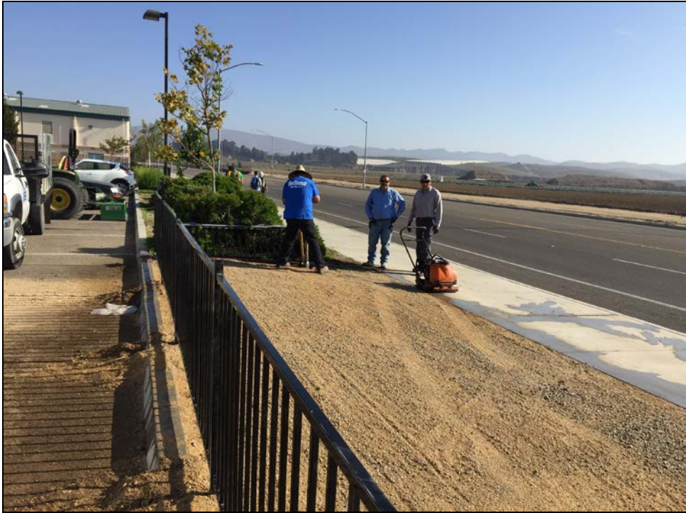
PVHS – New Bus Loading Que Under Construction
