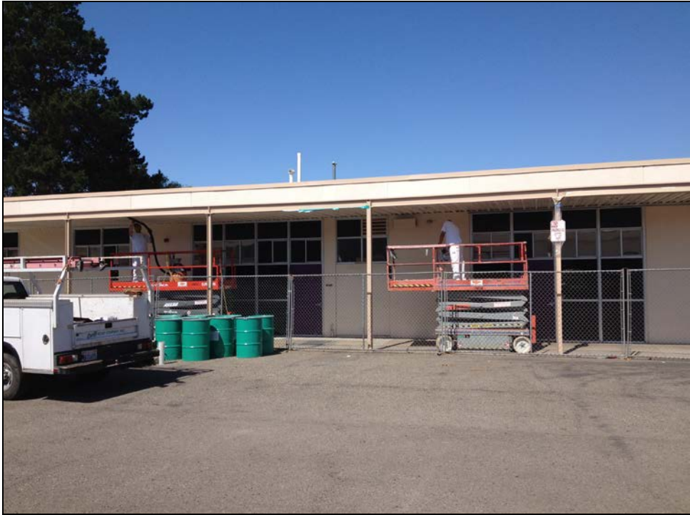
ERHS – Covered Walkways are Repainted
