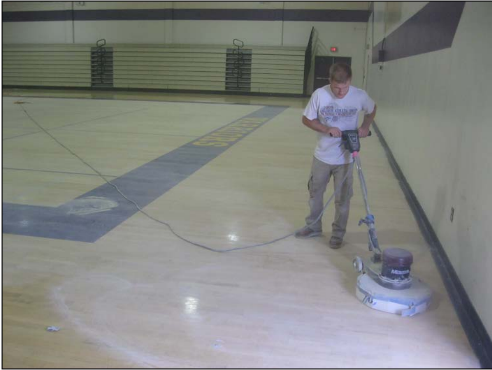
ERHS - Gymnasium Floor Undergoes Refinishing
