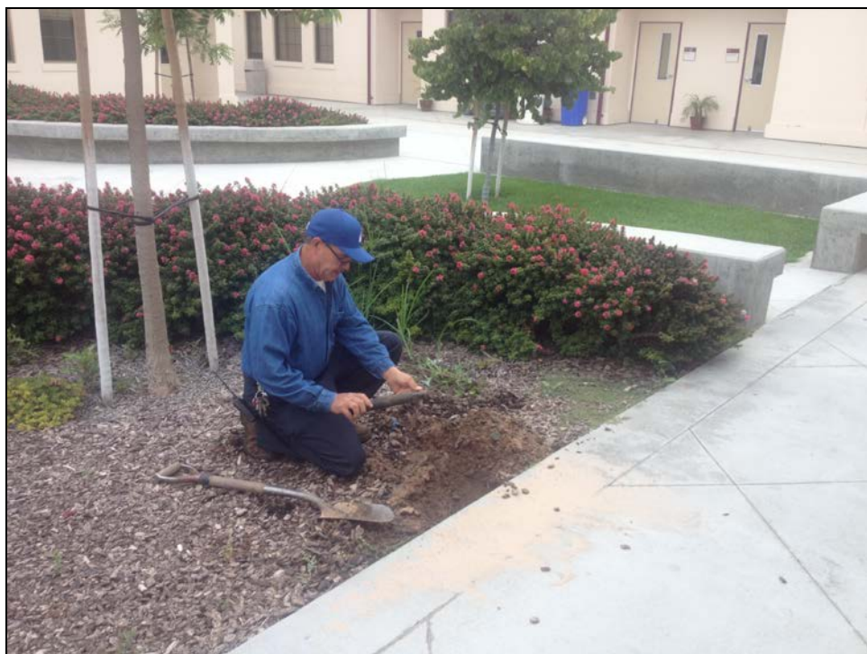
ERHS - Juan Rodriguez Replaces Sprinkler Heads
