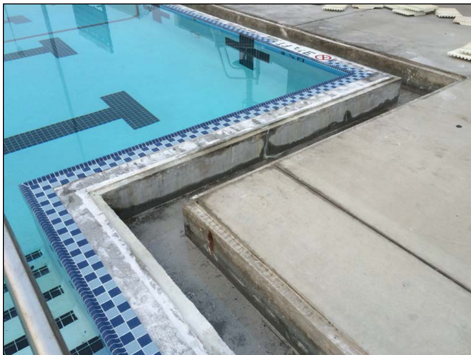
SMHS - Pool Tile Repair in Progress
