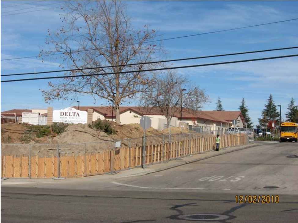
Retaining Wall for Delta High School (in progress)
