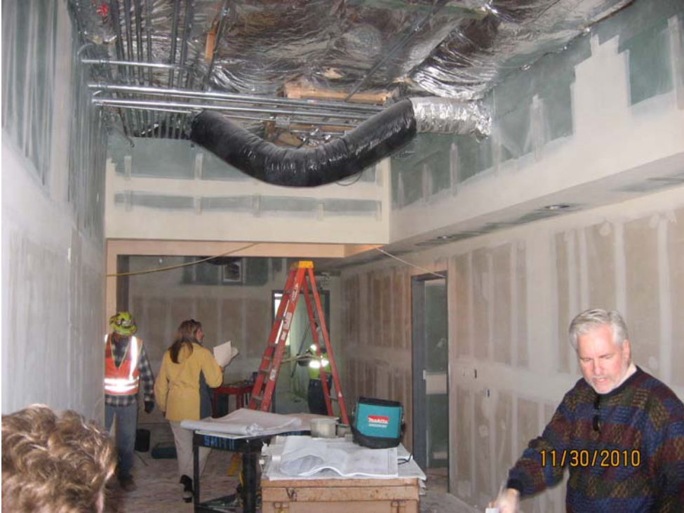
Righetti High Administration Renovations Take Shape
