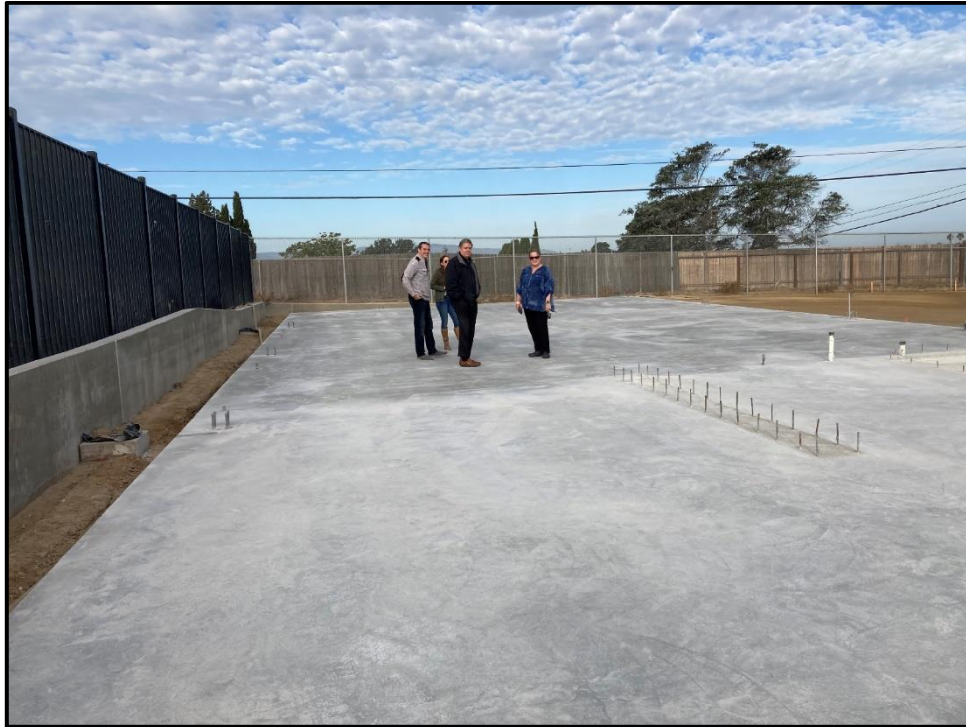
ERHS Maintenance and Operations Building – Design Team and Contractor Inspect the Maintenance Shop Floor Slab Finish
