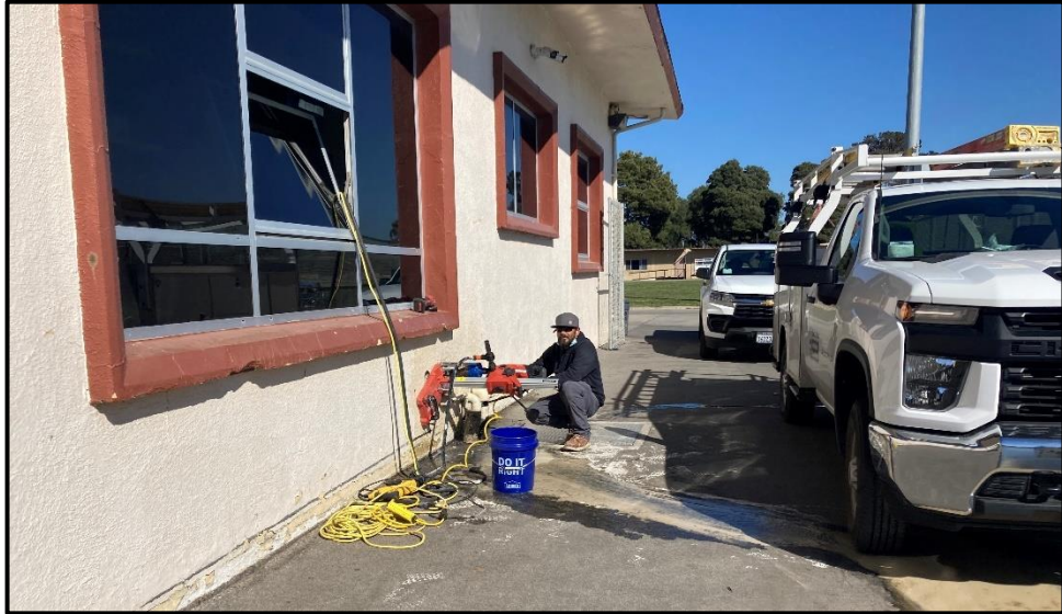
SMHS – Thomas Harbold Drilling Vent Holes for the Washer and Dryer in Wilson Gym
