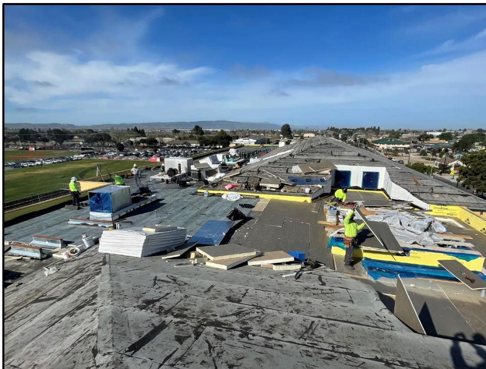
SMHS 50-Classroom Building – Roofing is Underway on Built-up Flat Sections as Well as Tile Peaked Areas
