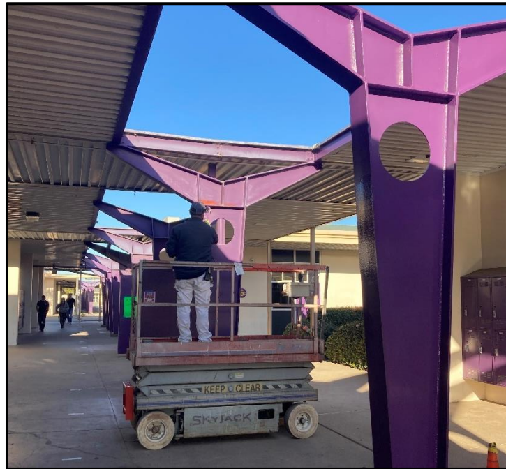
ERHS – Ernest Paz Repainting the Y Beams in the Hallway
