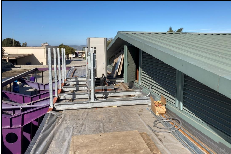
ERHS Modernization – Air Conditioning Compressors are Placed on the Covered Walkway Roofs
