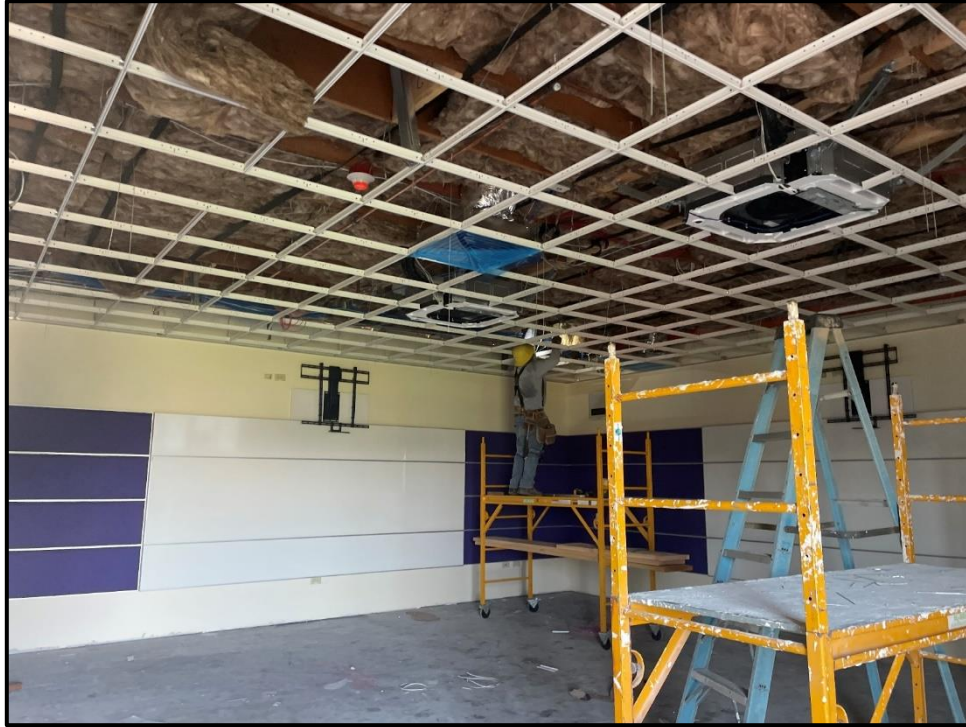
ERHS Modernization – Ceiling Grid is Installed
