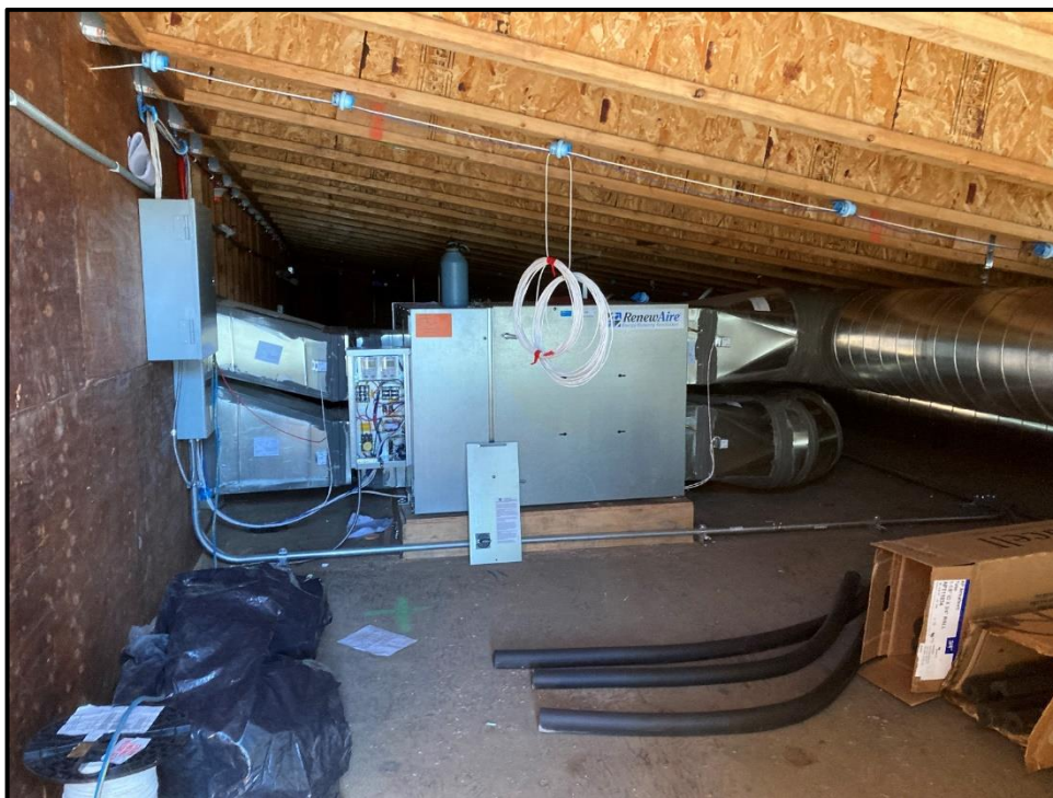
ERHS Modernization – Air Conditioning Evaporators are Located in the Attic with all New Air Ducts
