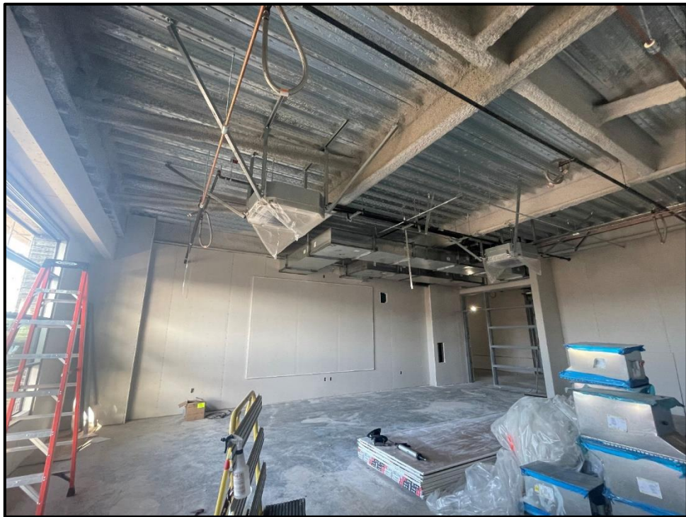
SMHS 50-Classroom Building – Classroom Interior Finishes and Air Conditioning Installation In-progress
