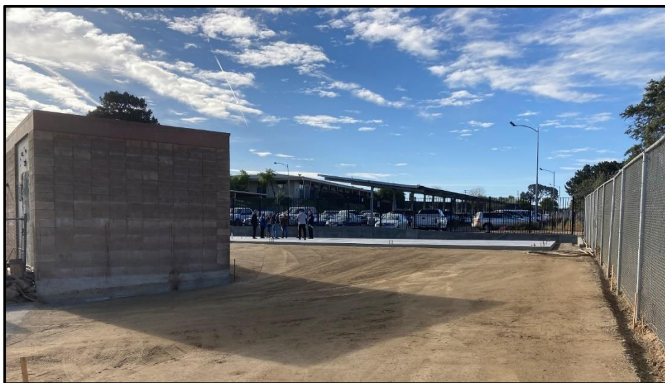
ERHS Maintenance and Operations Building – Grading of the Maintenance Yard is Complete
