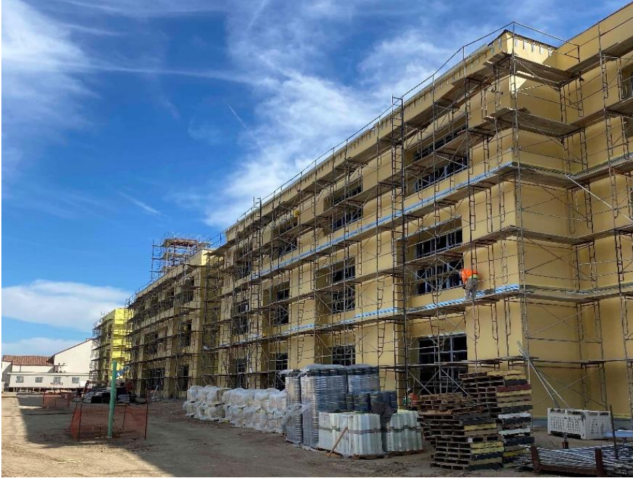
Santa Maria High School 50-Classroom & Administration Building March 2022
