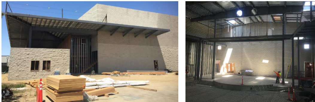
Pioneer Valley High School Performing Arts Center Construction Progress (July 2016)
