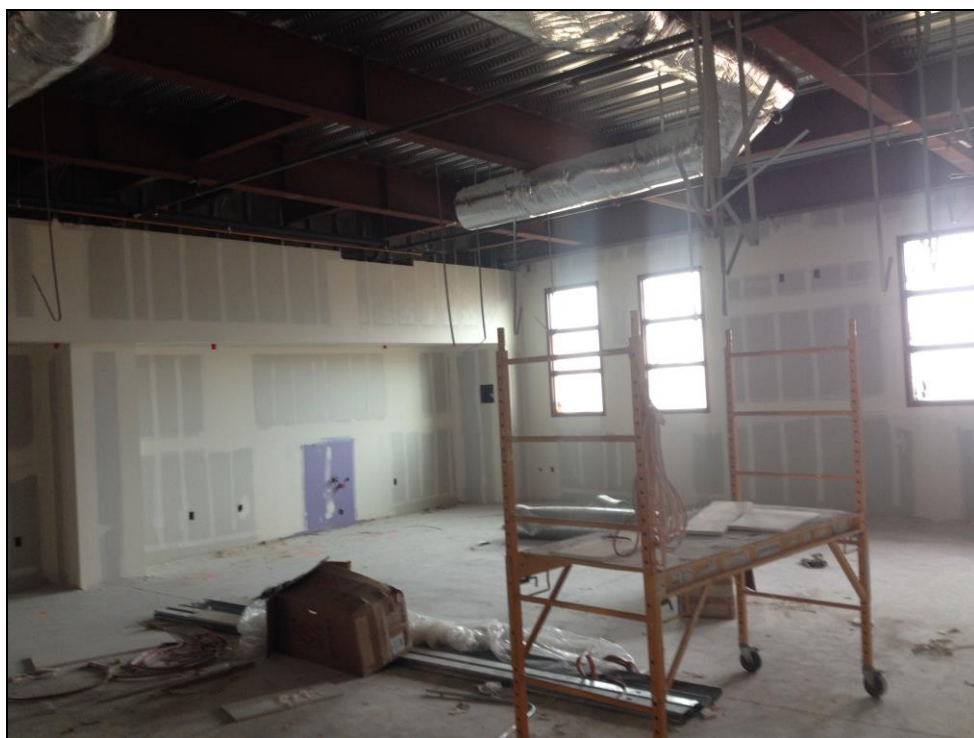
SMHS – 14-Classroom Building Interior Finish Work Underway
