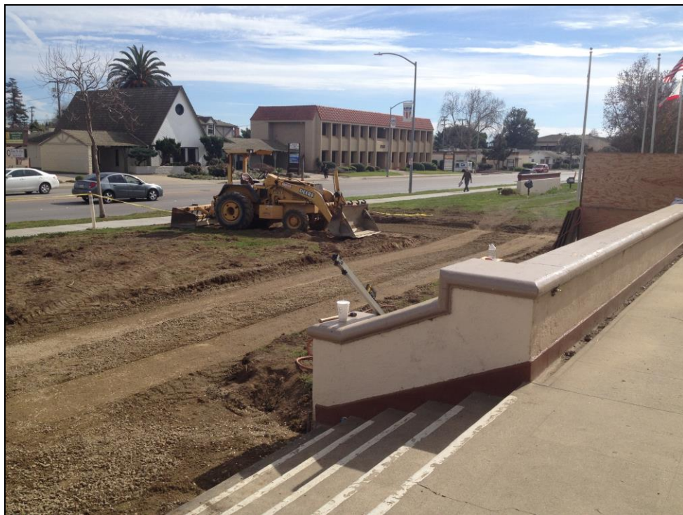
SMHS – New Walkways Improve Access to Ethel Pope Auditorium and the New Classrooms
