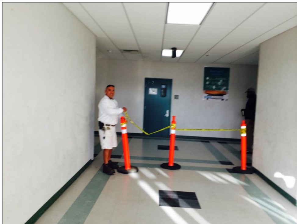
PVHS – Ray Segovia Repairs Damaged Walls in the Science Building Hallway
