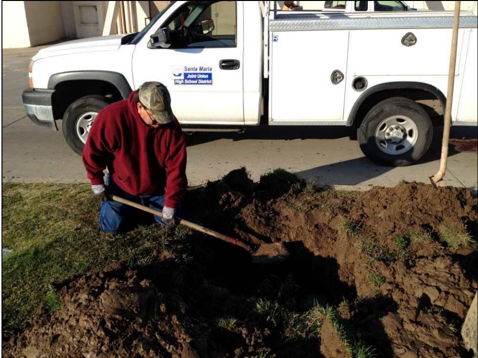
SMHS – Richard McKinley Repairs an Irrigation Water Leak in the Practice Field
