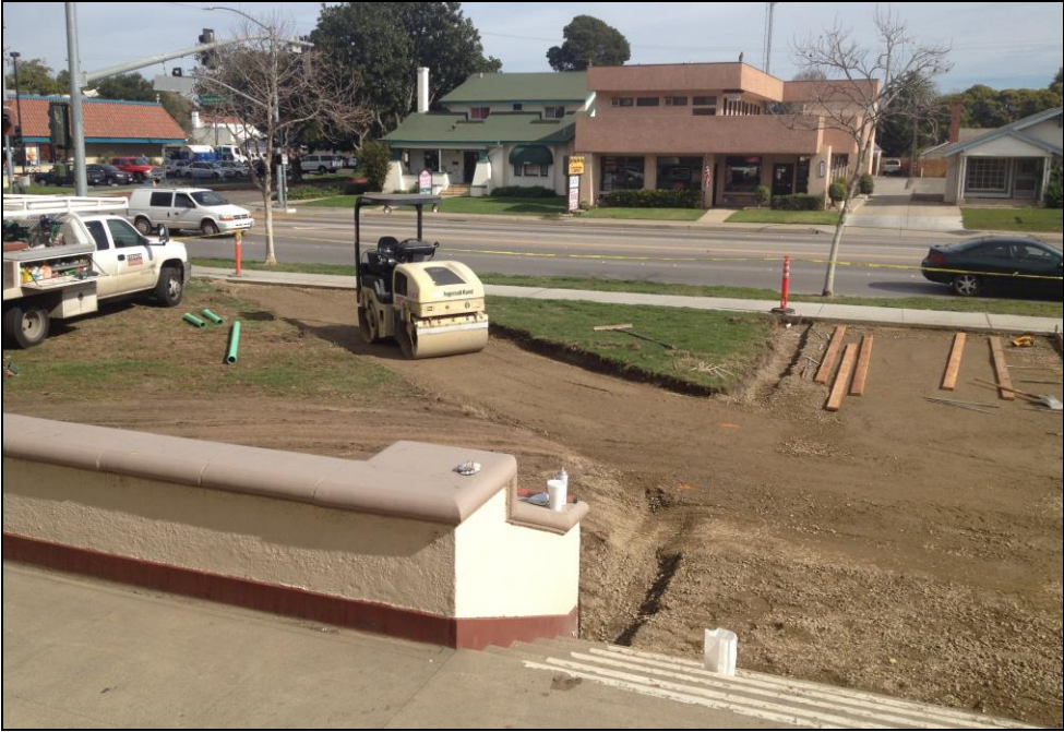
SMHS – New Walkways Accompany the 14 Classroom Addition
