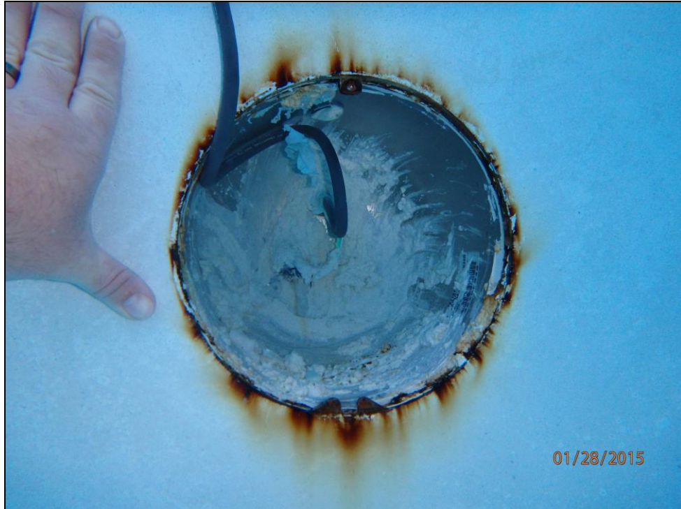
SMHS – City Pool Crew Repairs a Pool Light
