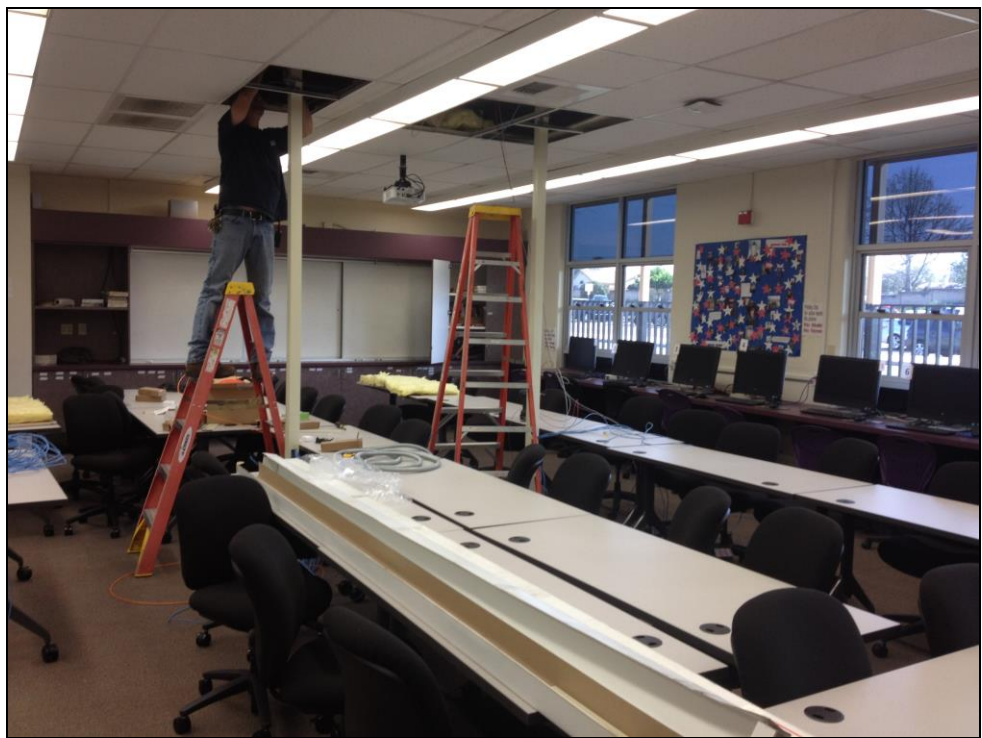
ERHS – Del Ward Wires the Library Lecture Area for Computerized Testing Lab
