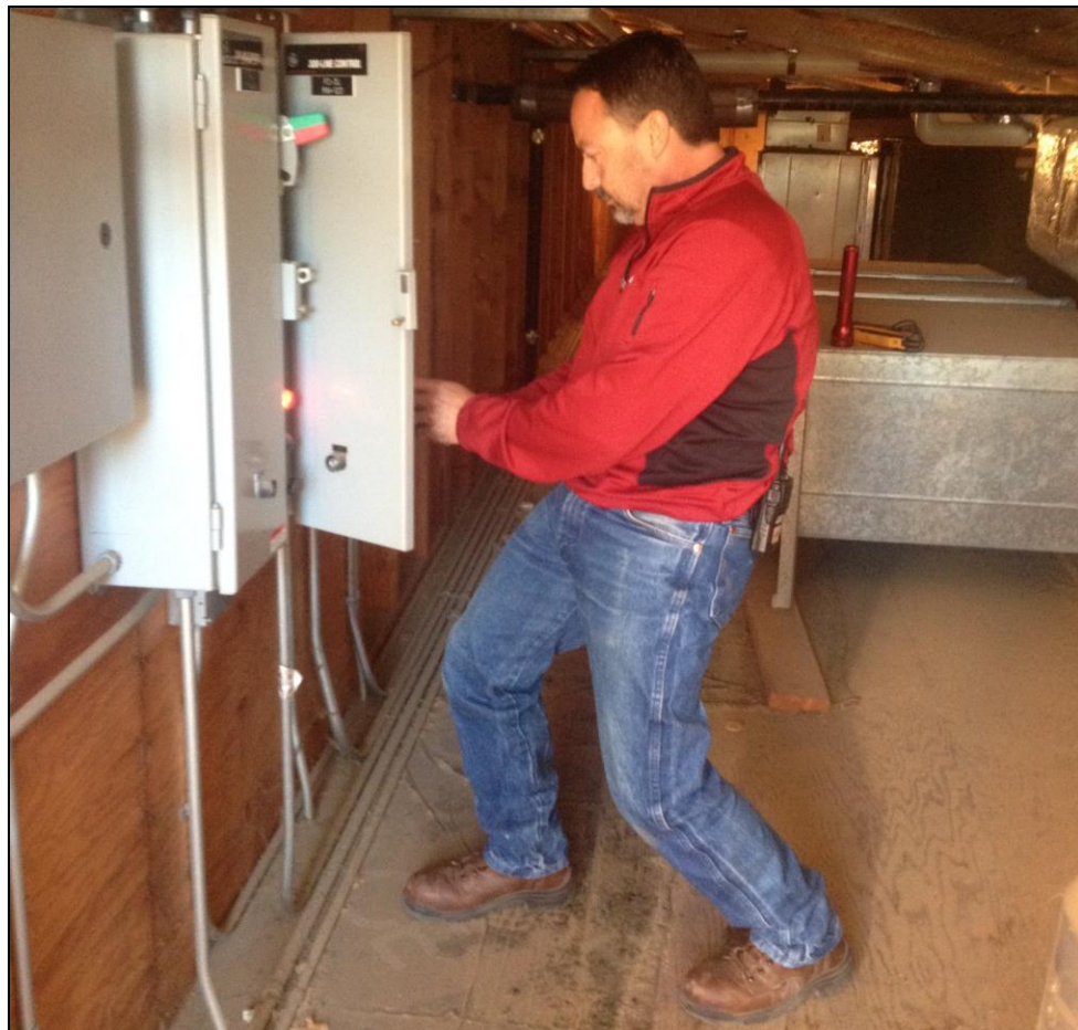
EHRH - Bernie Rayner in the Science Building Attic Services Heating Units
