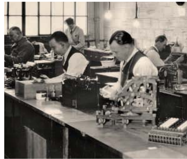
▲ The Civil Works Administration enabled these men to get jobs repairing typewriters and sewing machines.
