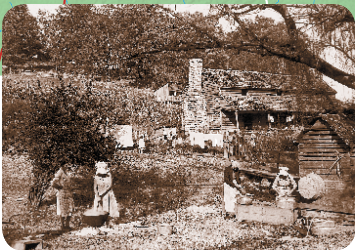
▲ Before 1930, most homes in the area had no electricity. Women wash clothes outside this homestead near Andersonville, Tennessee, in 1933. Their estate was submerged when the Norris Dam filled.
