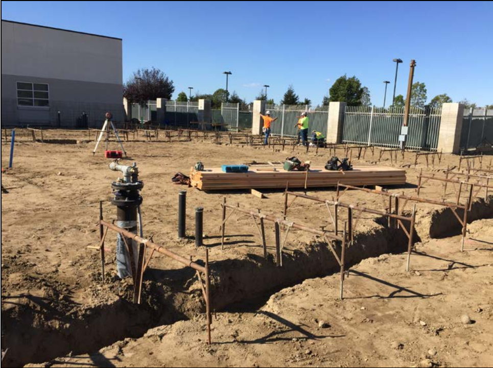
PVHS – Performing Arts Center Utilities Installed and Footings Await Rebar
