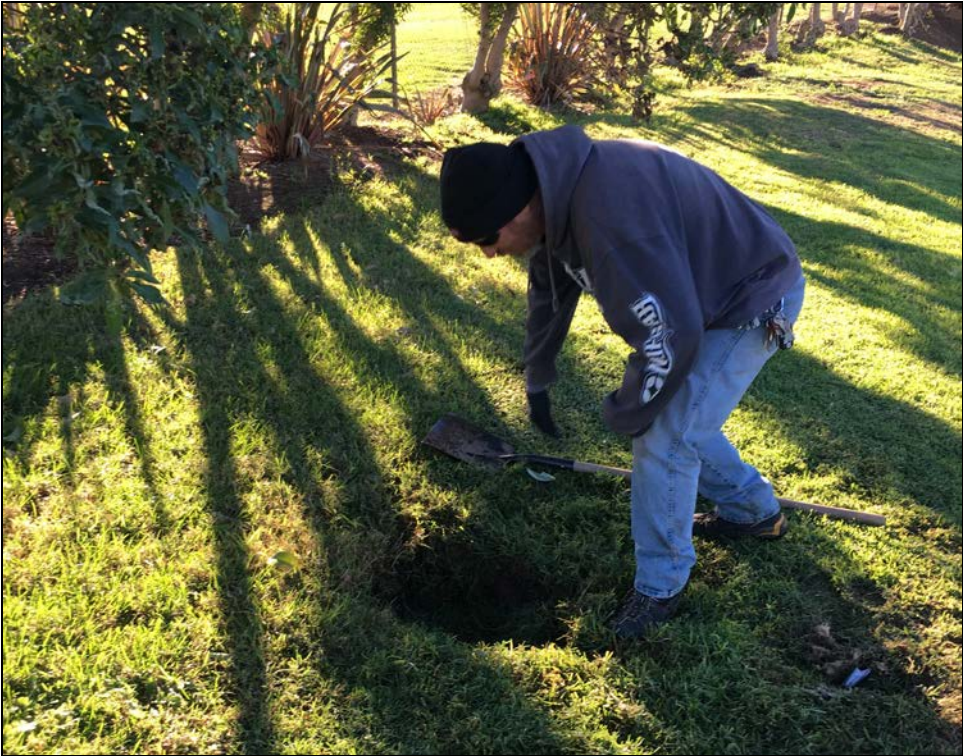
ERHS - Denton Tilley Repairs a Broken Sprinkler line Near Varsity Baseball
