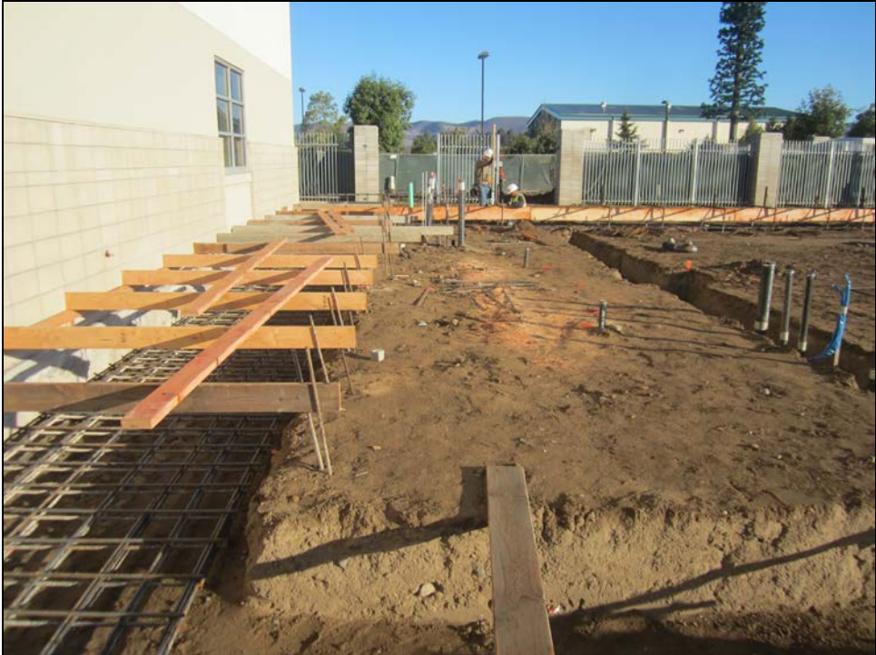
PVHS – Huge Footings Receive Rebar and Begin Forming for Concrete
