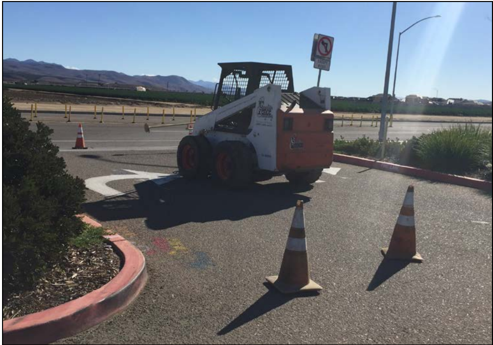
PVHS – New Gate Installation Begins at the Front of the School
