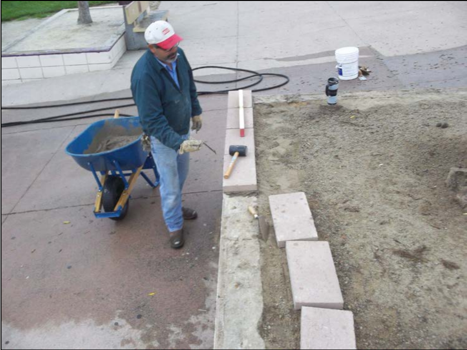
ERHS - José Placencia Replaces the Block Wall Caps in the Quad
