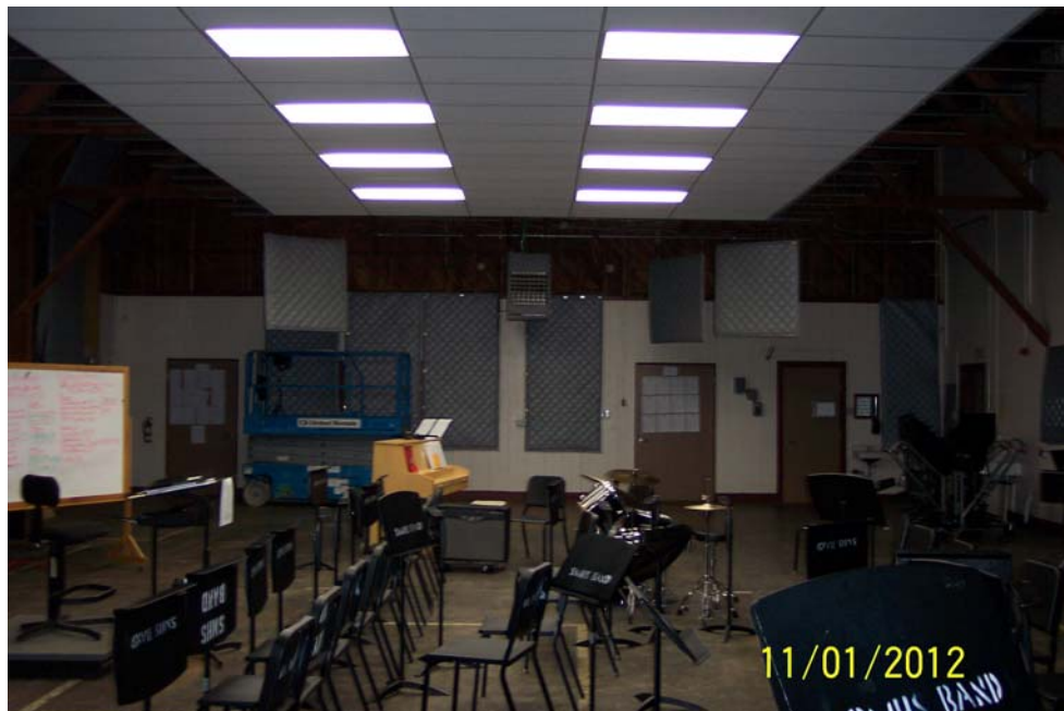
SMHS Band Room - Completed Acoustic Ceiling & Lighting Upgrades
