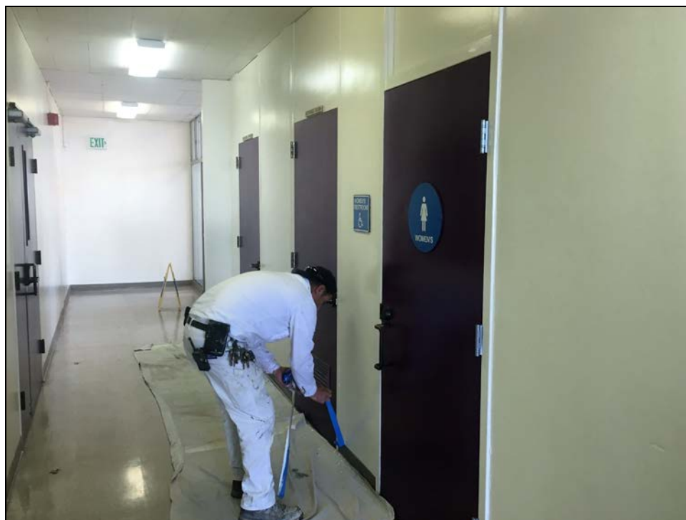
ERHS - Ernest Paz Completes Painting at the Cafeteria Restrooms
