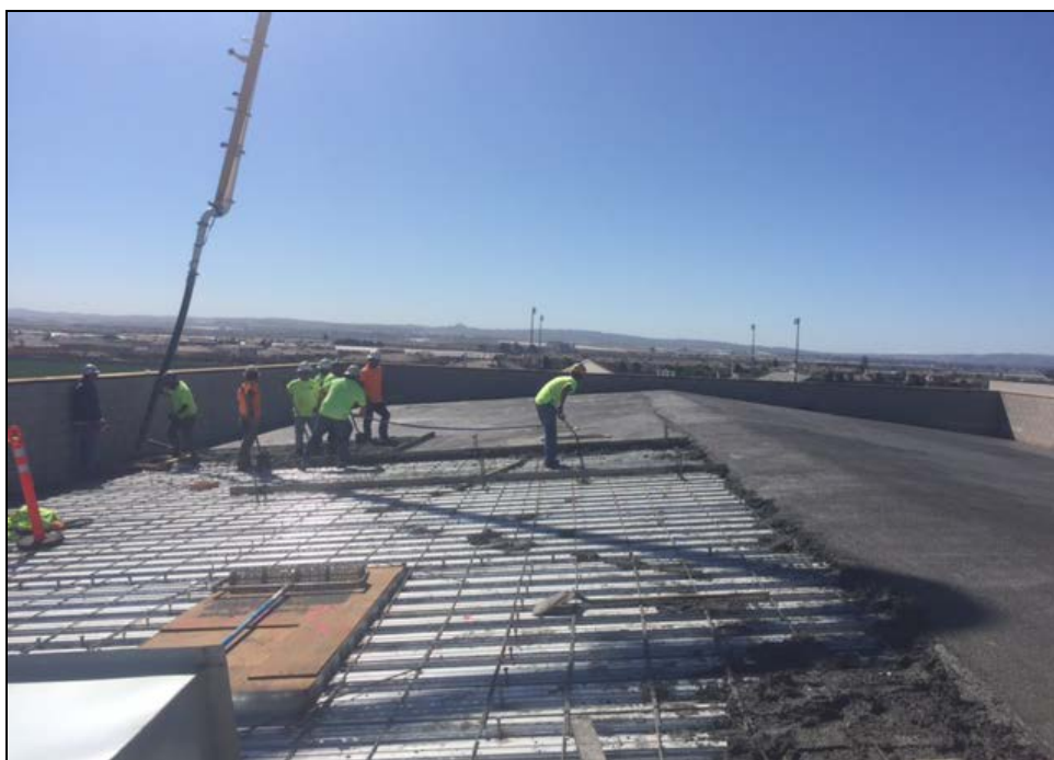
PVHS – Performing Arts Center Roof – Concrete Applied over the Metal Decking
