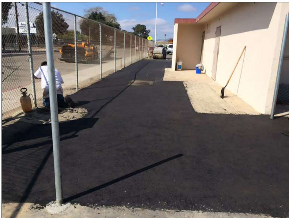
SMHS - Asphalt Improvements at the Football Stadium Restrooms
