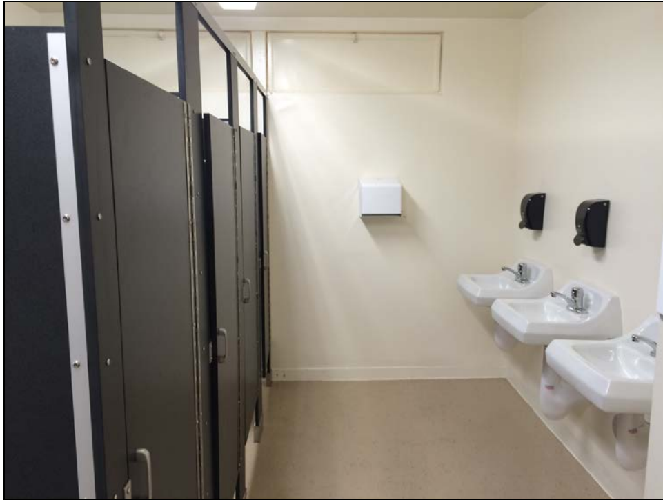
SMHS - New Restroom Partitions and sinks at the Football Stadium
