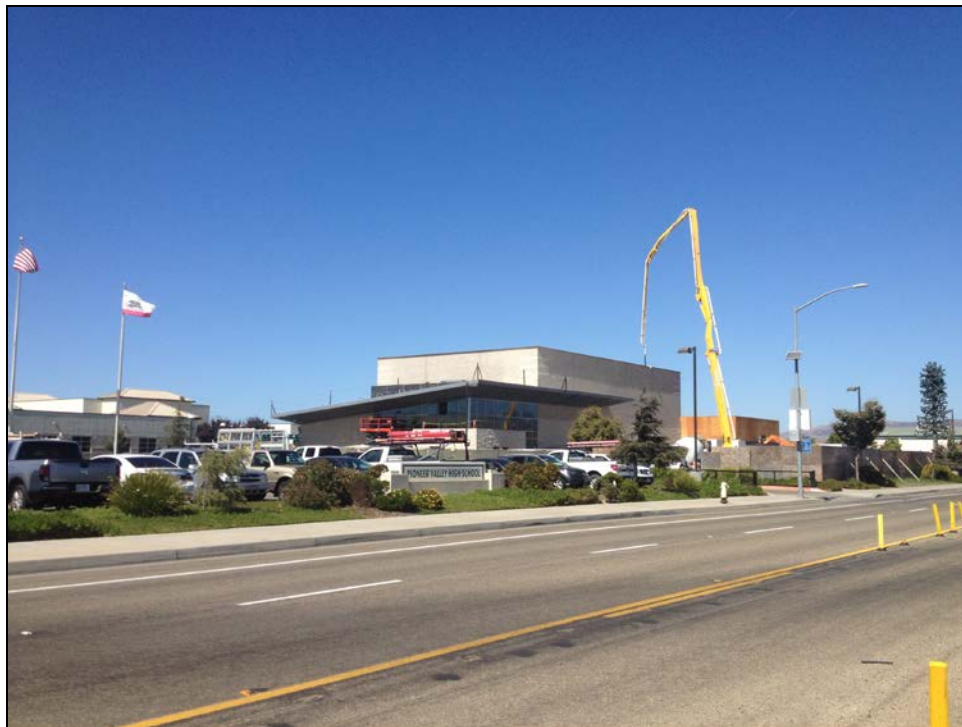
PVHS – Concrete Pump Lifts Lightweight Concrete to the Performing Arts Center Roof
