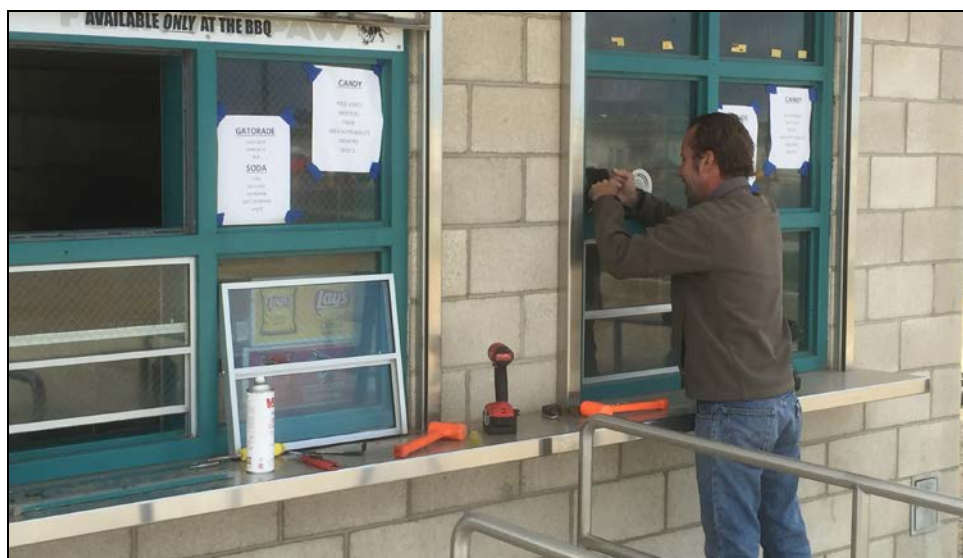
PVHS – Improved Serving Windows Installed at the Football Concession Stand
