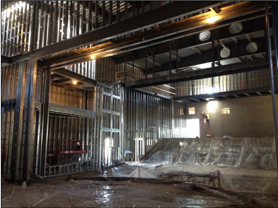
PVHS – Protecting the Theater Below While Pouring the Roof Deck
