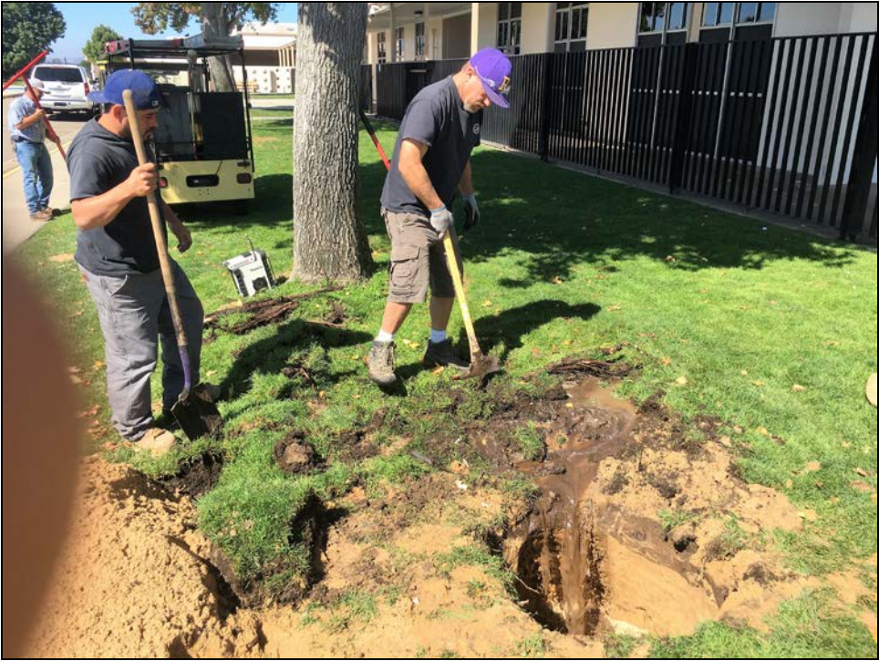
ERHS – Flavio Rodriguez and Denton Tilley Excavate a Water Leak in Front of the School
