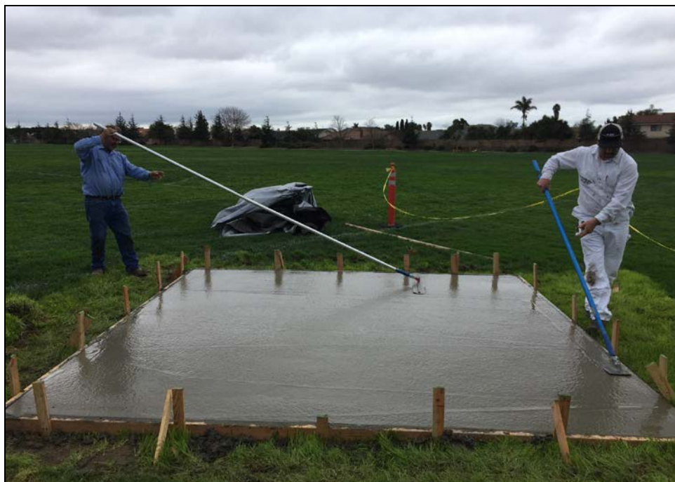
PVHS – José Placencia and Ernest Paz finish replacement concrete pad for Discus
