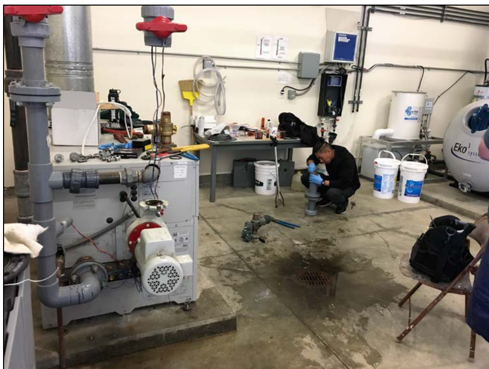
ERHS – Pool Heater Mixing Valve Repairs in Progress
