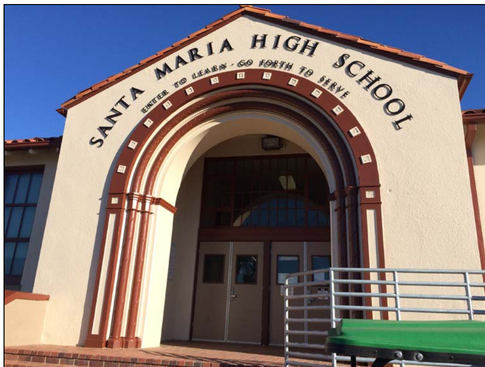
SMHS – Camino Colegio Street Entrance Receives New Paint
