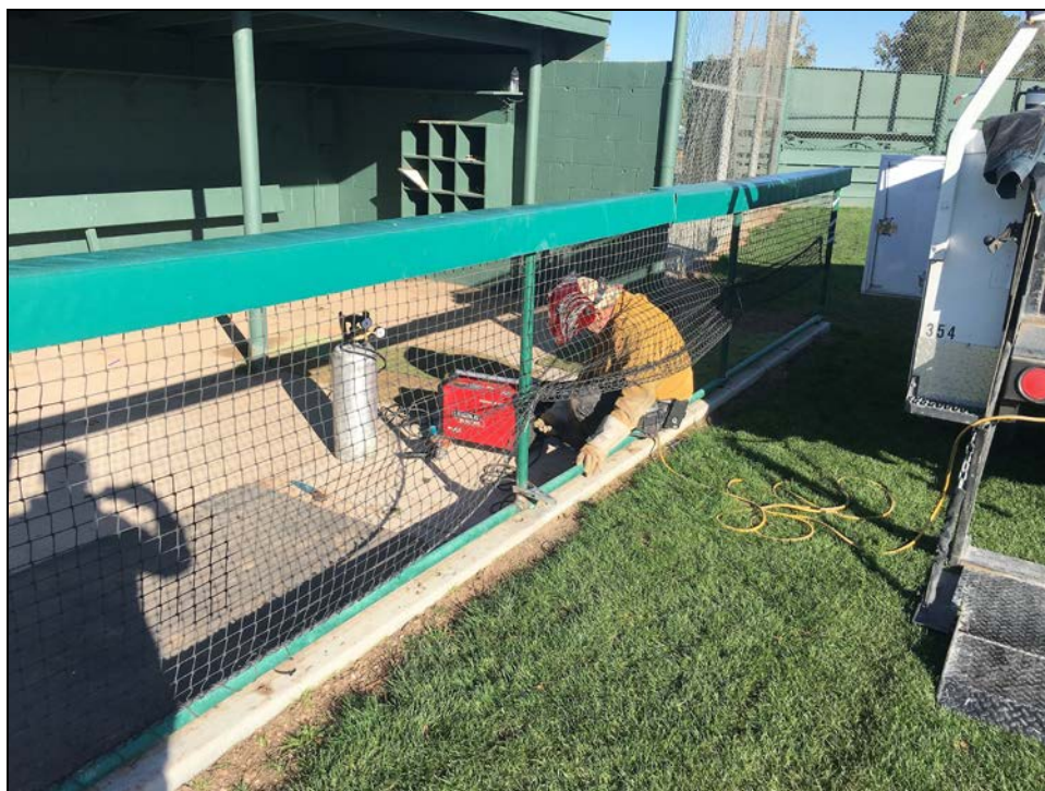
ERHS – José Placencia installs Safety Rail at the Varsity Baseball Dugouts
