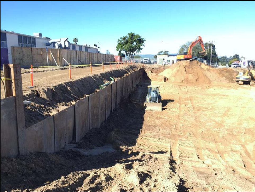
ERHS 38 Classroom Building – Excavation Underway!
