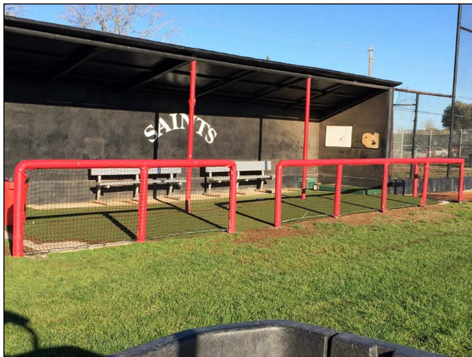
SMHS – New Safety Railing at the Baseball Dugouts
