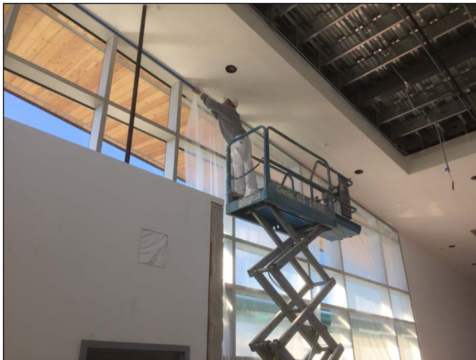
PVHS Performing Arts Center – Interior Painting in the Lobby
