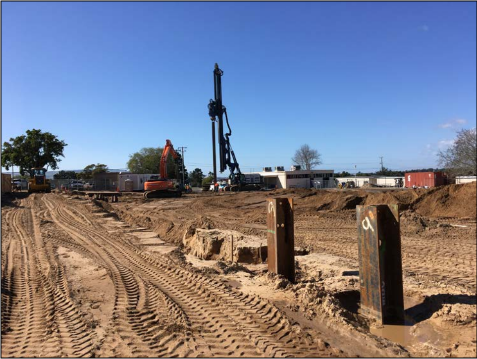
ERHS 38 Classroom Building – Pile Driver Prepares the Site for Excavation
