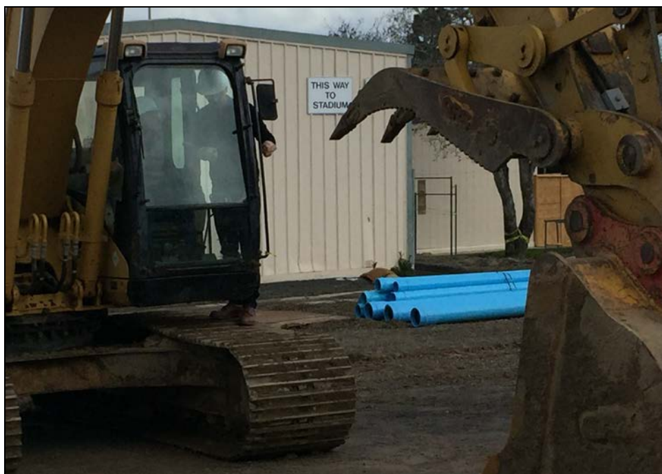
... and 21 st Century Ground Breaking – Dr. Karamitsos Operates Hydraulic Excavator
