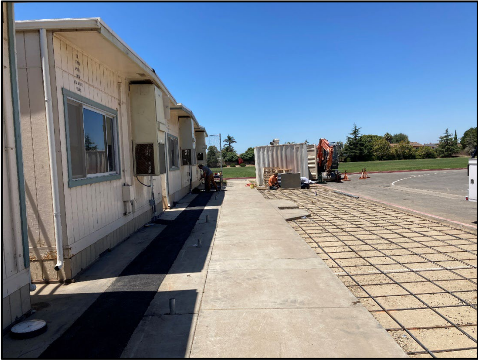
PVHS 10 Portable Classrooms – Concrete Replaces a Grass Parkway
