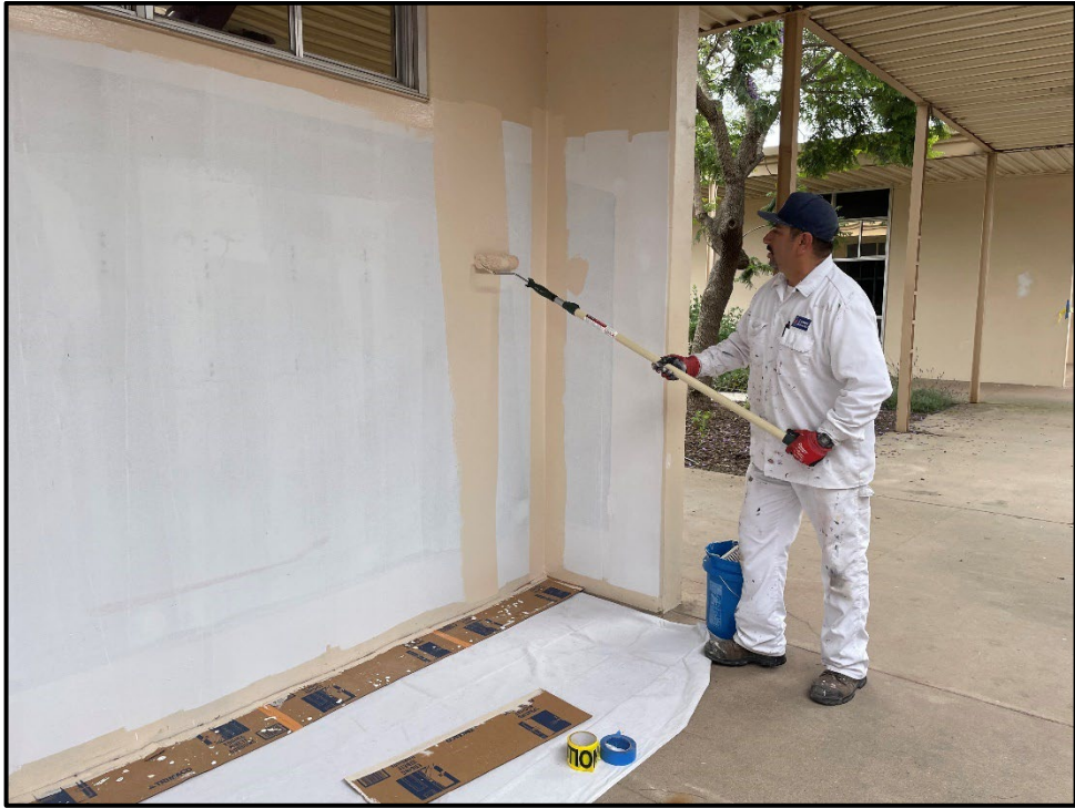
ERHS – Ernest Paz Painting Exterior Walls following Locker Removal
