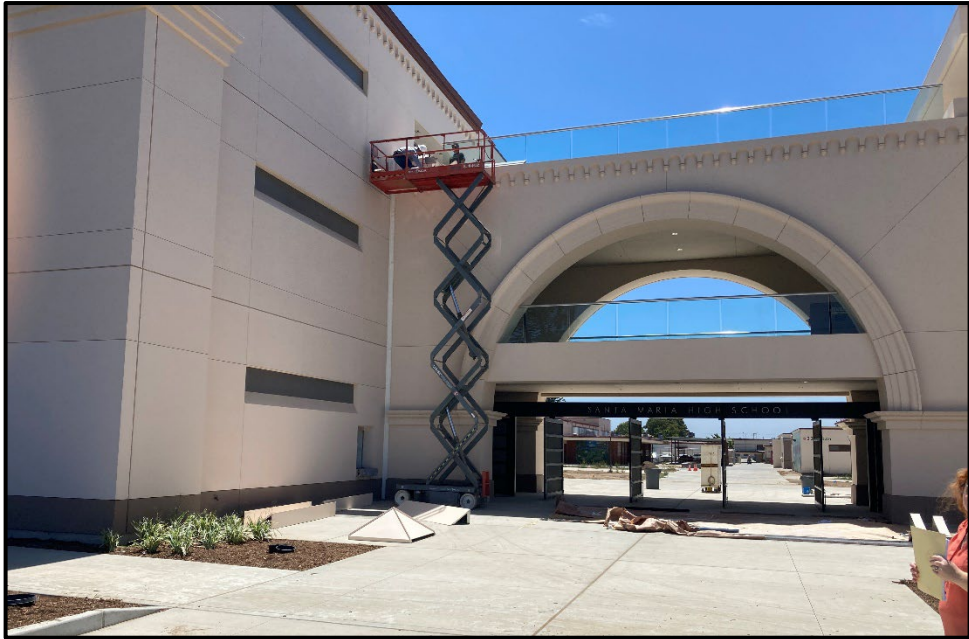
SMHS 50-Classroom Building – Installing the Third Floor Bridge Safety Enhancements
