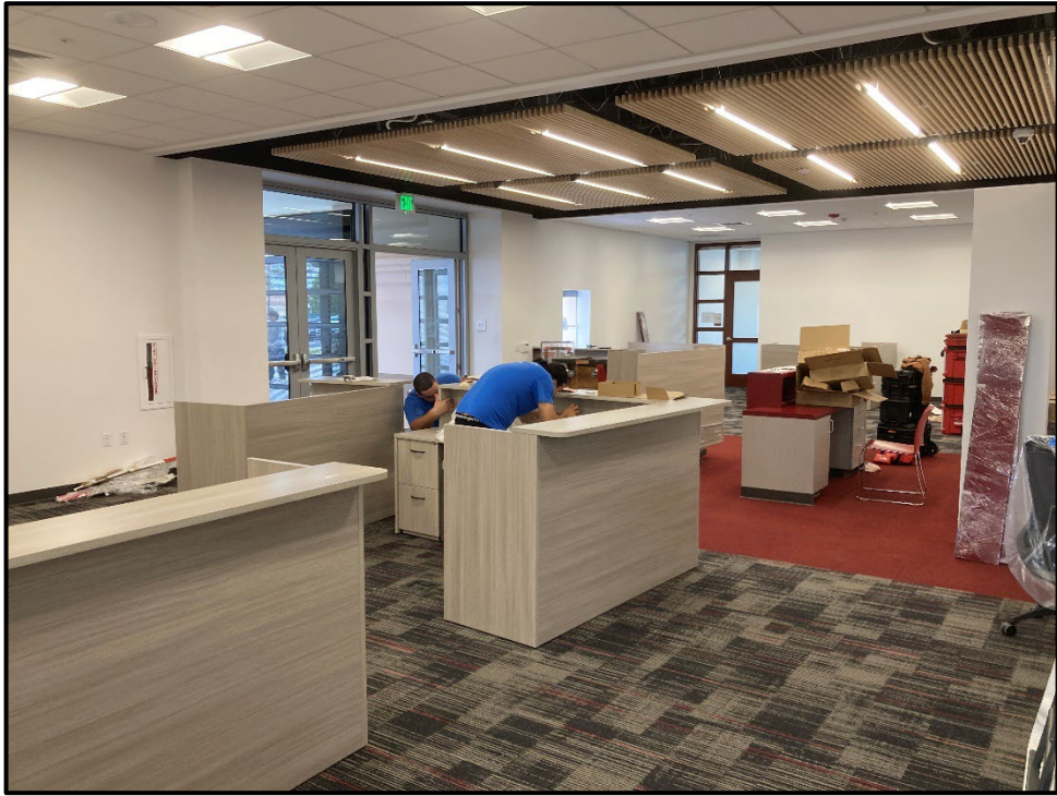
SMHS 50-Classroom Building – Administration Furniture Installation In-Progress
