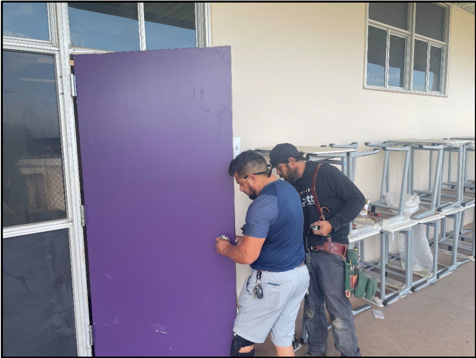
ERHS – Leo Avila and Tom Harbold Repairing Door Hardware
