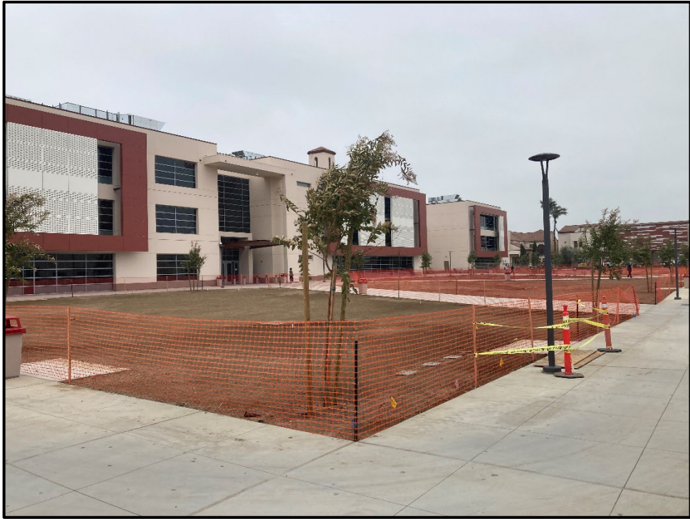
SMHS 50-Classroom Building – Newly Hydroseeded Lawn Begins to Sprout
