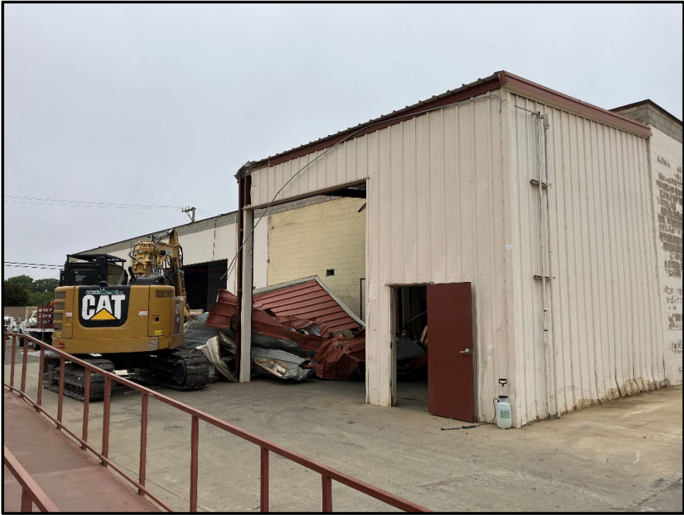
SMHS CTE Modernization – Demolition of Non-DSA Structure at Agriculture Mechanics Shop
