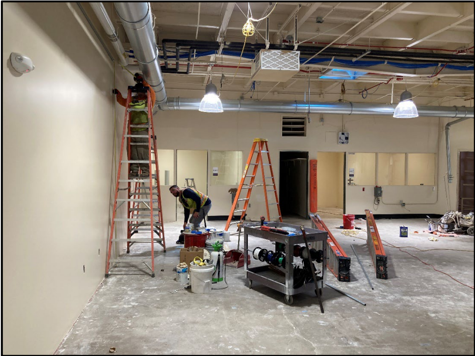
ERHS CTE Modernization – Electrical Power Upgrades Underway
