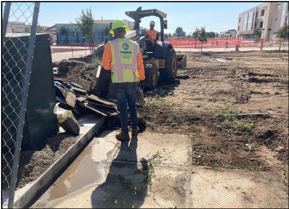
SMHS 50-Classroom Building – Landscaping South of the New Building Continues
