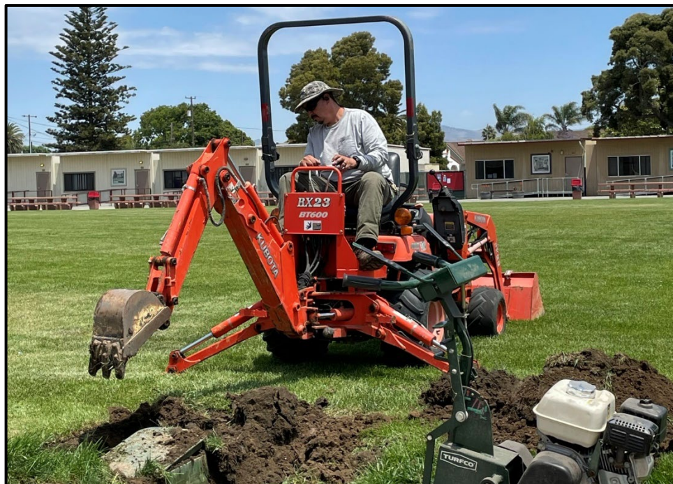
SMHS – Alan Rodriguez Installing New Irrigation Valves in the Practice Field
