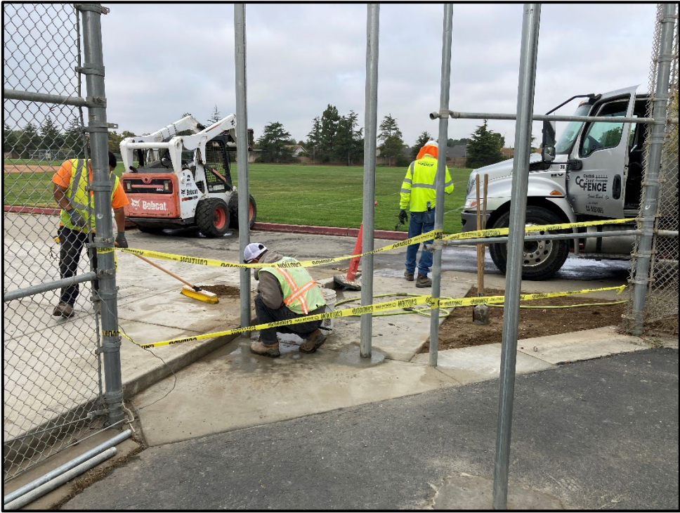
PVHS 10 Portable Classrooms – Installing New Fencing and Gates
