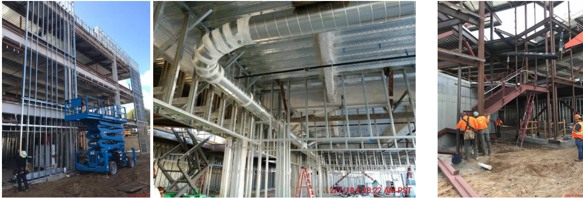
Righetti High School New 38 Classroom Building Construction Progress (February 2018)
