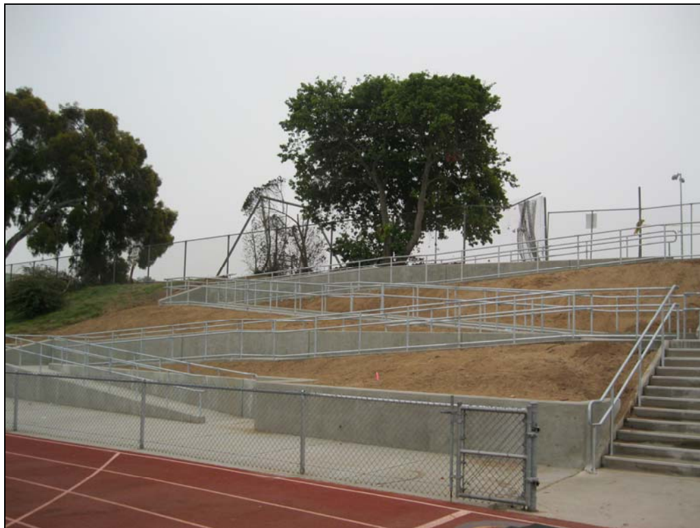
Football Stadium Ramp Before Hydro-seeding ...
