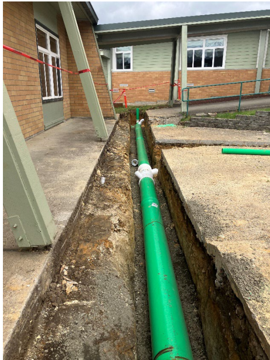
The new courtyard drainage is installed.
