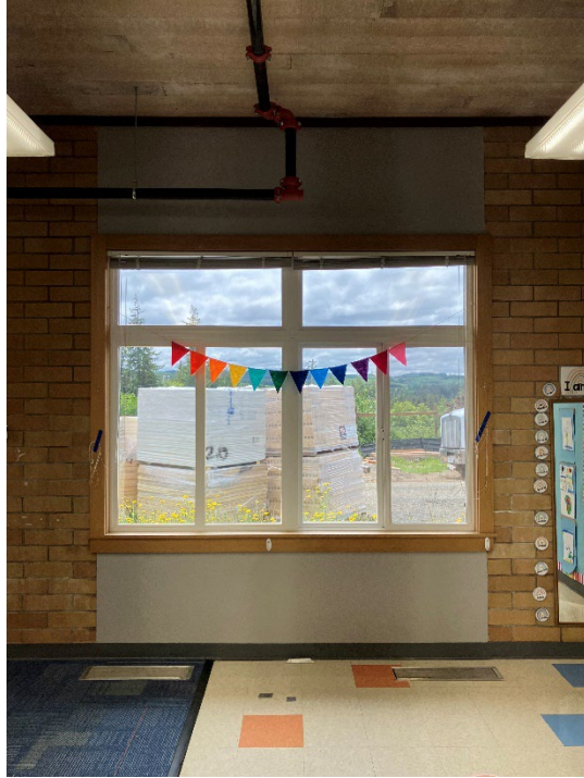
The paint crew is freshening up the HLE classrooms.
