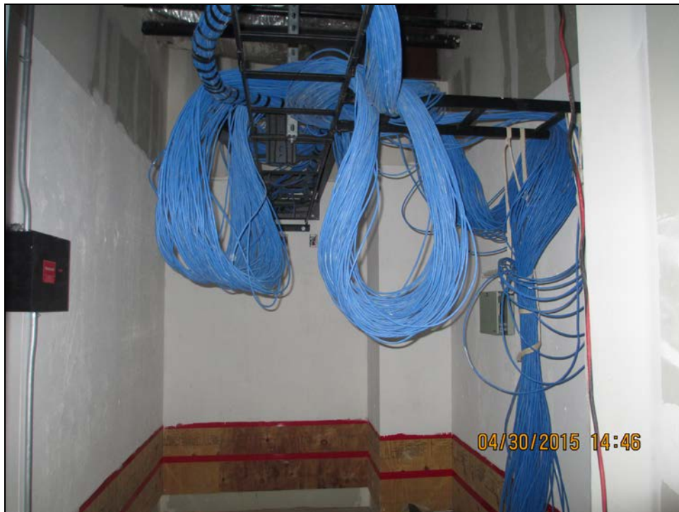
SMHS – Large Quantities of Computer Cable go into the Broadway Classroom Building
