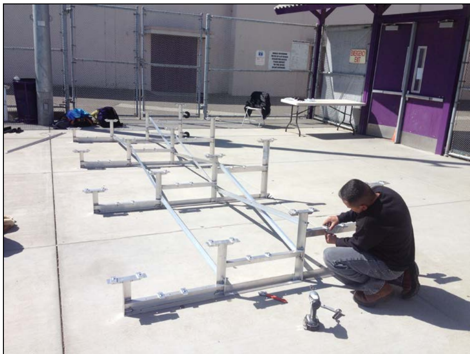
ERHS - Jimmy Salutan Assembles New Bleachers at the Pool
