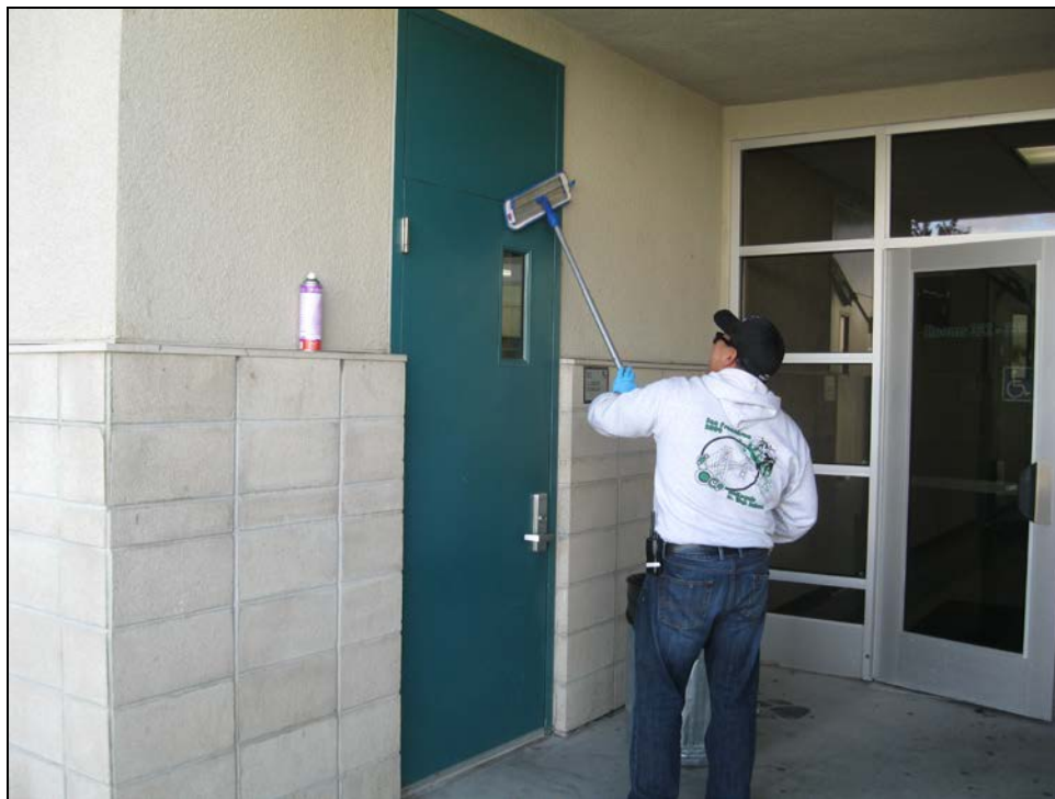
PVHS - José Rivera-Pompa Cleans Exterior Doors During Spring Break
