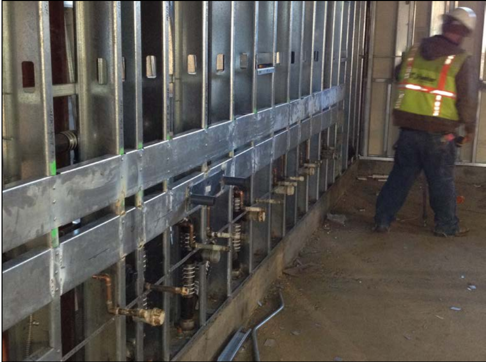
SMHS – 14 Classroom Building Rough Plumbing Underway
