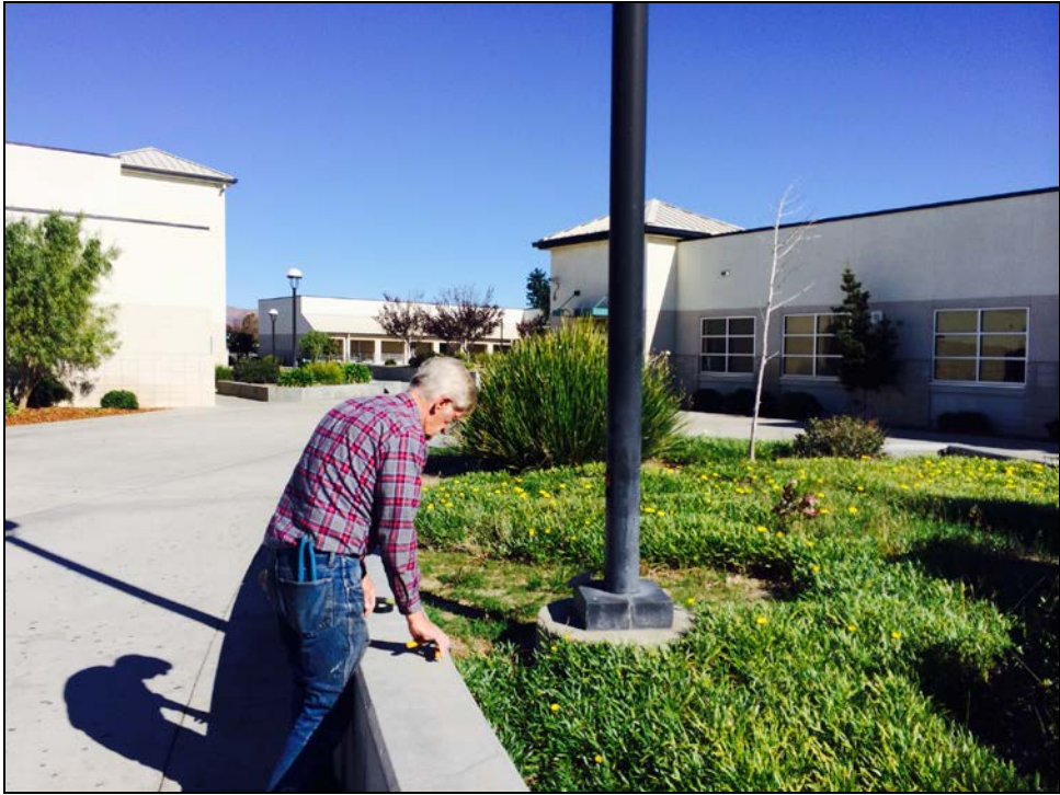
PVHS – John Swanson Repairs the Exterior Lighting in the Quad
