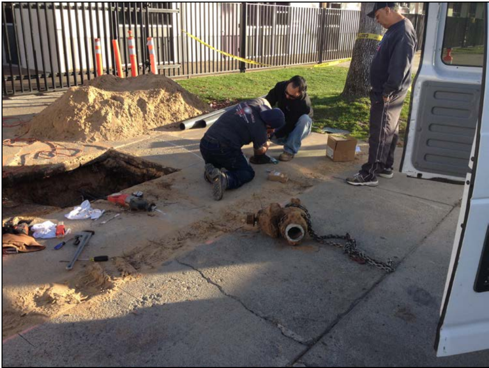
ERHS – Flavio Rodriguez & Ricardo Eliserio Replace a Water Valve Before New Walkway is Poured.
