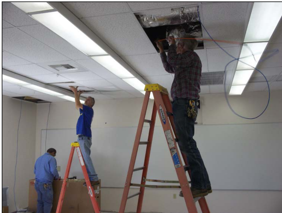
ERHS – District Carpenter and Electricians convert 21 st Century Demonstration Classroom
