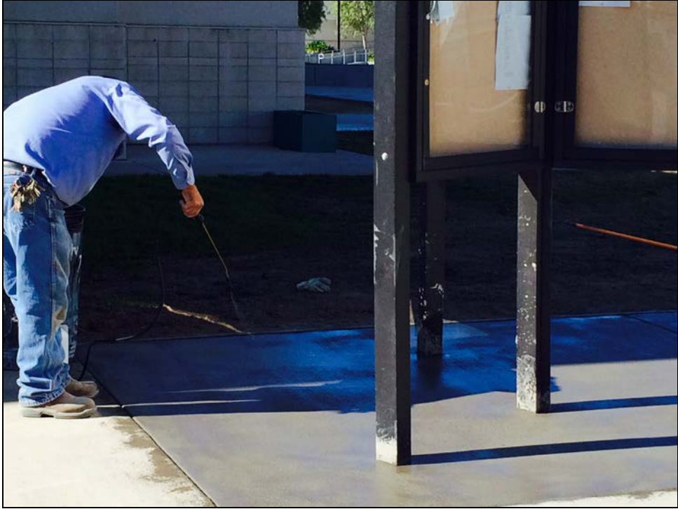
PVHS – José Placencia Finishes Concrete Around a New Information Kiosk
