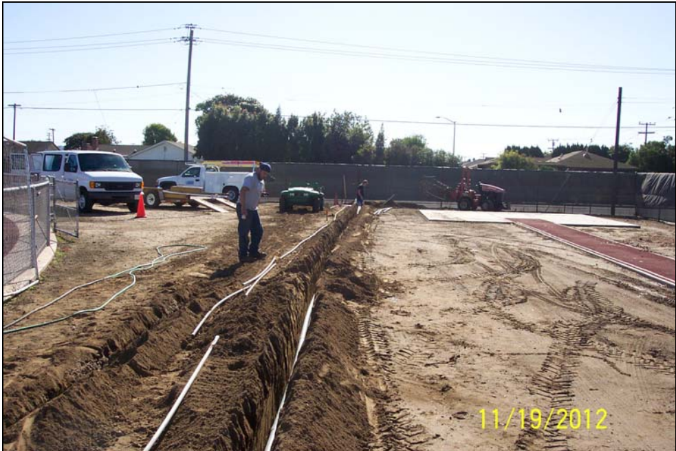
SMHS irrigation pump – preparing electrical and plumbing connections
