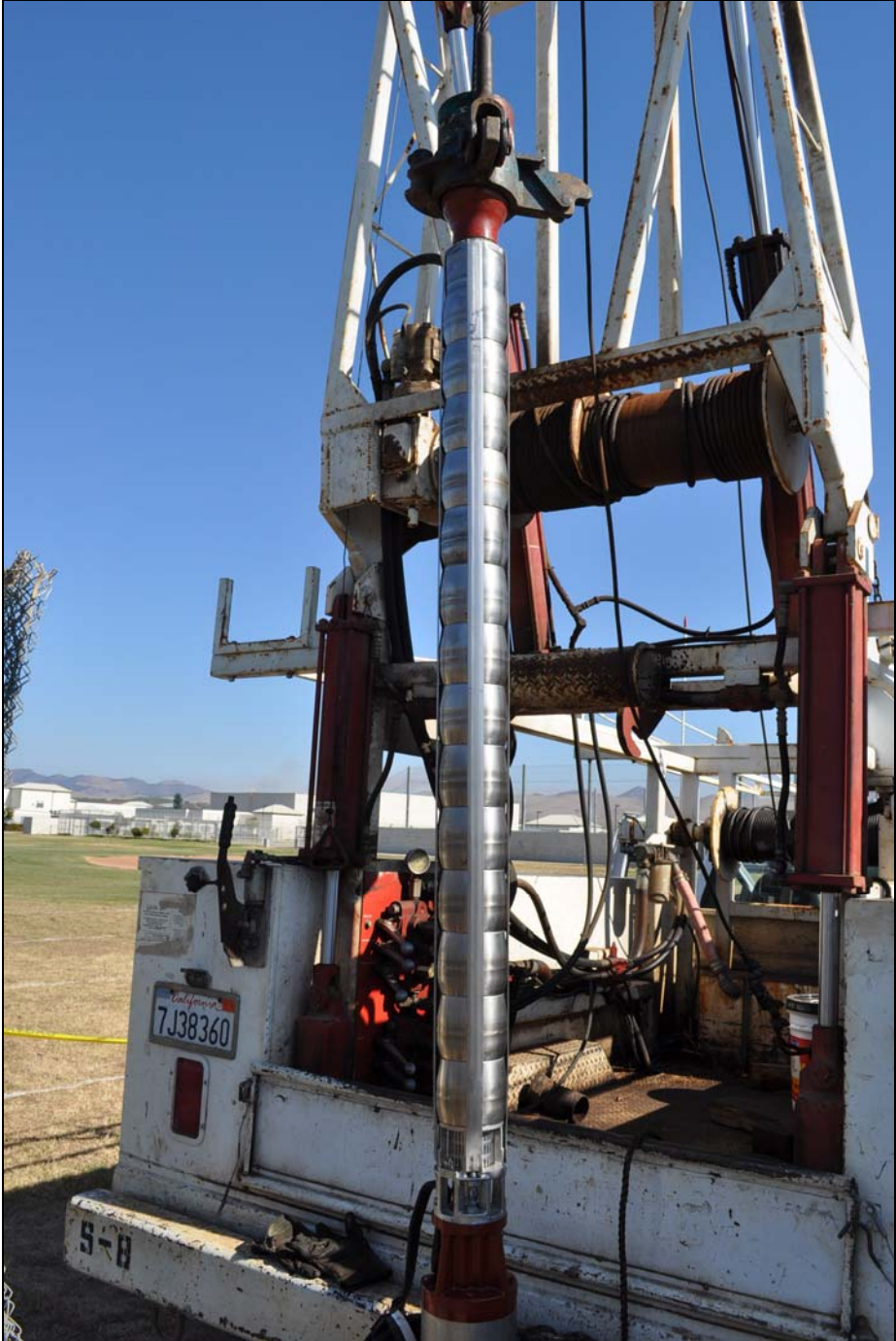
PVHS gets a new irrigation well pump
