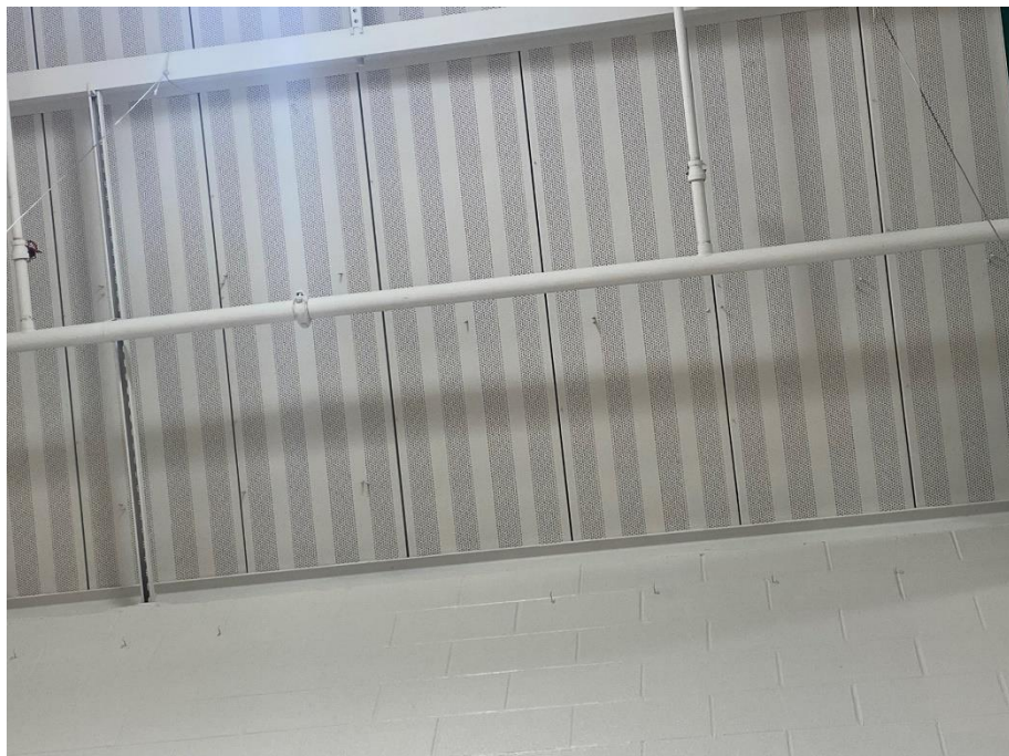
Photo 6: Variations in clip spacing and single screws
