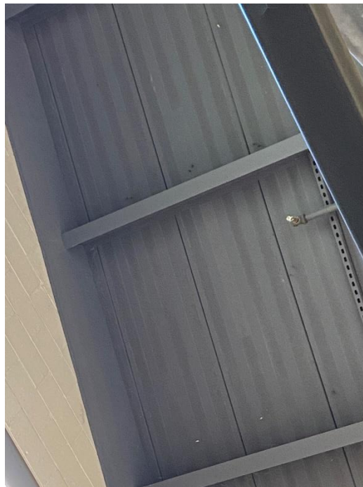
Photo 4: Excessive fastener spacing at gable end
