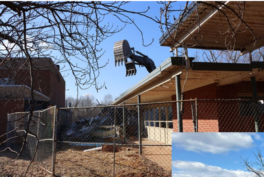
Middle School Demolition
