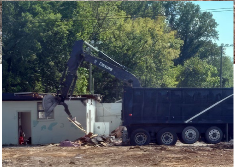
Pool and locker room demolition
