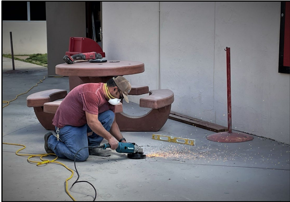
SMHS – Ricardo Eliserio Installing New Concrete Lunch Tables
