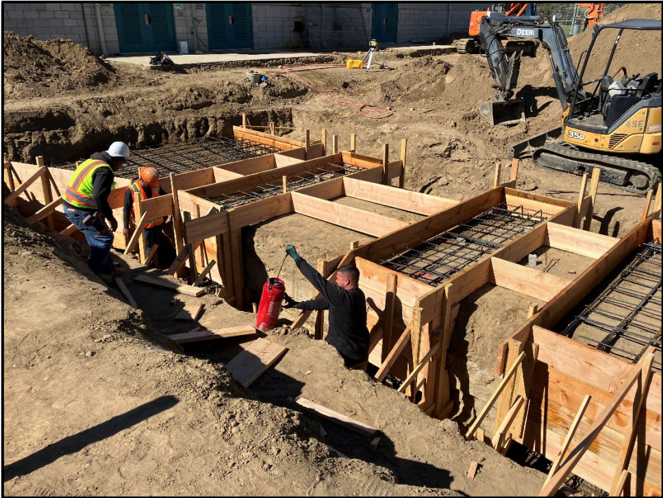
PVHS New Modular Classrooms – Footing Installation Underway
