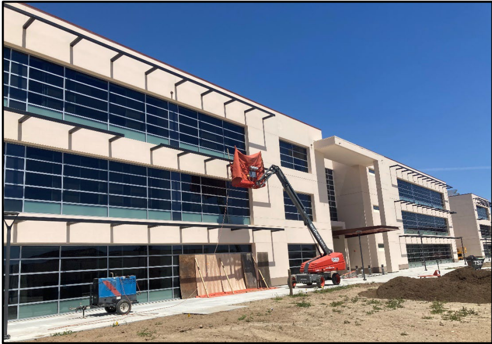
SMHS 50-Classroom Building – Installing Exterior Shade Panels
