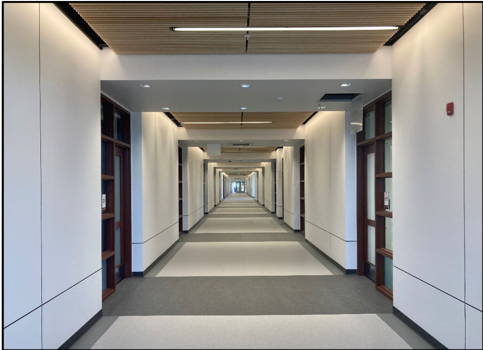
SMHS 50-Classroom Building – Classroom Hallway Nearing Completion
