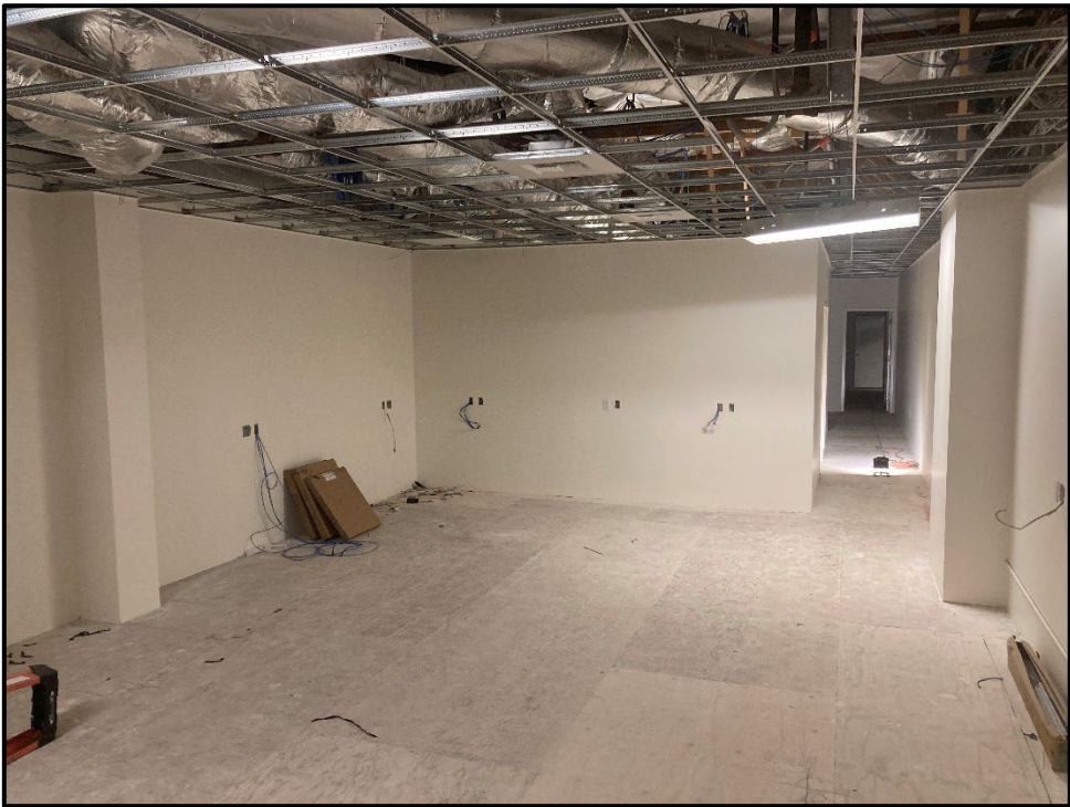
SSC Second Story Reconfiguration – Drywall and Ceiling Grid Installation Continues
