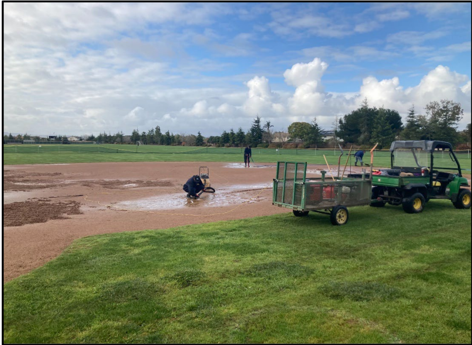
PVHS – Grounds Crew Pumping Rainwater at the Junior Varsity Softball Field
