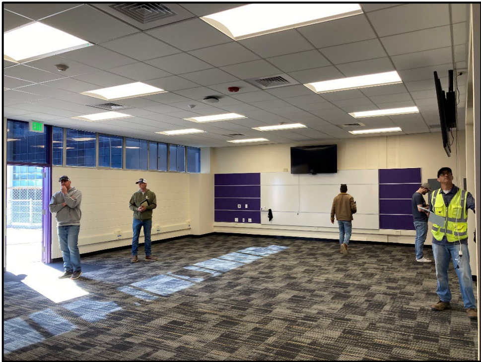
ERHS Modernization – Phase 2 Completion Punch List Walk
