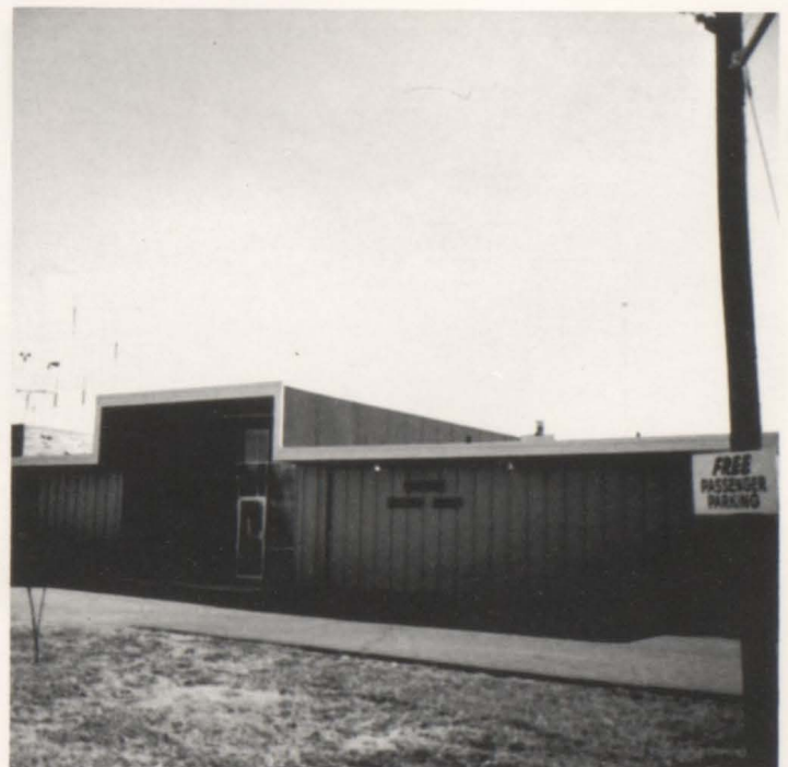
Crossville has recently acquired a new municipal airport building and daily Southern Airways flights.
