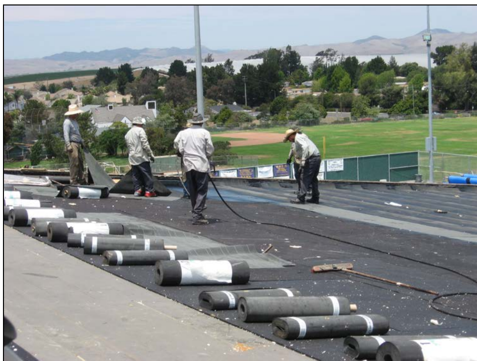
ERHS – Adhesive is Applied Between Each Layer of Roofing Ply
