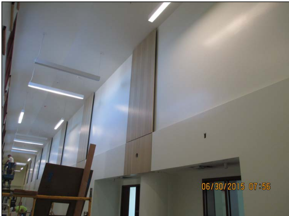
SMHS – Broadway Classroom Second Story Hallway Receives Final Finishes
