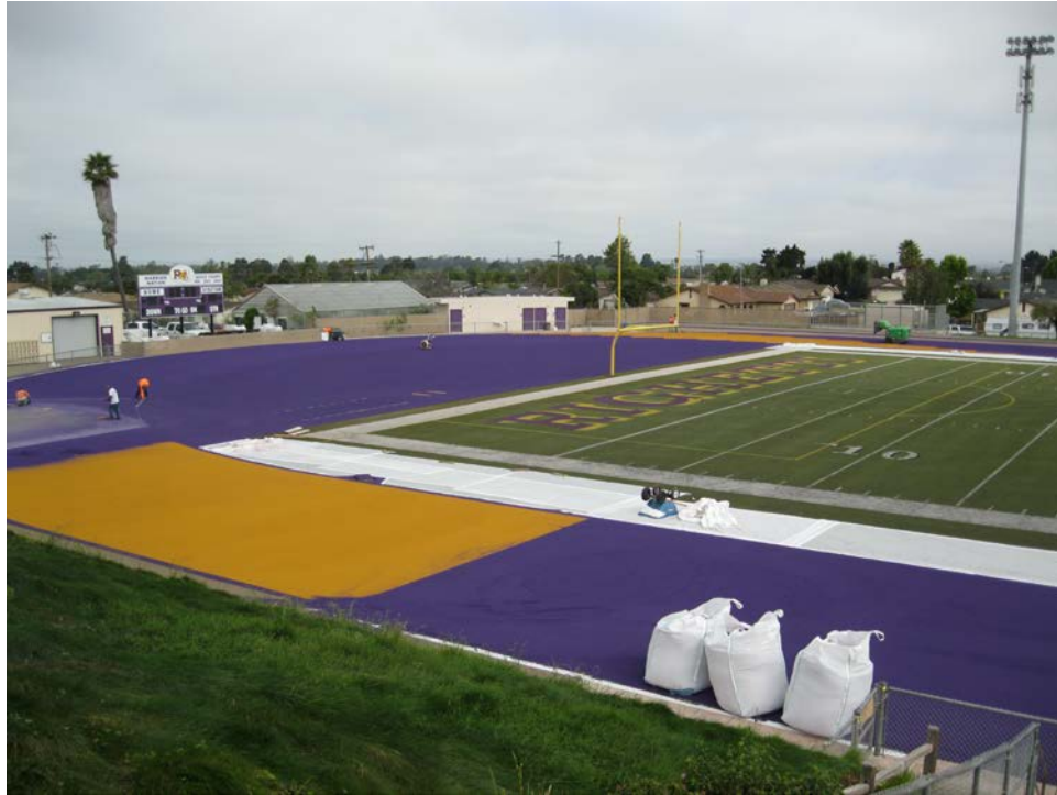
ERHS - Track Resurfacing: the new Rubber is Applied Over the Slurry Coat
