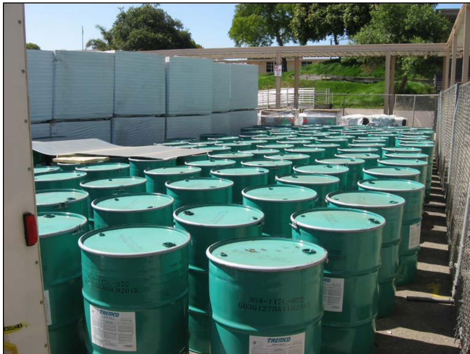
ERHS – Gymnasium Roof: Stacks of Insulation Many Barrels of Burmastic® Adhesive
