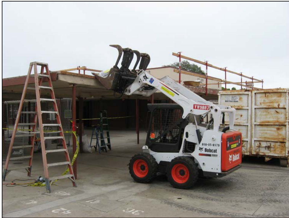
SMHS - Breezeway Canopy Removal Underway
