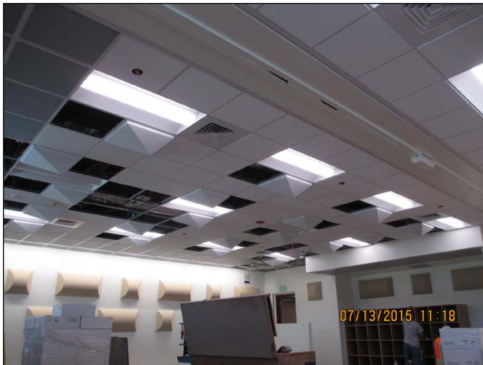
SMHS – Broadway Classroom Building Band Acoustic Panels Installed
