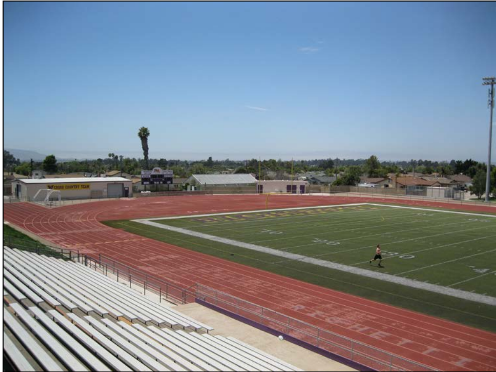
ERHS – Track Before Resurfacing
