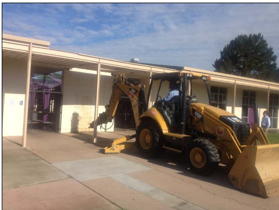
ERHS – Jose Placencia Prepares to Demolish a Block Wall to pen the Campus Traffic Flow
