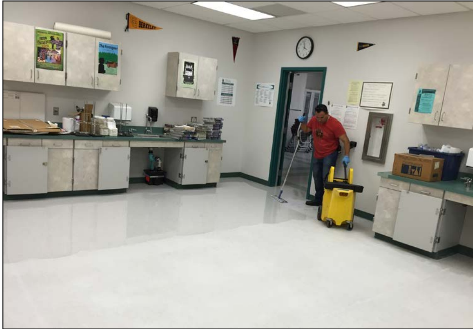
PVHS – Jose Rivera-Pompa Applies a Coat of Floor Finish to the Scrubbed Floor
