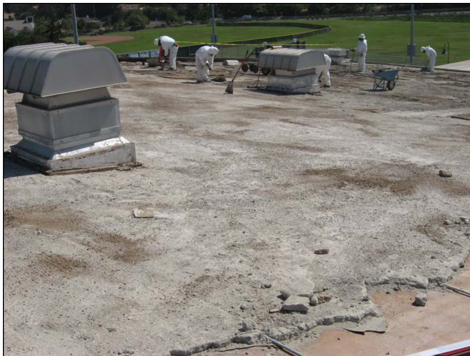
ERHS - Gymnasium Roof Tear-off in Progress
