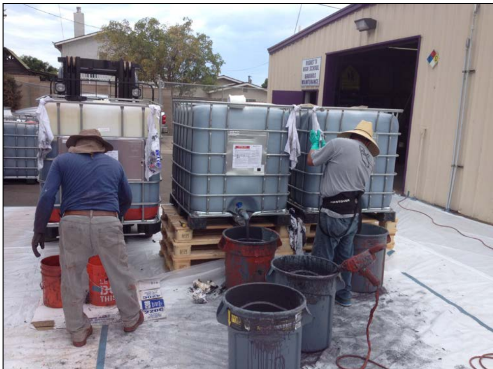
ERHS – Track Resurfacing: Gallons and Gallons of Slurry to Mix and Apply
