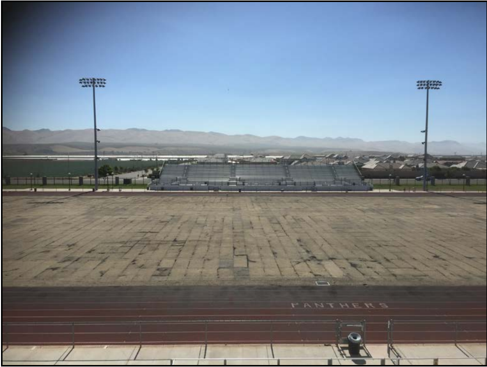
PVHS Stadium – Turf and Underlayment Removed and Ready for New Turf
