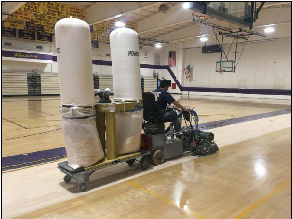
ERHS - Resurfacing the Gymnasium Floor Begins ...
