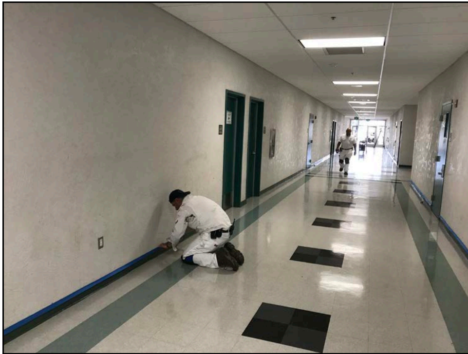
PVHS – Ernest Paz and Ray Segovia Repair and Repaint a Classroom Hallway
