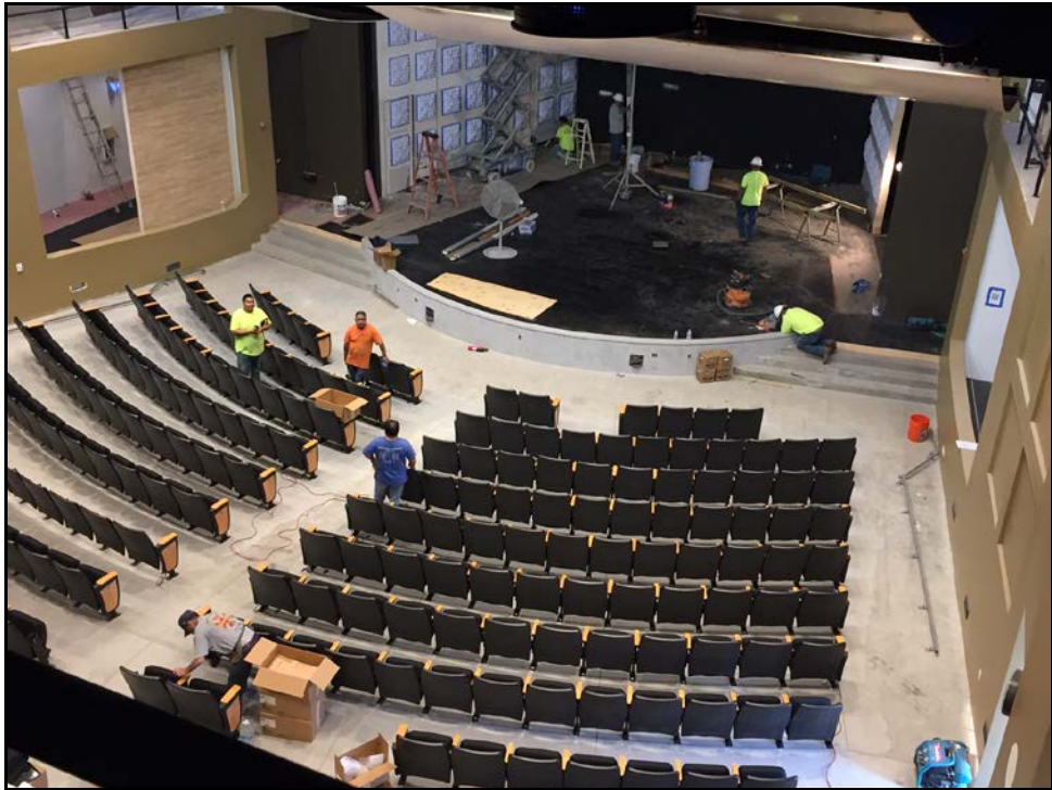
... Floor is Sealed and Audience Chair Installation Underway
