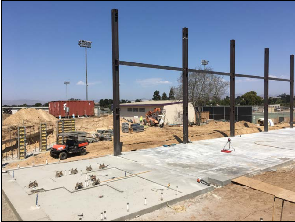
ERHS 38 Classroom Building - Plumbing in Place and First Floor Concrete Poured
