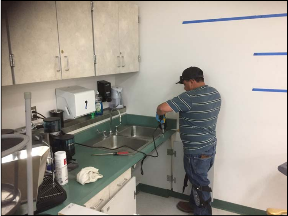
PVHS - Jesus Reyes Installs Upgraded Sinks and Faucets in the Foods Lab
