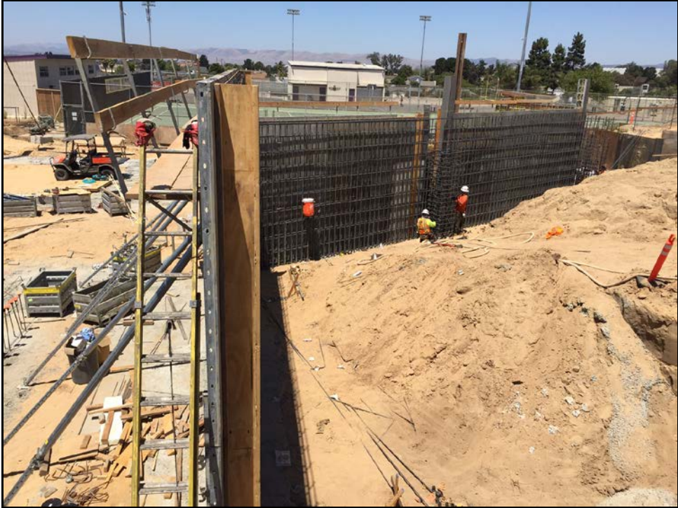
ERHS 38 Classroom Building – Forming Retaining Walls
