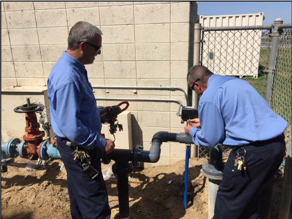
ERHS – Del Ward and Andy Freitas make Final Adjustments on New Irrigation Controls
