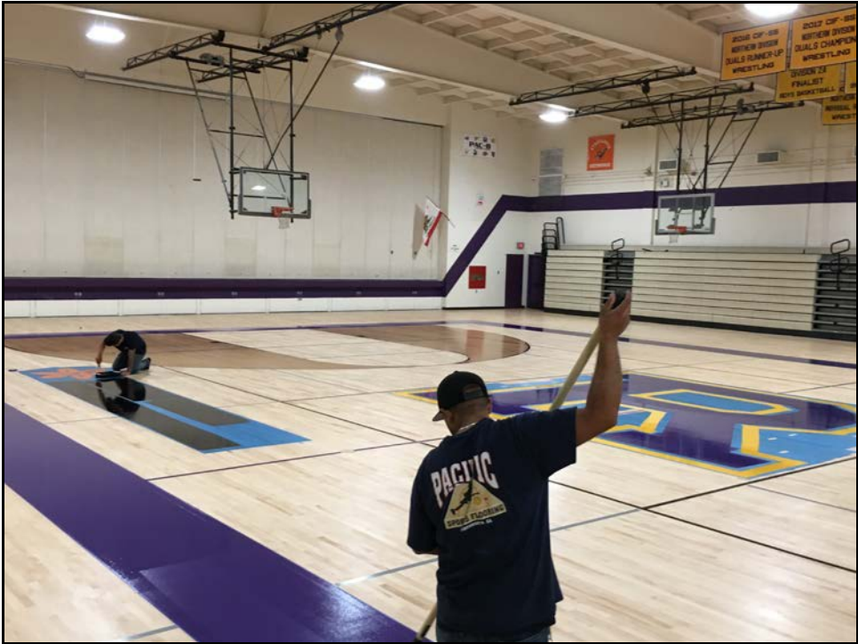
... Resurfaced Floor Gets all New Paint
