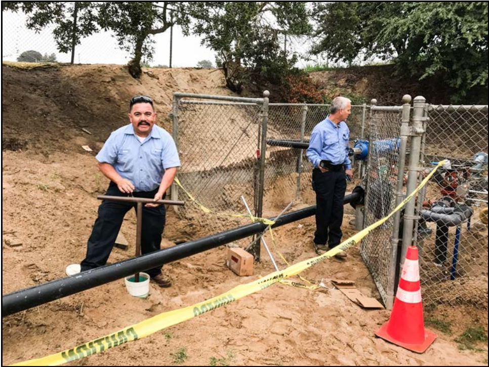
ERHS – Jesus Reyes and Del Ward Set up Temporary Irrigation to the Play Fields
