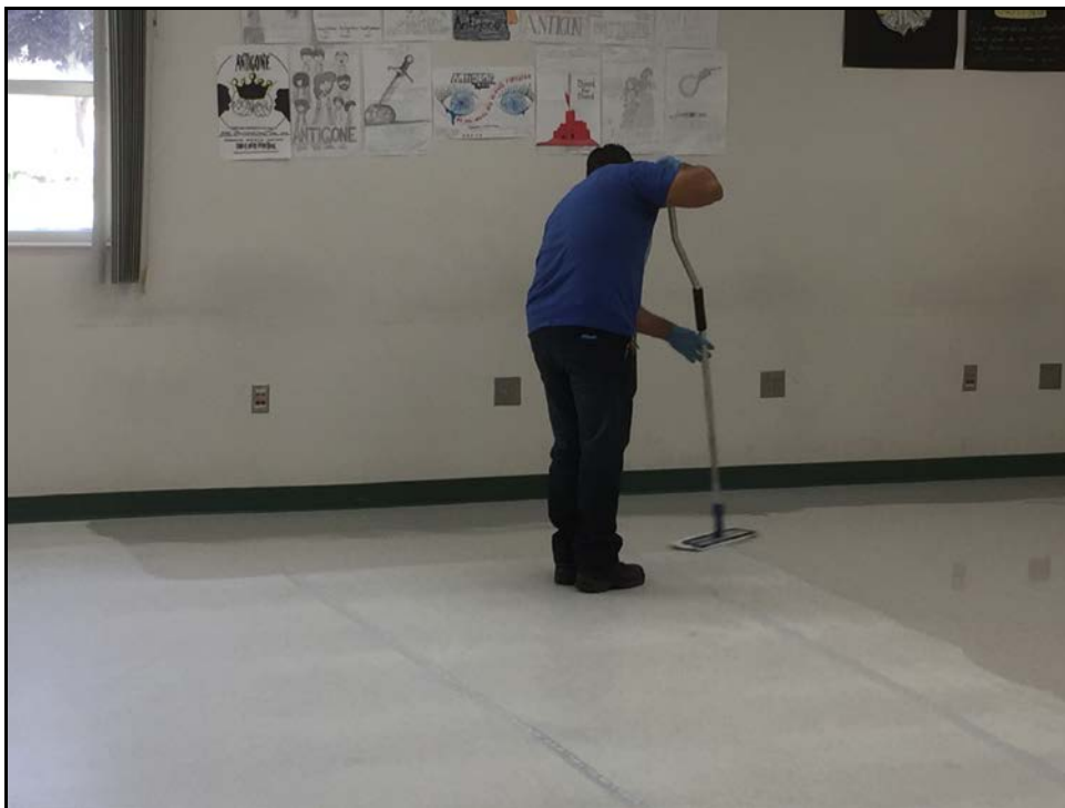
PVHS – Manuel Pompa-Rivera Uses the KaiMotion to Apply Floor Finish in a Classroom
