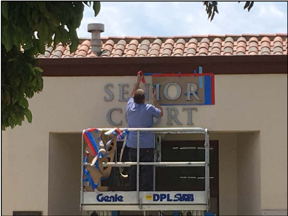
SMHS - Erik Fulton Installs Letters for the Senior Court Near the Administration Building
