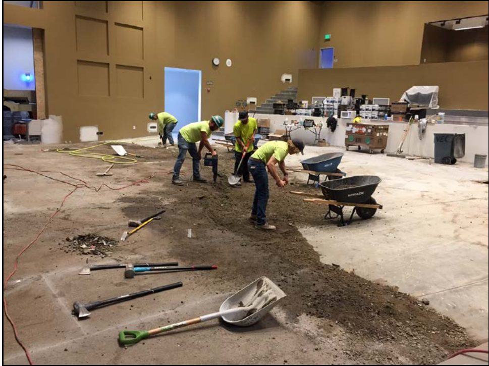
PVHS Performing Arts Center – Laborers Remove the Earth Protecting the Audience Floor During Construction ...
