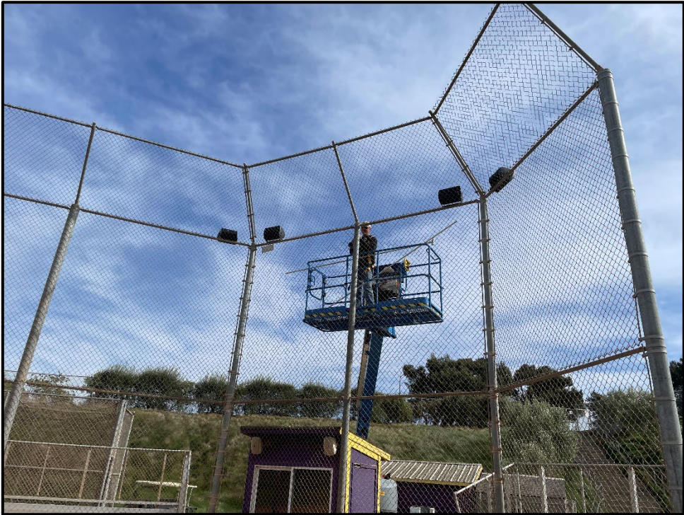
ERHS – Del Ward Installing the New Sound System
