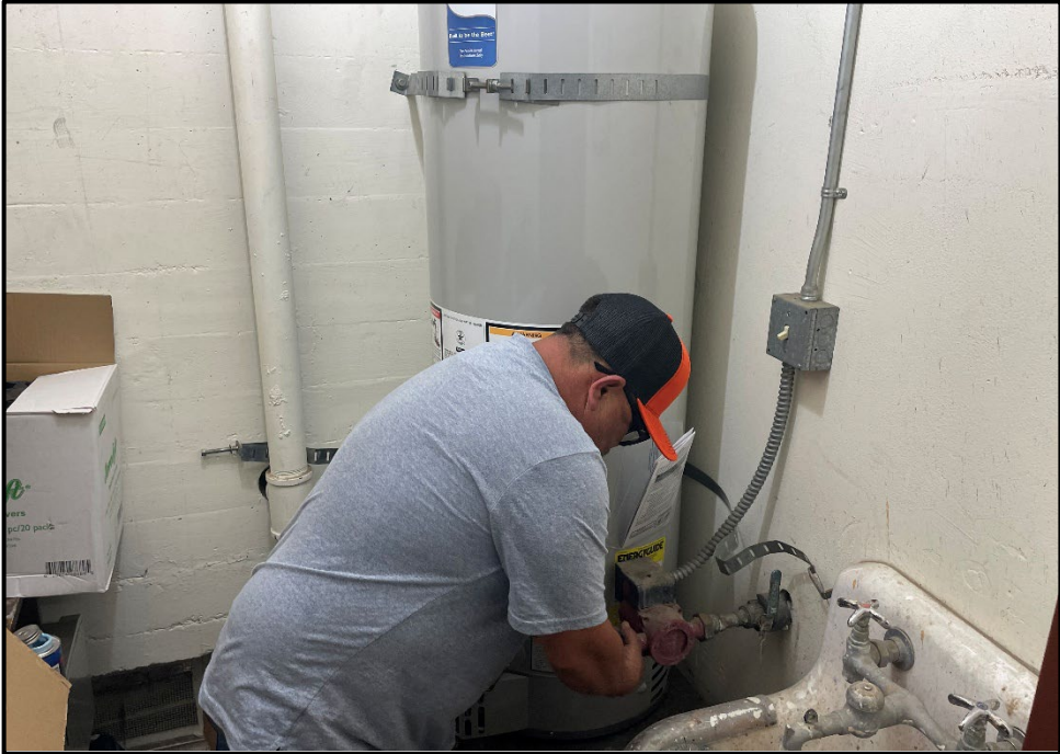
SMHS – Jesus Reyes Replacing the Water Heater in the Wilson Gym
