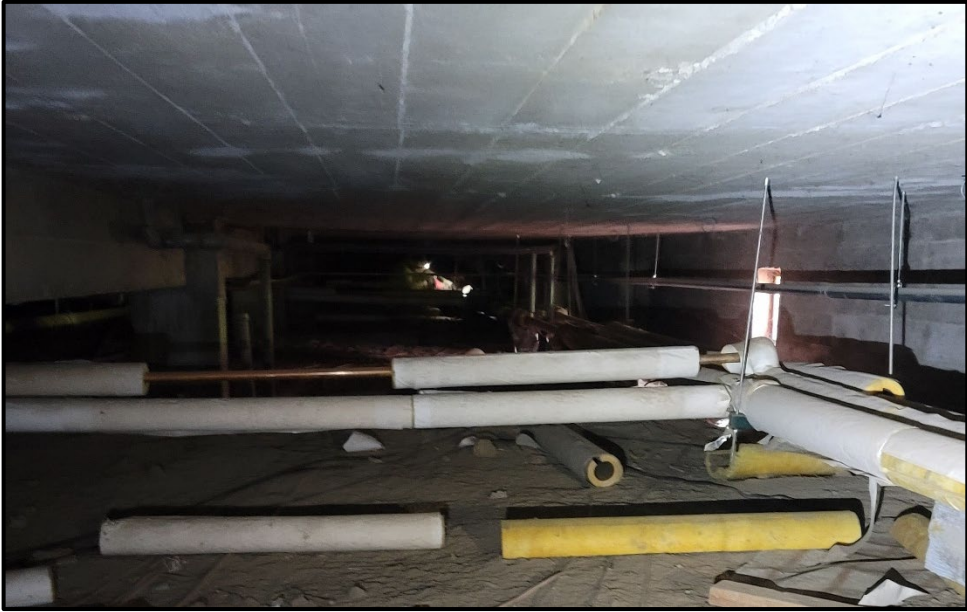
SMHS Admin to Classroom – Underground Conduit Being Installed
