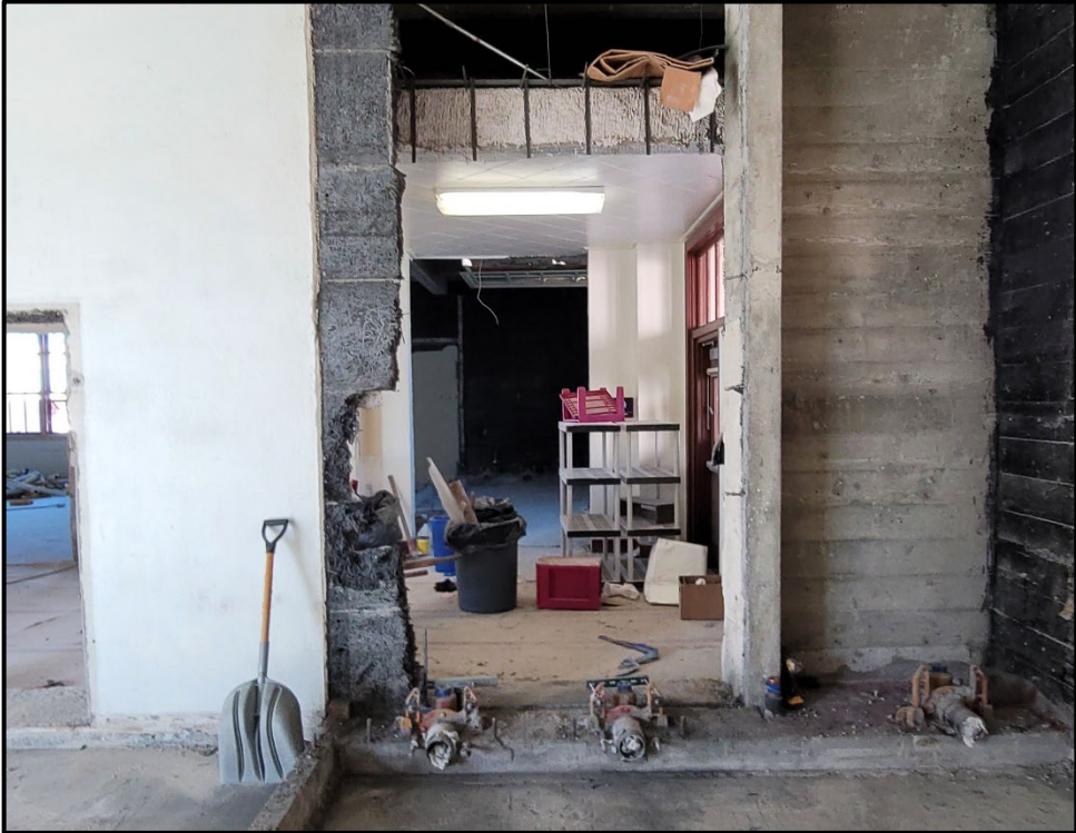
SMHS Admin to Classroom – Demolition Continues in the Old Administration Building
