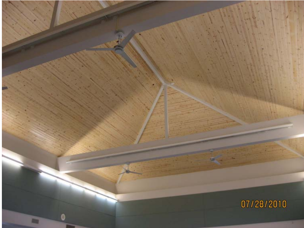
New tongue and groove ceiling – Pioneer Valley High Cafeteria
