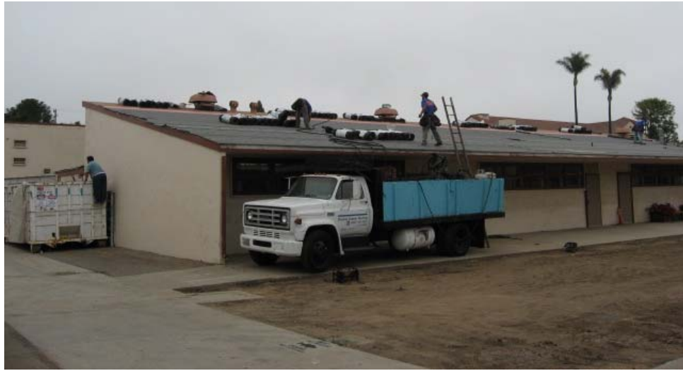
New Roof – Santa Maria High Arts and Crafts
