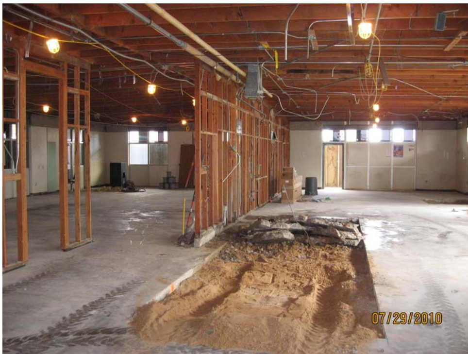
Early demolition at the Administration Building – Righetti High
