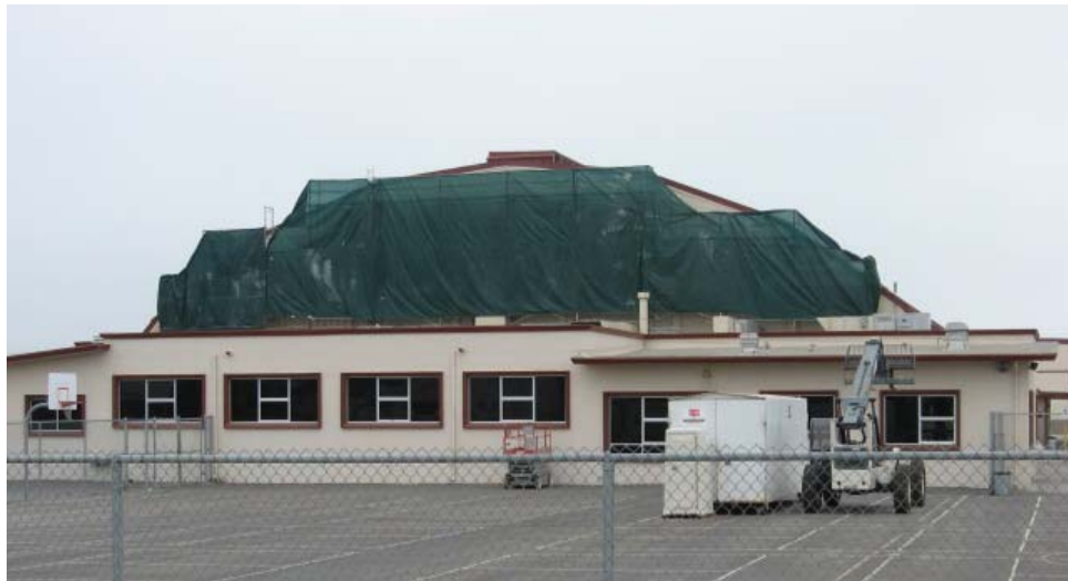
Lead paint removal for mural – Santa Maria High Wilson Gym
