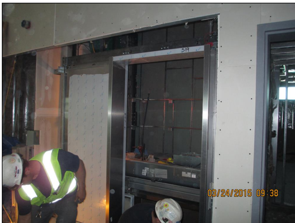
SMHS – Elevator Installation for the Broadway Classroom Building
