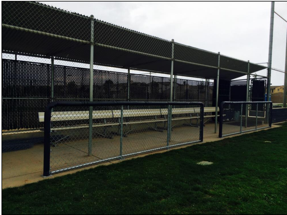
PVHS – Revised Varsity Baseball Dugout: Safety Rail and New Roof
