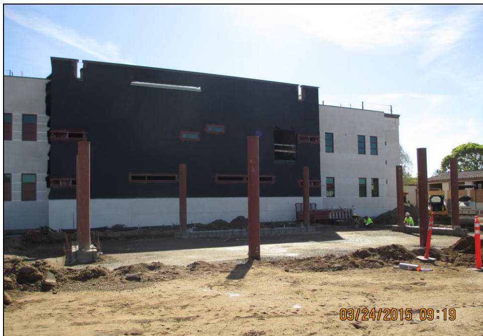
SMHS – Broadway Classroom Building Student Pavilion Takes Shape
