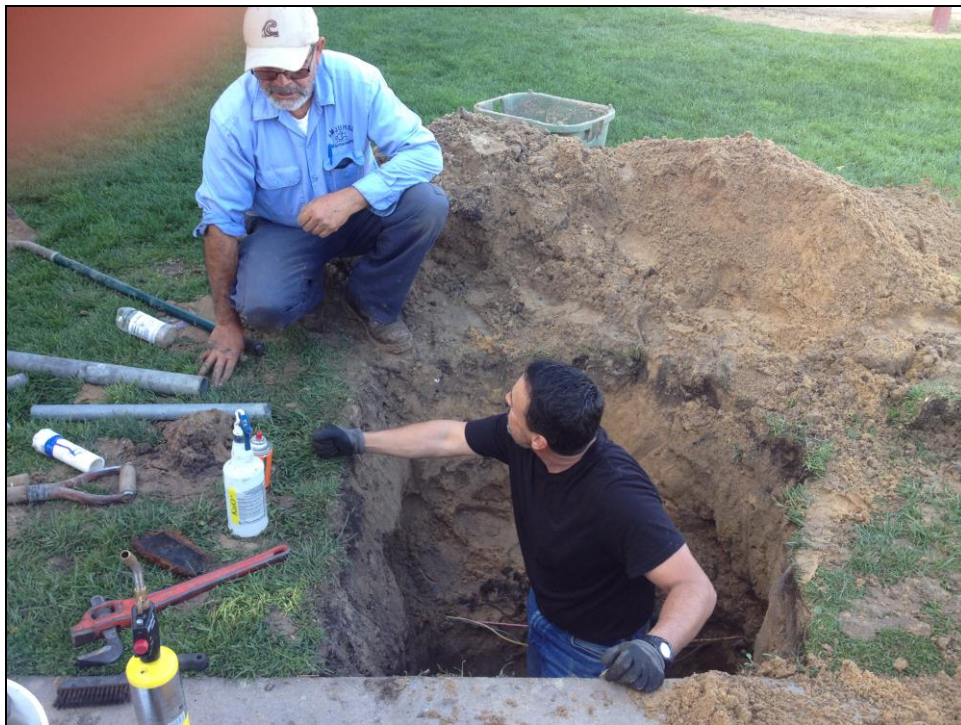
EHRS - Bernie Rayner and Juan Rodriguez Repair a Broken Water Line in the Quad Area
