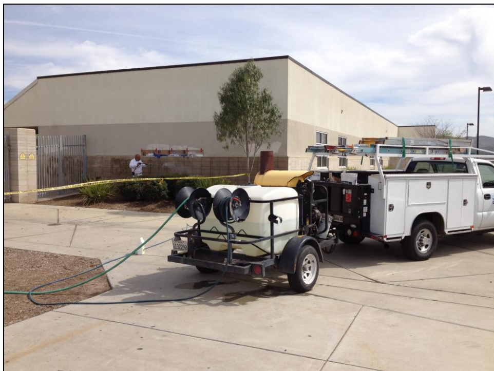
PVHS - Ray Segovia Power washes Graffiti from the Cafeteria
