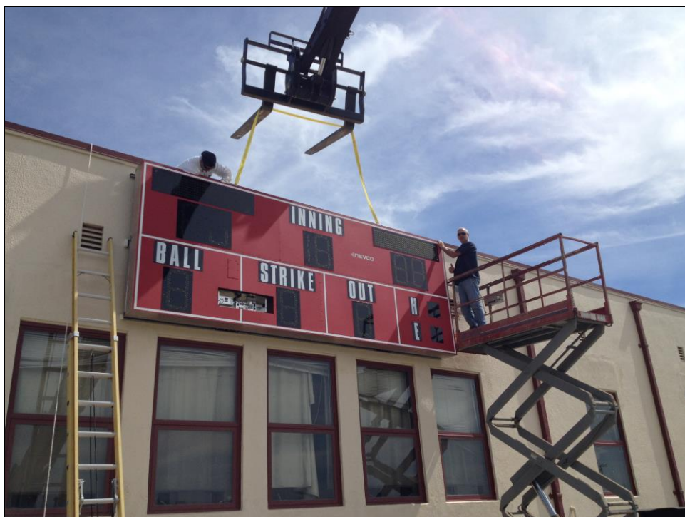
SMHS – Del Ward and Ernest Paz Secure the New Softball Scoreboard While José Placencia Hoists it in Place
