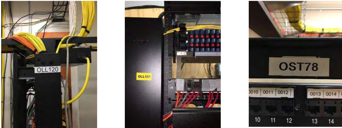
Figure 12: Samples of Equipment Rack Label
