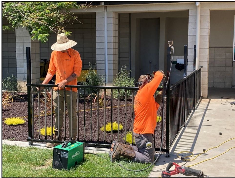
PVHS - Fencing is Installed at the Gymnasium to Protect the Campus Planters
