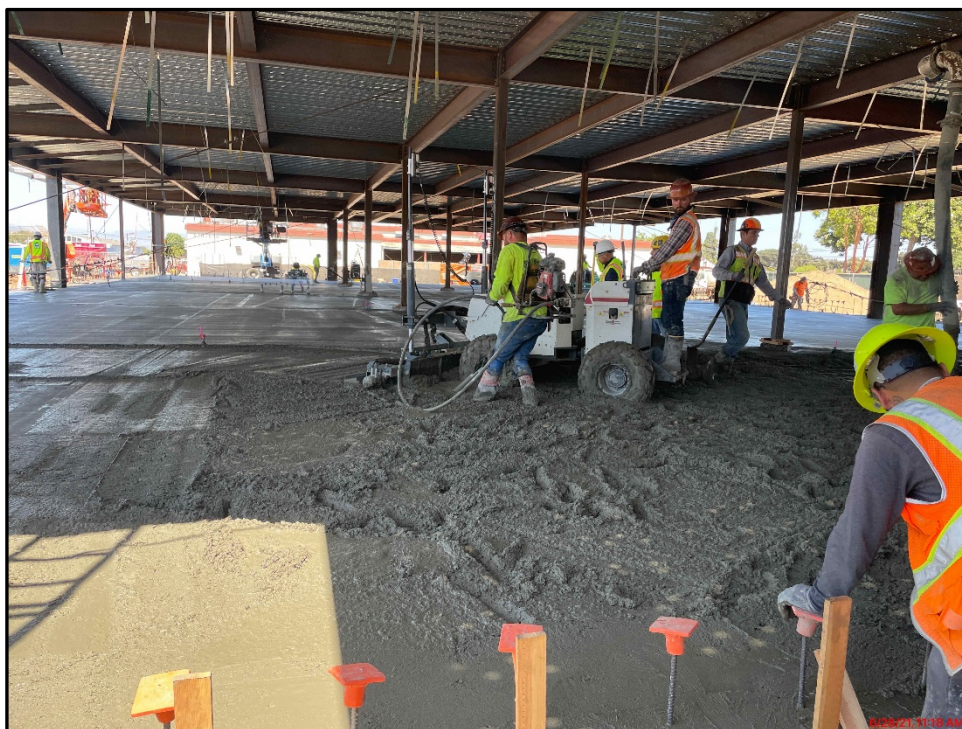
SMHS 50-Classroom Building – More Than 1,000 of Yards of Concrete Create the First Floor
