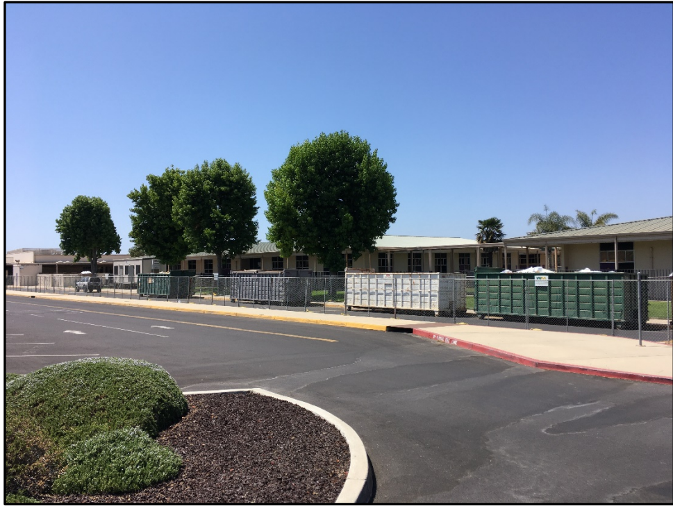
ERHS Modernization – Contractor Laydown Area and Fencing are Set in Place
