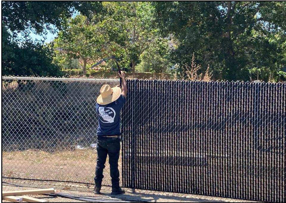
PVHS –José Gamino Installs Privacy Slats in the Softball Outfield Fence to Provide a Windscreen
