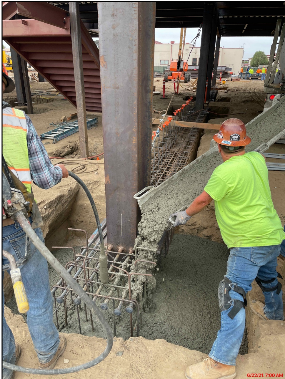
SMHS 50-Classroom Building – Concrete Pour in Progress. Agriculture Science Building in the Background
