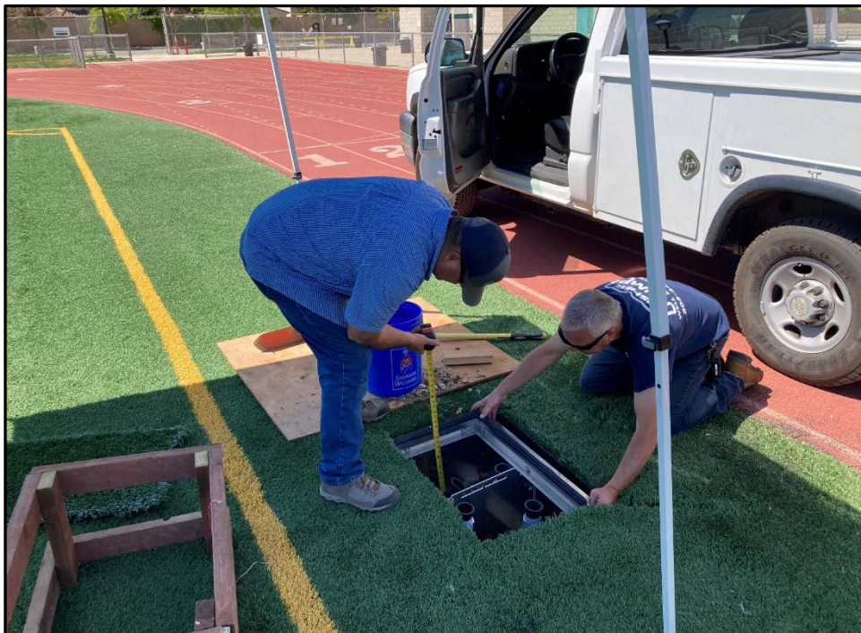
PVHS – Andy Freitas and Del Ward Prepare to Pull Communications and Power Wire into the Stadium Field
