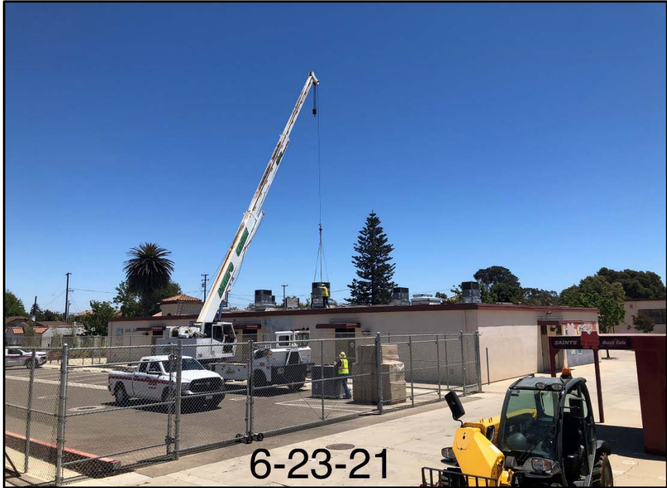
SMHS 240 Science Building – New HVAC Units are Craned into Place
