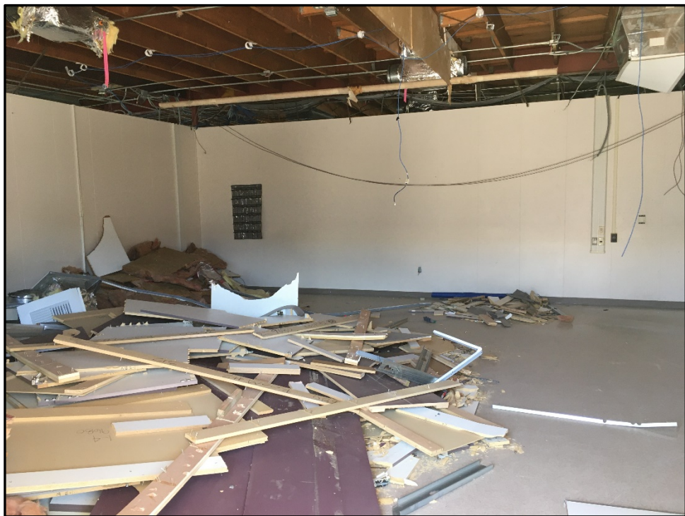
ERHS Modernization – 21 st Century Classrooms Begin with Demolition of Interiors
