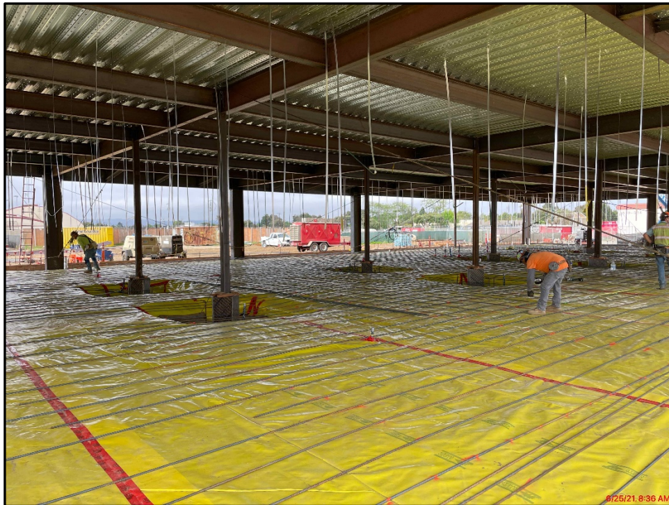
SMHS 50-Classroom Building – Preparing the Ground Floor for Concrete
