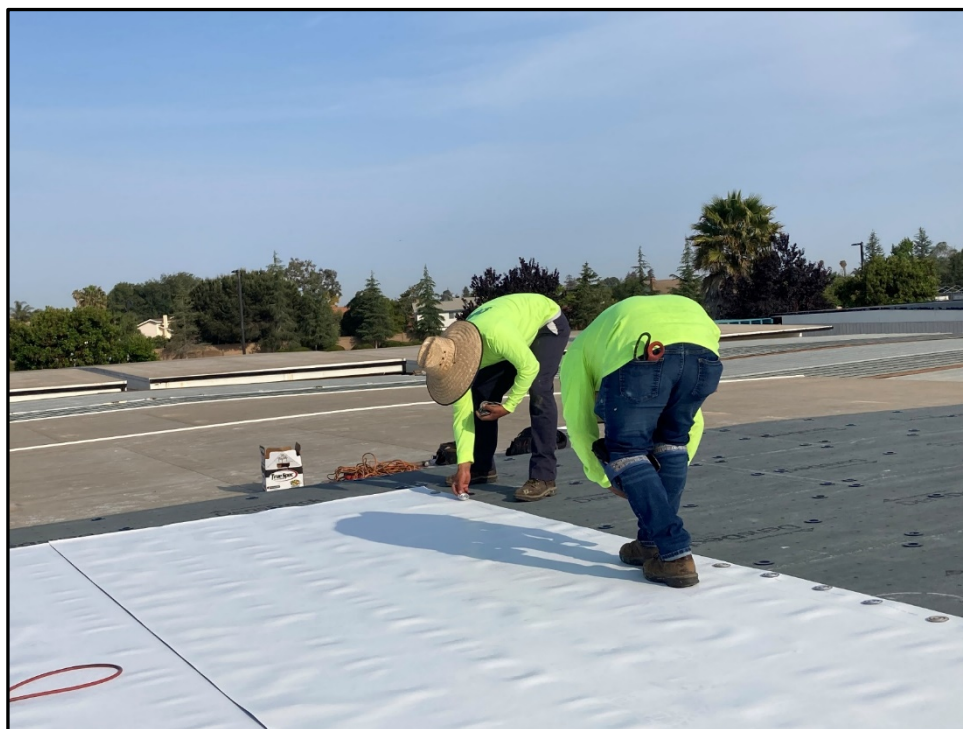
PVHS - Classroom 608 and 610 Receive New Roofs
