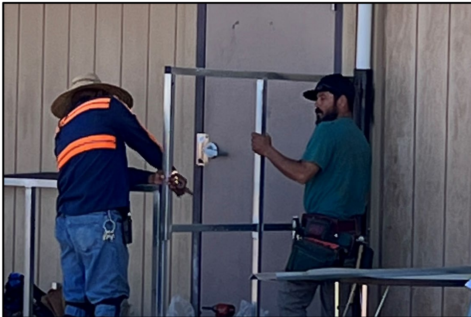
SMHS – Tom Harbold and Alex Anguiano Replace Portable Classroom Ramps
