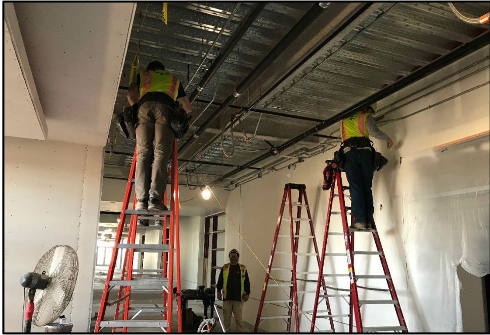
SMHS 50-Classroom Building – Fire Sprinkler Progress and Electrical Work in the Hallways
