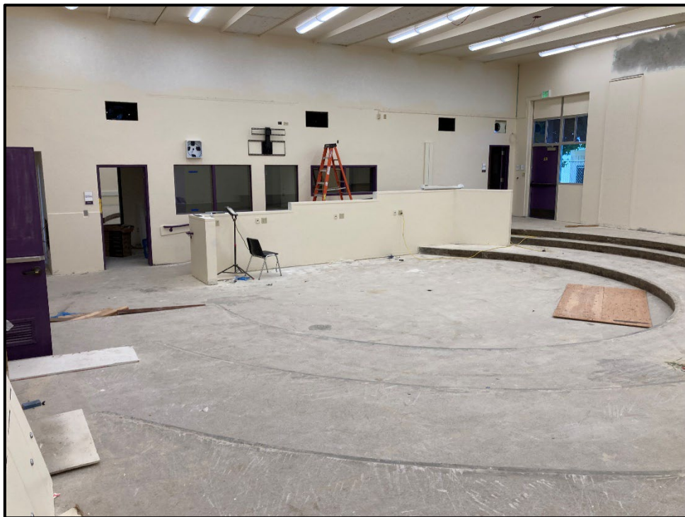
ERHS Modernization – The Band Room Receives New LED Lighting and Awaits Carpet
