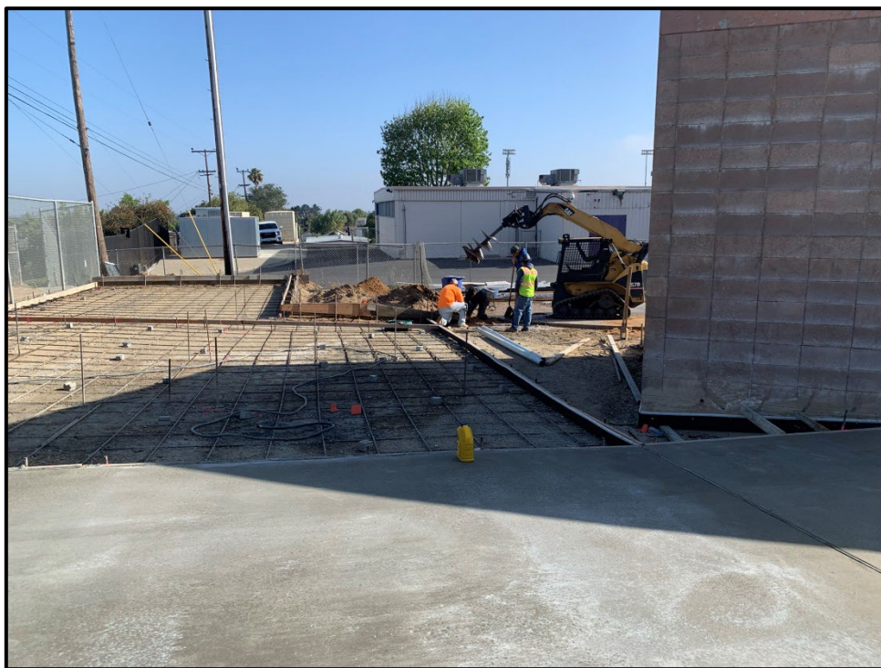
ERHS M&O Building – Maintenance Yard Parking Takes Shape
