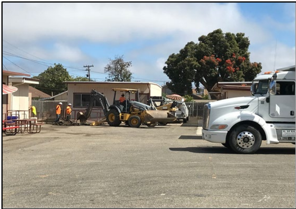
SMHS Lincoln Center – Paving Demolition Begins
