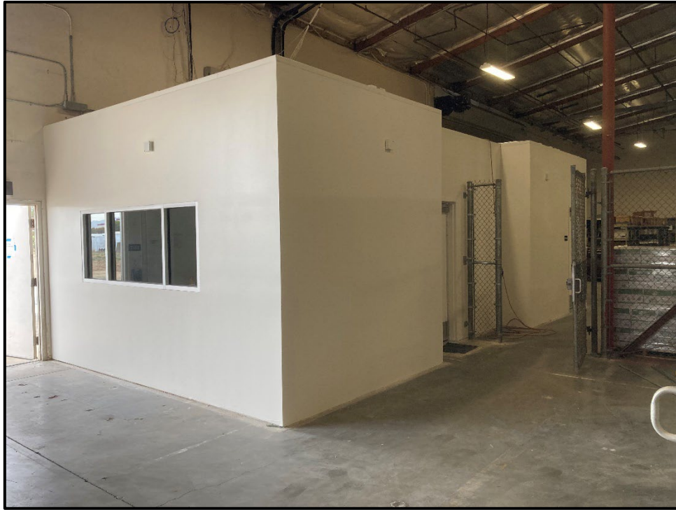
SSC Purchasing Office – Expanded Office Space Nears Completion
