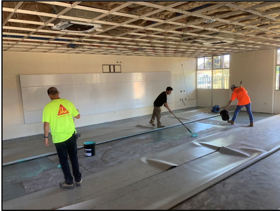
ERHS Modernization – New Hybrid Resilient Carpet Replaces Floor Tiles
