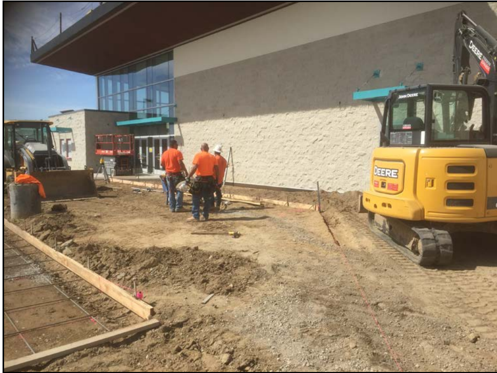
PVHS Performing Arts Center – Concrete Walkway Installation in Progress
