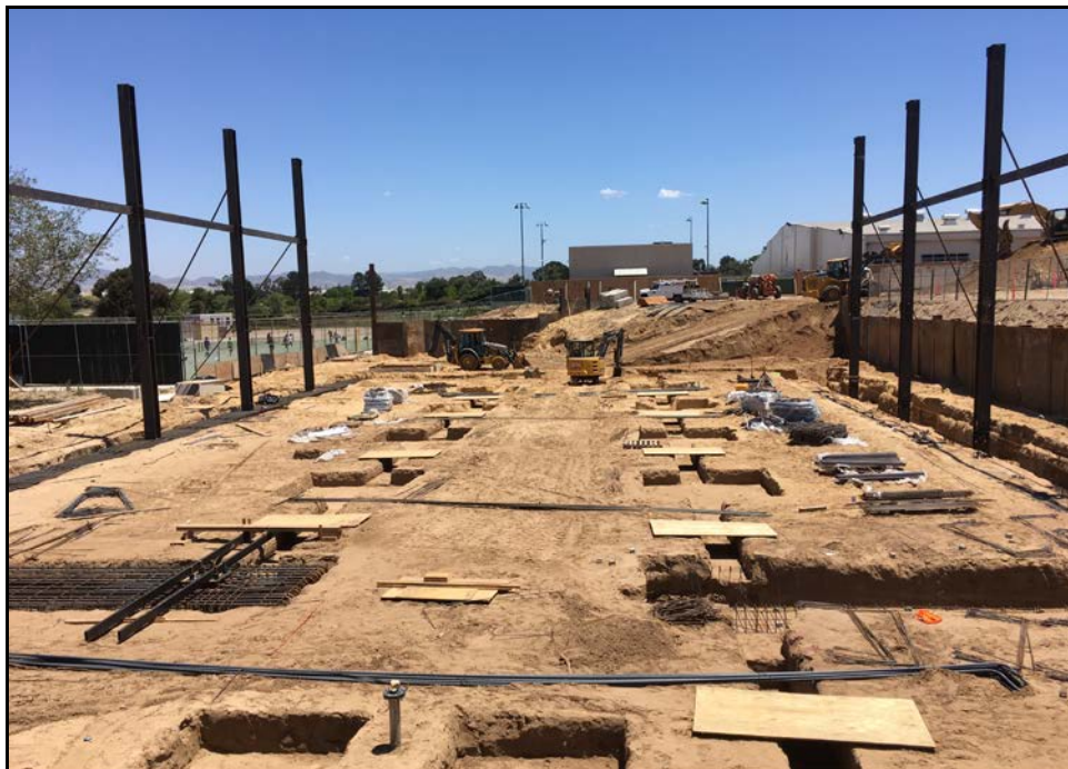
ERHS 38 Classroom Building – Forming for Concrete Footing Begins
