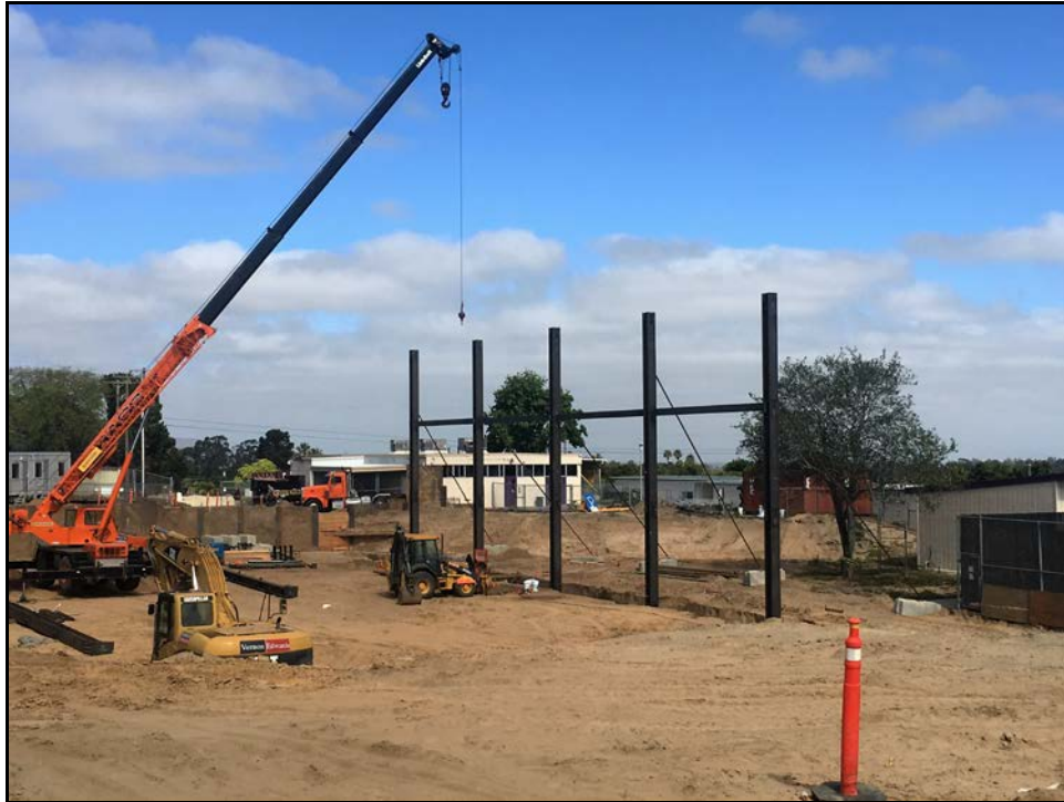
ERHS 38 Classroom Building – Steel Columns Being Placed on the Concrete Footings
