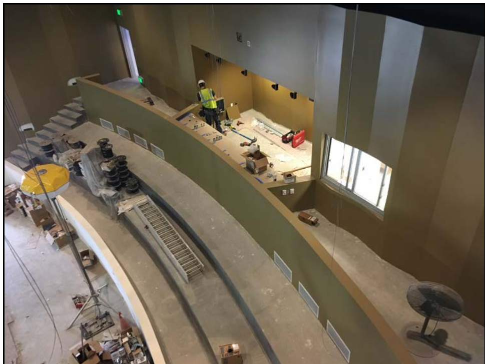
PVHS Performing Arts Center – Interior Finishes at the Sound Booth
