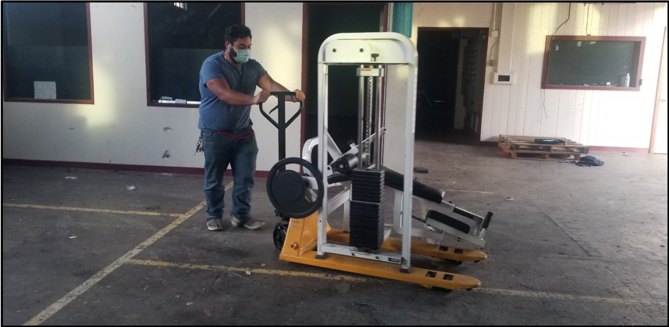
SMHS – Abraham Vasquez Clears Weight Machines from the Old Wood Shop-Band Room-Weight Room Prior to Demolition for the 50-Classroom Building
