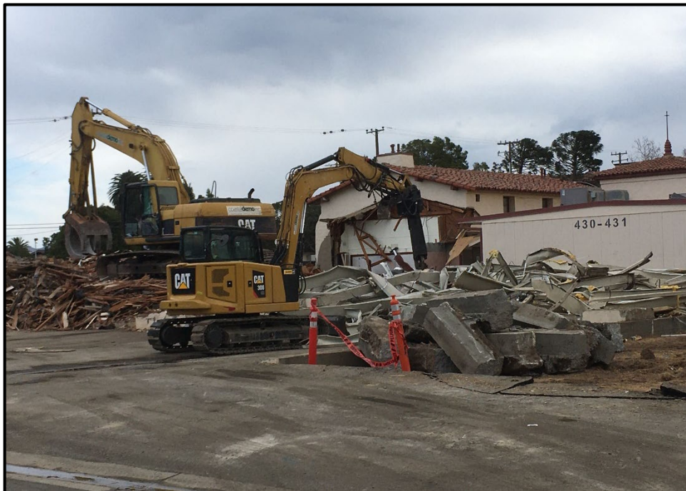
SMHS 50-Classroom Building – Demolition Begins in Earnest
