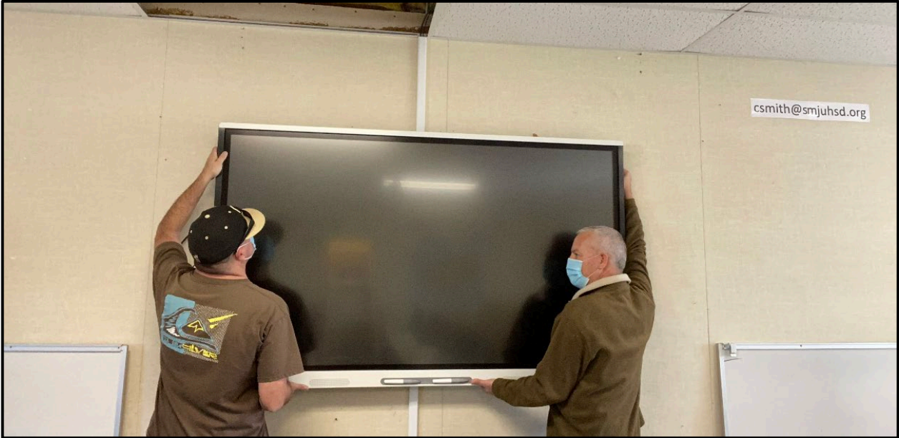
... The Electricians Make the Finished Product Look Easy
