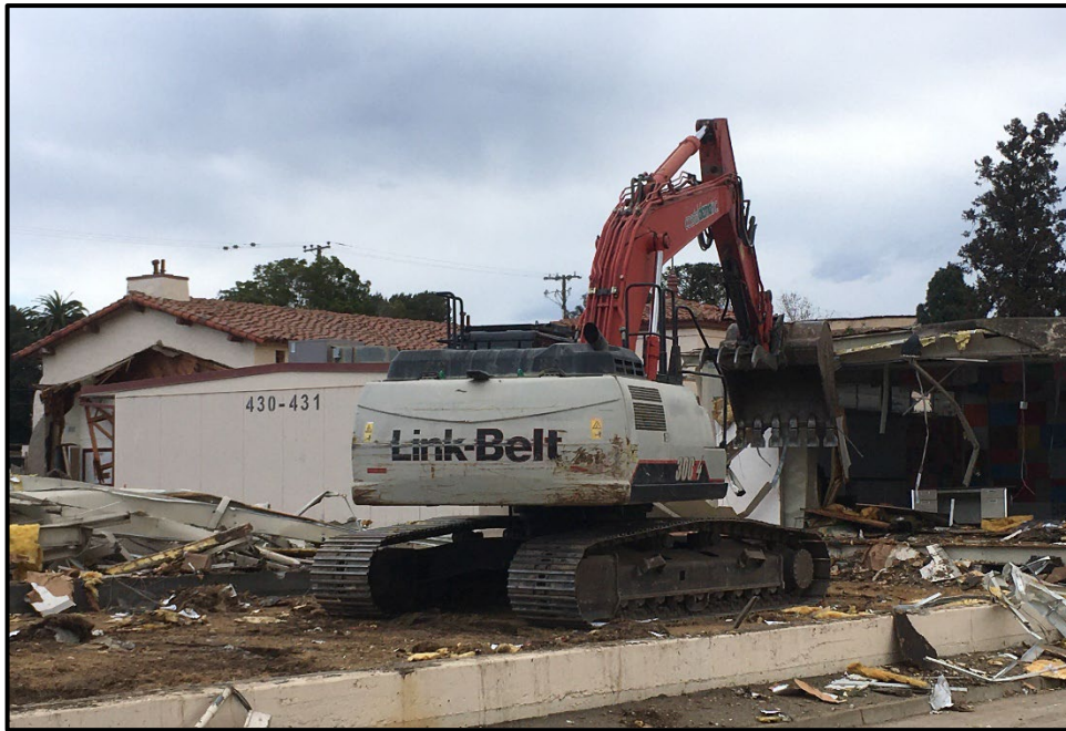
SMHS 50-Classroom Building – Demolition is Underway
