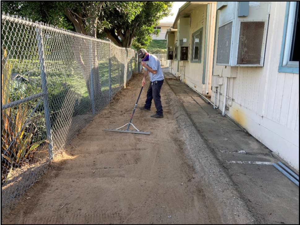
ERHS – Jordan Markstone Prepares the Ground for Rubber Mulch Behind Portable Classrooms
