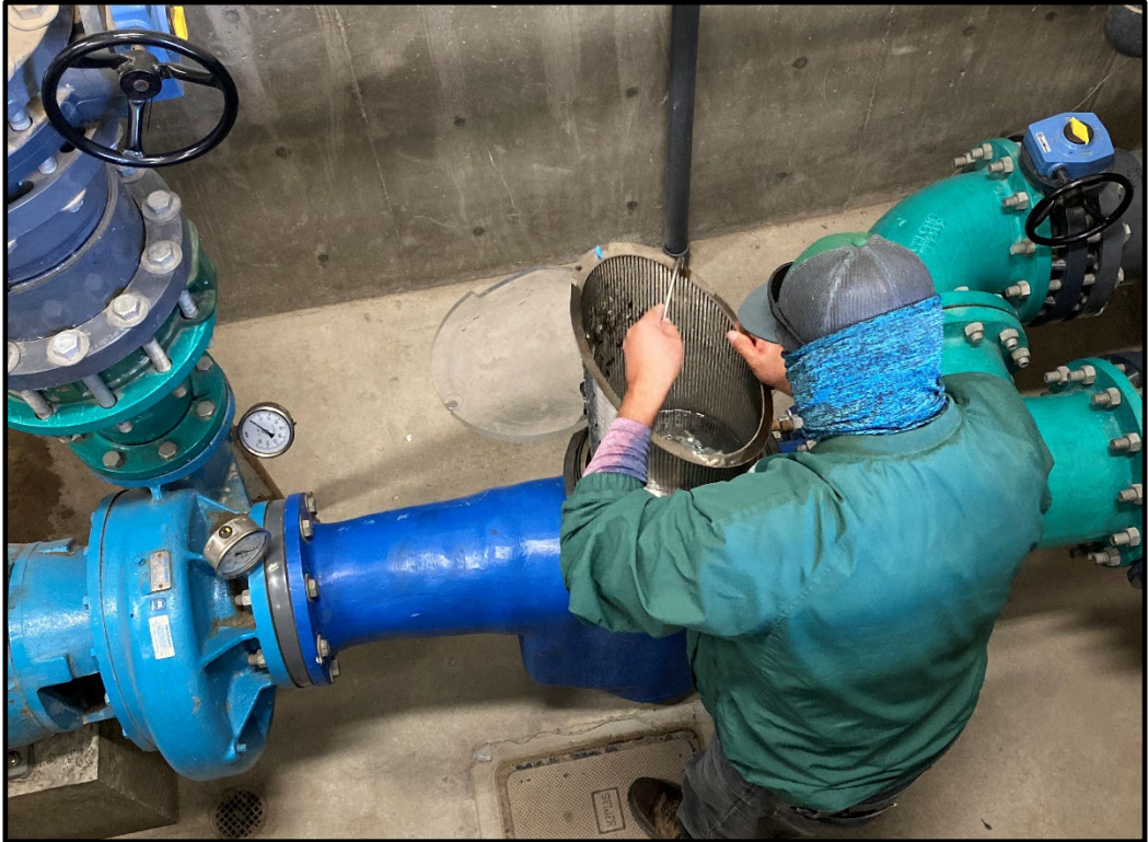
PVHS – City Pool Operator Cleans the Recirculating Pump Filter
