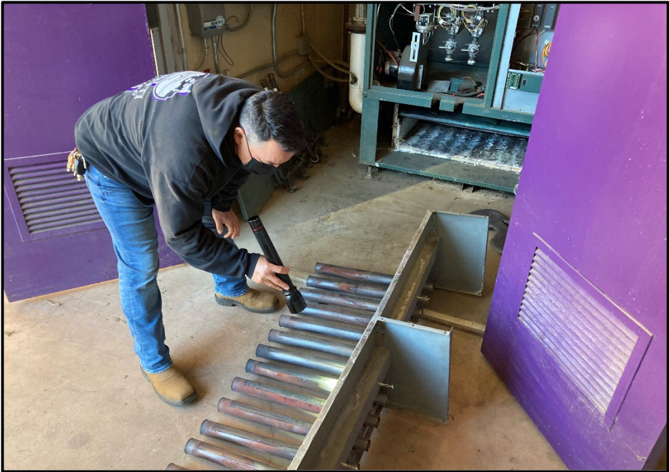
ERHS – Bernie Rayner Inspects the Heating Boiler Burners During a Preventive Maintenance Service
