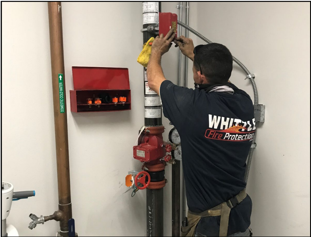
PVHS – Fire Riser Control Valve is Replaced in the Cafeteria
