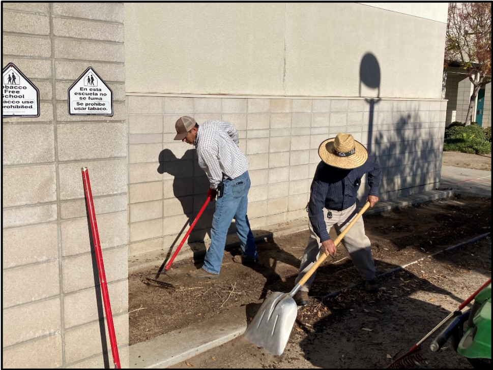
PVHS – José Gamino and Pepé Gutierrez Renovate the Planters at the Gymnasium
