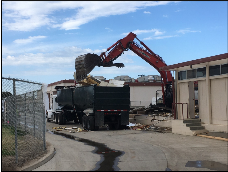
SMHS 50-Classroom Building – The First Truckloads Leave the Campus!
