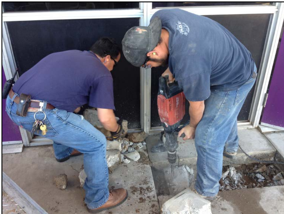
ERHS – Bernie Rayner & Flavio Rodriguez Repairing a Broken Water Line at the Gymnasium
