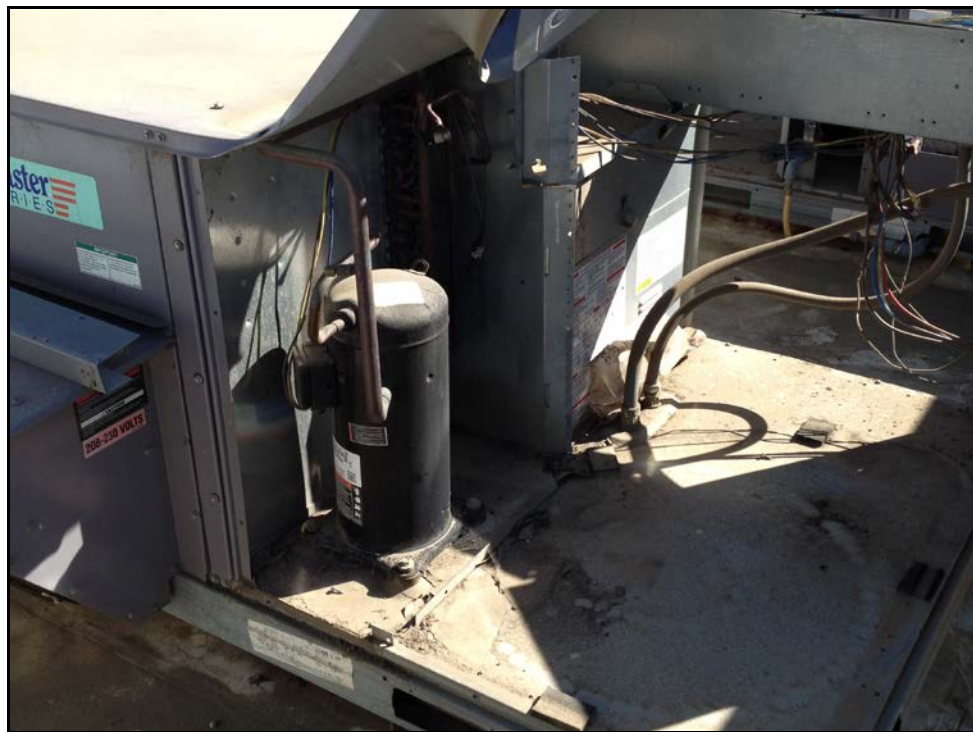
SMHS – Second Round of Copper Stolen From Rooftop HVAC Units
