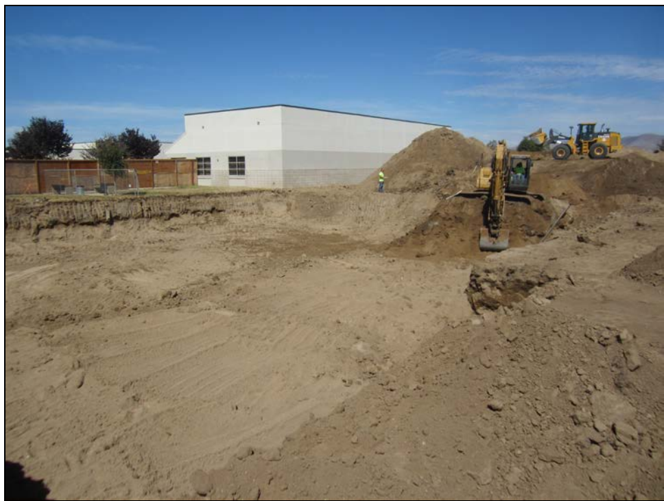
PVHS – Performing Arts Center Excavation and Utility Work Underway
