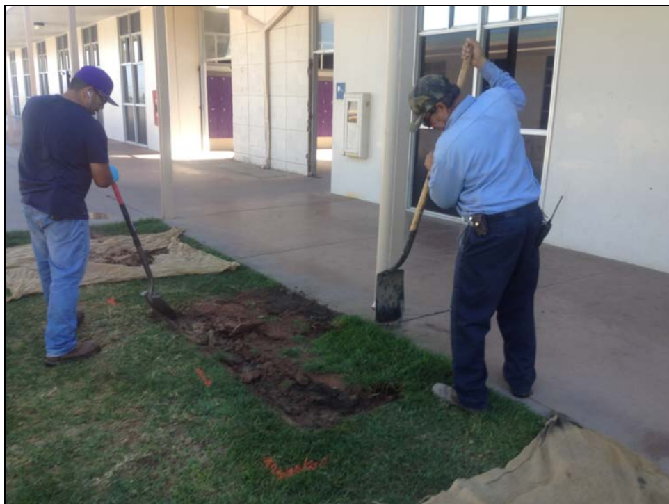
ERHS – Nelson Frutos and Juan Rodriguez prepare a new rain gutter drainage area
