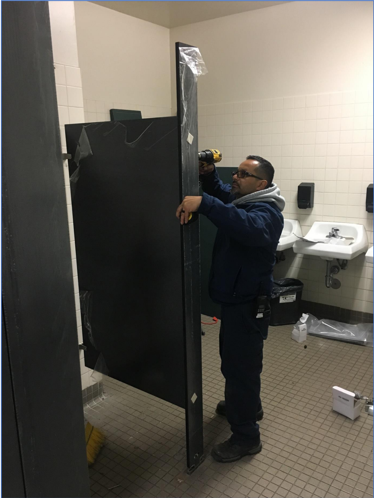
ERHS – Jimmy Salutan Replaces a Damaged Restroom Partition
