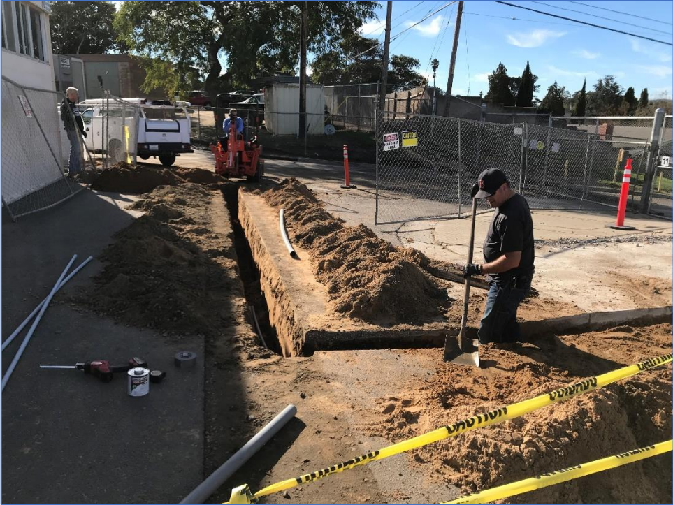
ERHS – District Maintenance Crew Excavates for Power to New Ag Science Cooler
