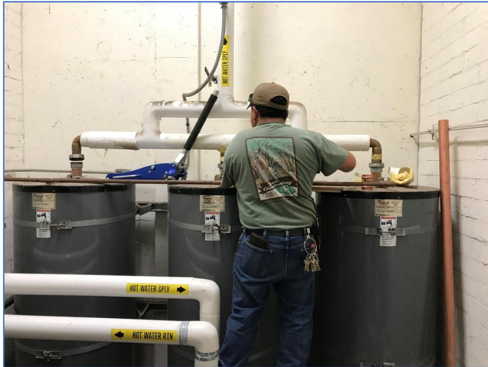
PVHS – Jesus Reyes Repairs a Water Leak on the Gymnasium Water Heaters
