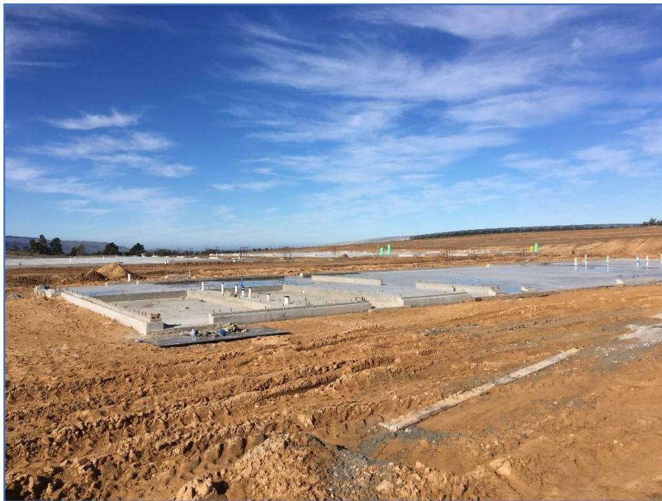
CTE Ag Center – Culinary Arts Floor Slab is Poured and Curing
