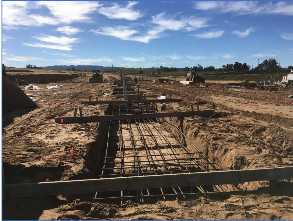
CTE Ag Center – The Barn Footings are Massive
