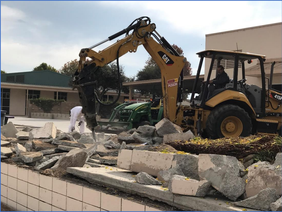
ERHS – José Placencia and Ernest Paz Clear Concrete from the Quad Planter
