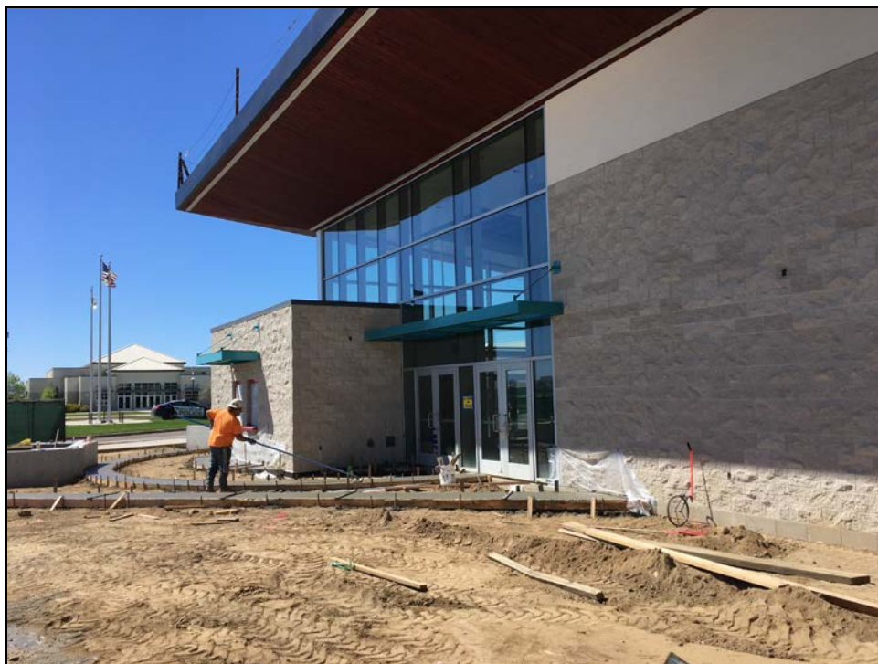
PVHS Performing Arts Center – Exterior Walkways are Taking Shape
