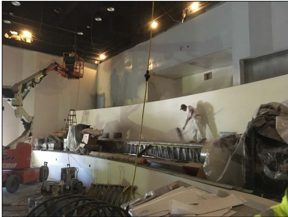
PVHS Performing Arts Center – Interior Painting and Electrical Work Underway
