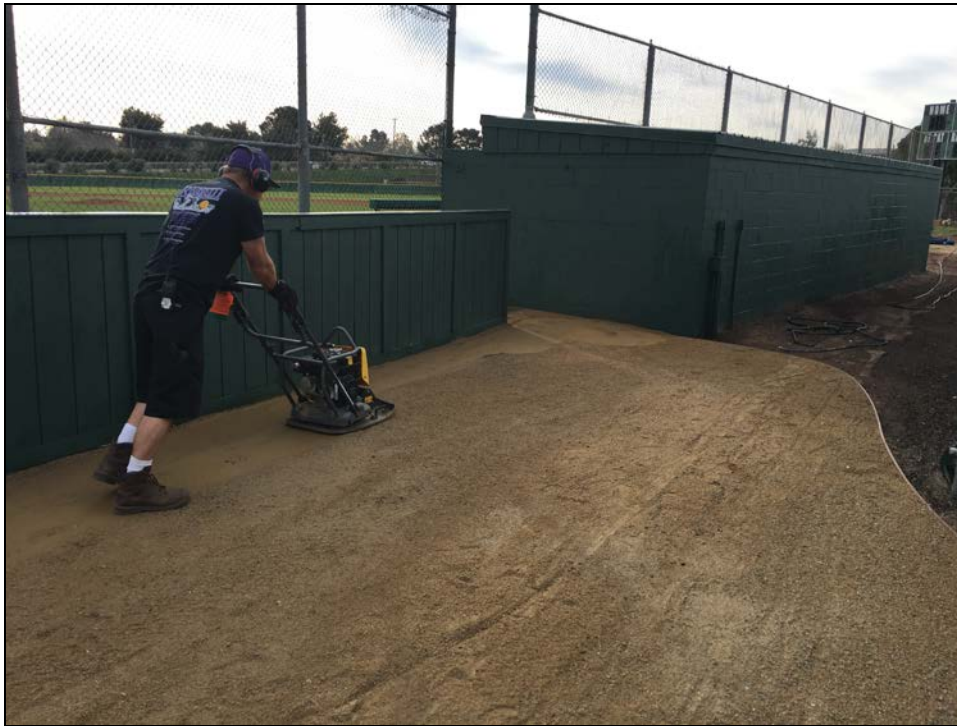
ERHS - Denton Tilley Compacts the Walkway to Varsity Baseball Bleachers
