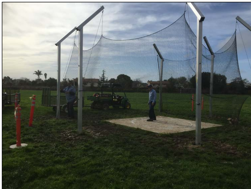
ERHS – Pepé Gutierrez and Elias Comacho Install a Safety Cage at the Discus Pad
