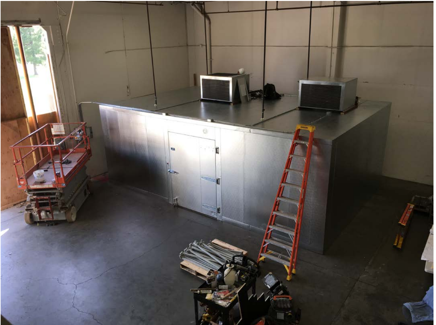
Support Services Center – New Efficient Freezer Replaces Two Older Units for Food Service Program
