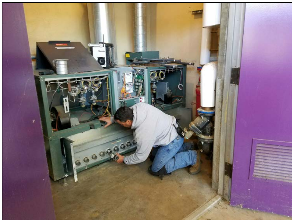
ERHS - Bernie Rayner Services a Heating Boiler
