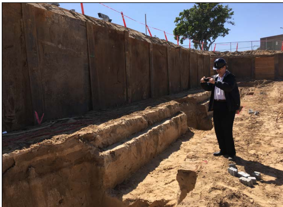
ERHS 38 Classroom Building – Architect Placed for Perspective on the Size of Footings
