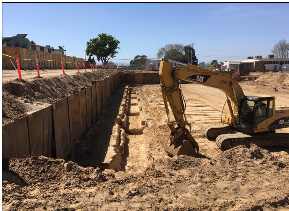
ERHS 38 Classroom Building – Excavation for Footings Underway
