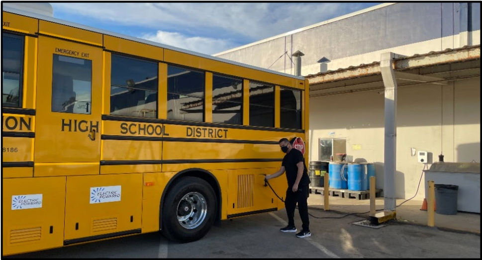
SSC – Mark Cabatuan Plugs in Electric Bus 007 with the New Charger
