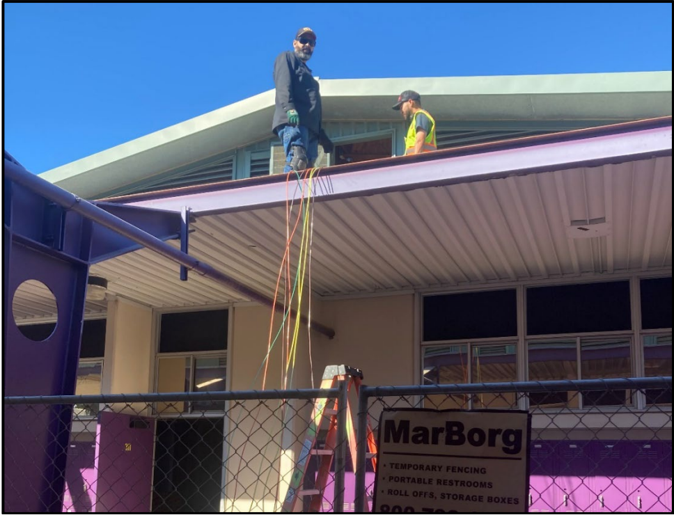
ERHS Modernization – New Electrical Feeder Wire is Installed in the Attic
