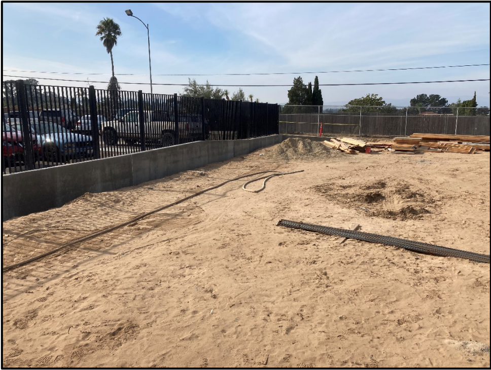
ERHS Maintenance and Operations Building – Retaining Wall is Complete
