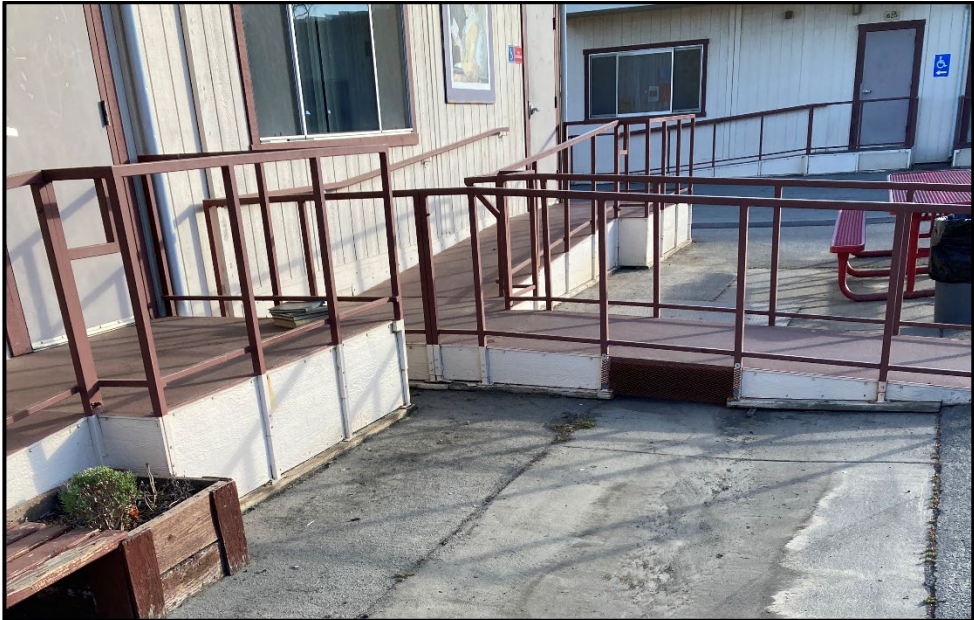
SMHS – Improved Storm Water Drainage Under Portable Ramps
