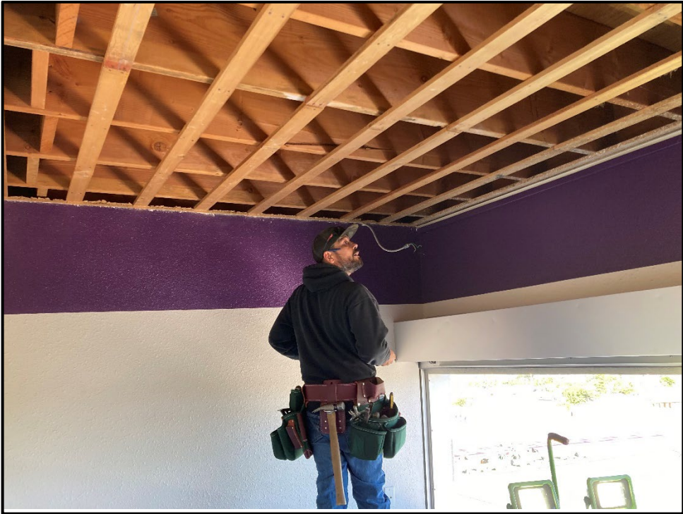
ERHS – Tom Harbold Installs Drywall Inside the Stadium Press Box
