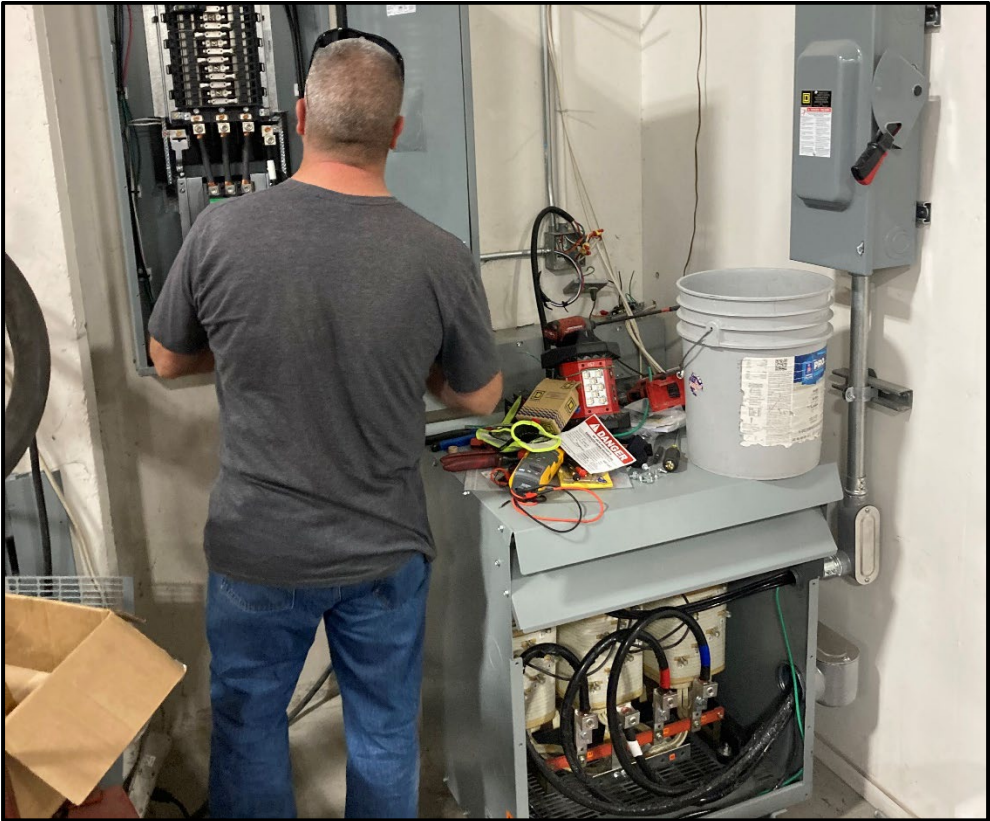
Transportation – Andy Freitas Installs a New Electric Transformer and Panel to Charge Buses
