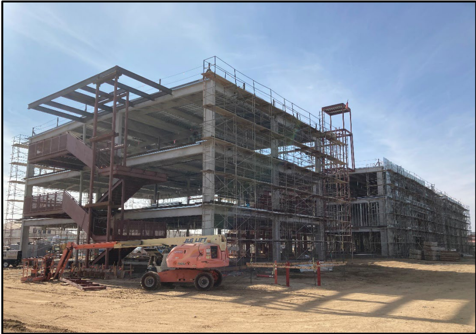
SMHS 50-Classroom Building – View of the Front of the Structure and the Bell Tower
