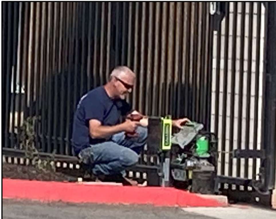
PVHS-Gates – Del Ward Installs Five Remote Operated Openers for Electric Gates
