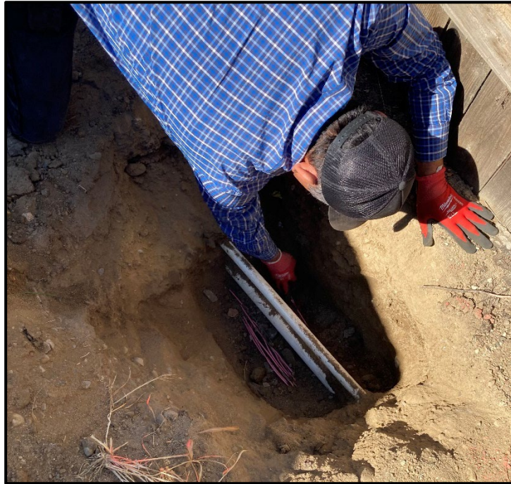
PVHS- Jose Gamino Repairs a Broken Irrigation Communication Line
