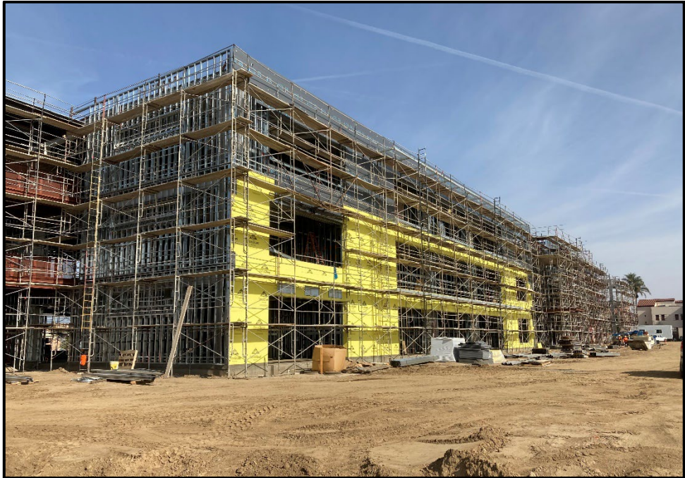
SMHS 50-Classroom Building – Scaffolding is in Place for Exterior Work
