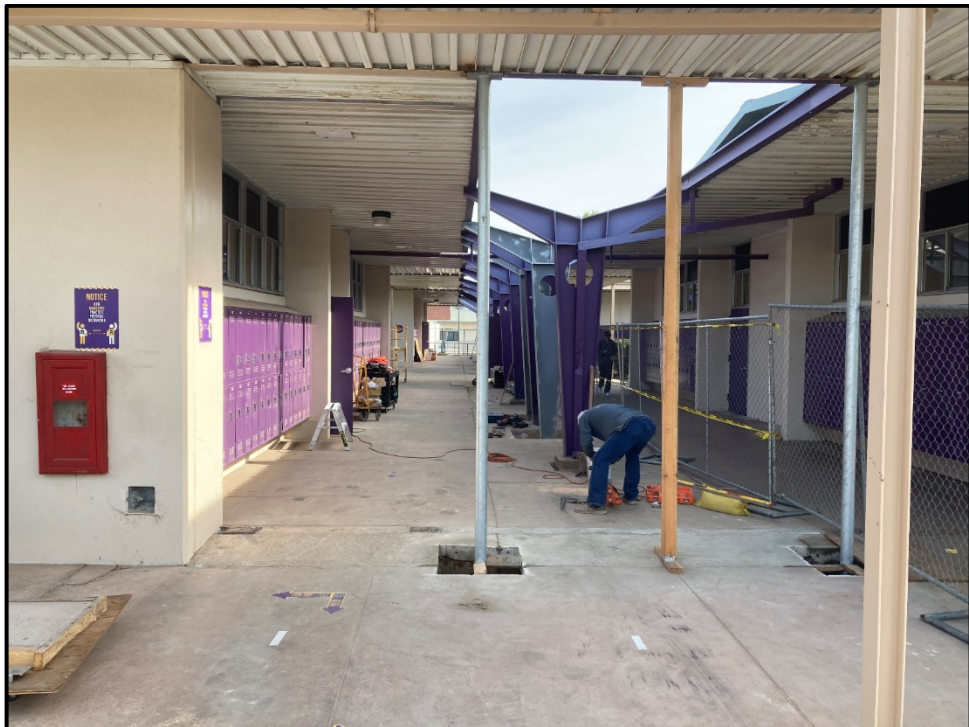
ERHS Modernization- New Columns Support HVAC on Walkway Roofs
