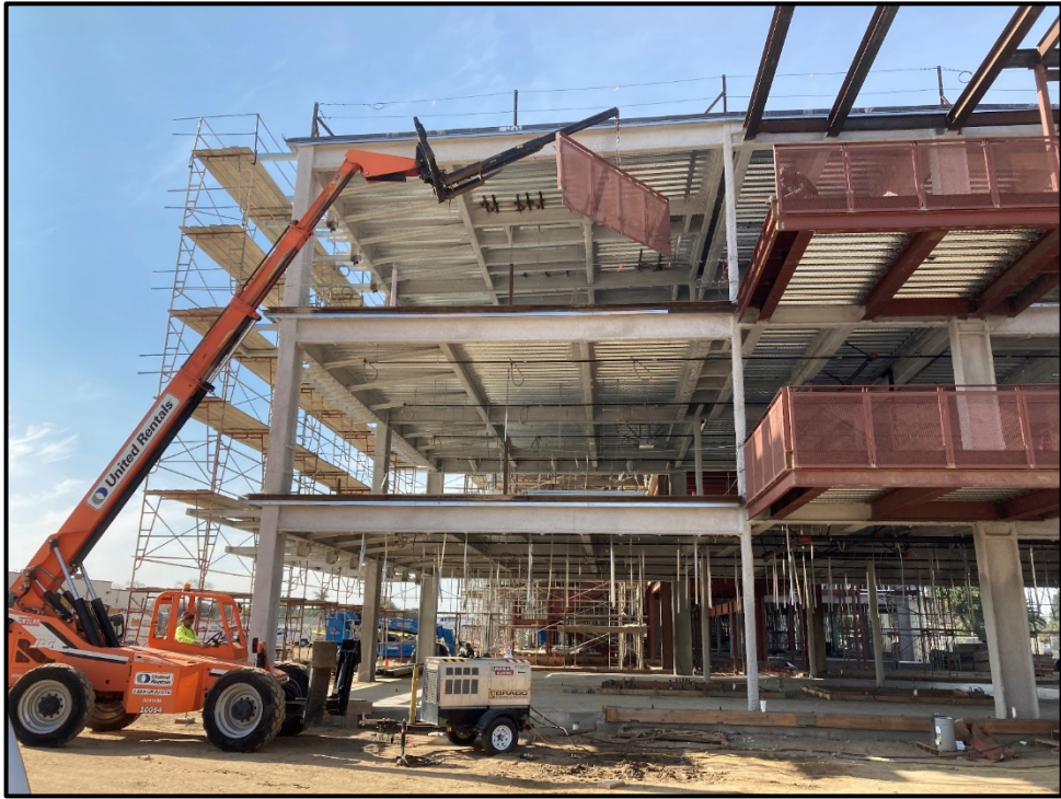
SMHS 50-Classroom Building – Exterior Stairway Assembly is In Progress
