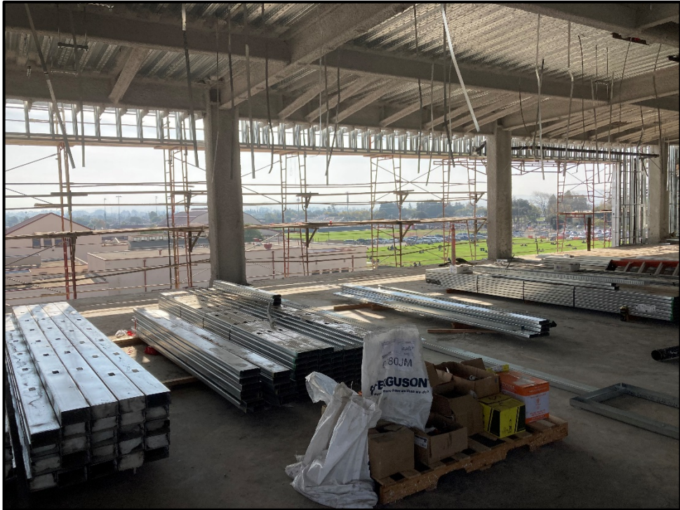
SMHS 50-Classroom Building – Third Story Looks Over the Existing Campus
