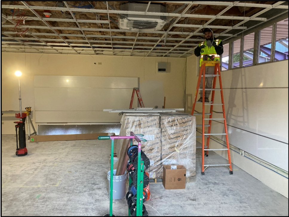
ERHS Modernization – New Ceiling T-Bar is in Place
