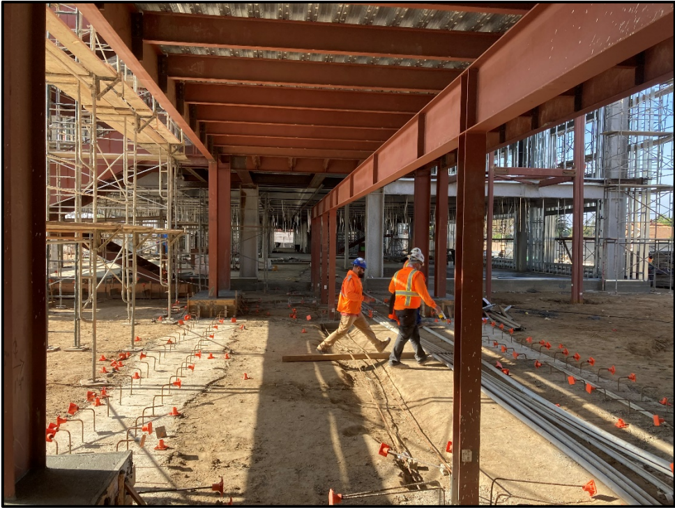
SMHS 50-Classroom Building – Ground Floor Entrance is Ready for Concrete
