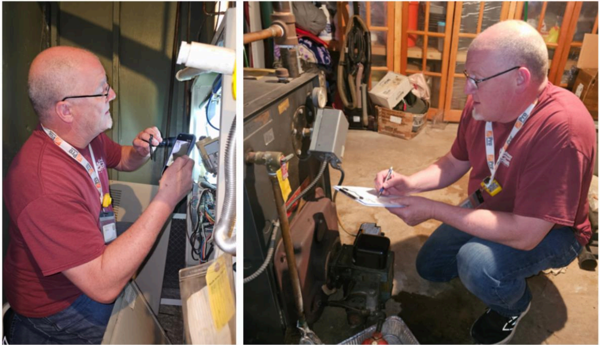
Energy Auditor John Smythe conducts key home-safety and efficiency checks, including combustion testing a heating system and documenting system information to ensure accurate assessments and safe operation.
