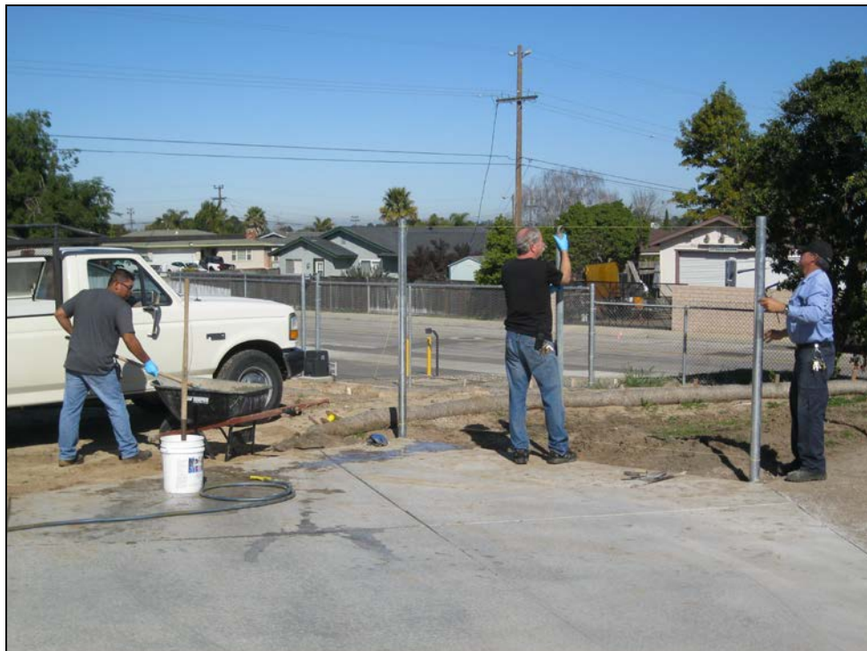
ERHS - Building Fencing at the Football Stadium & Greenhouse Area
