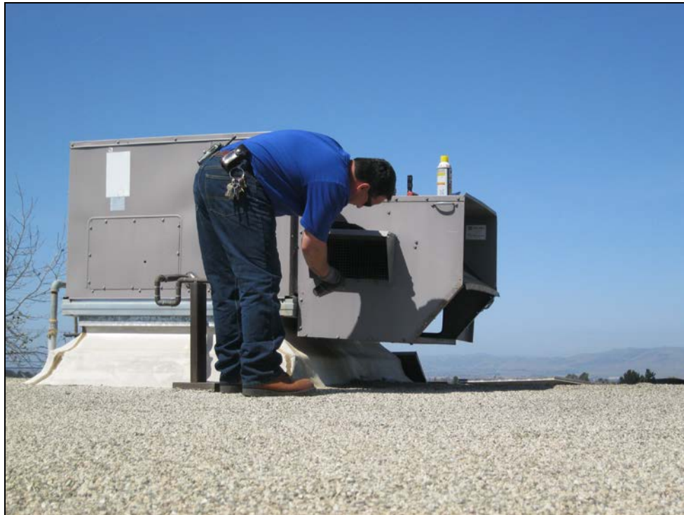
ERHS – Preventive Maintenance on a Roof Top Heating Unit (great view of the valley)
