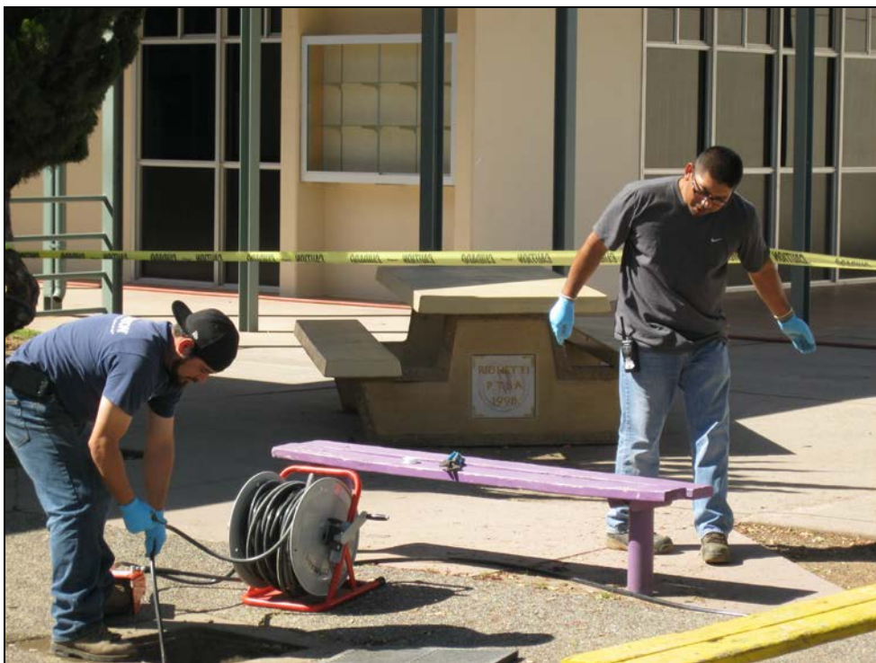
ERHS - Cleaning Storm Drains on Campus
