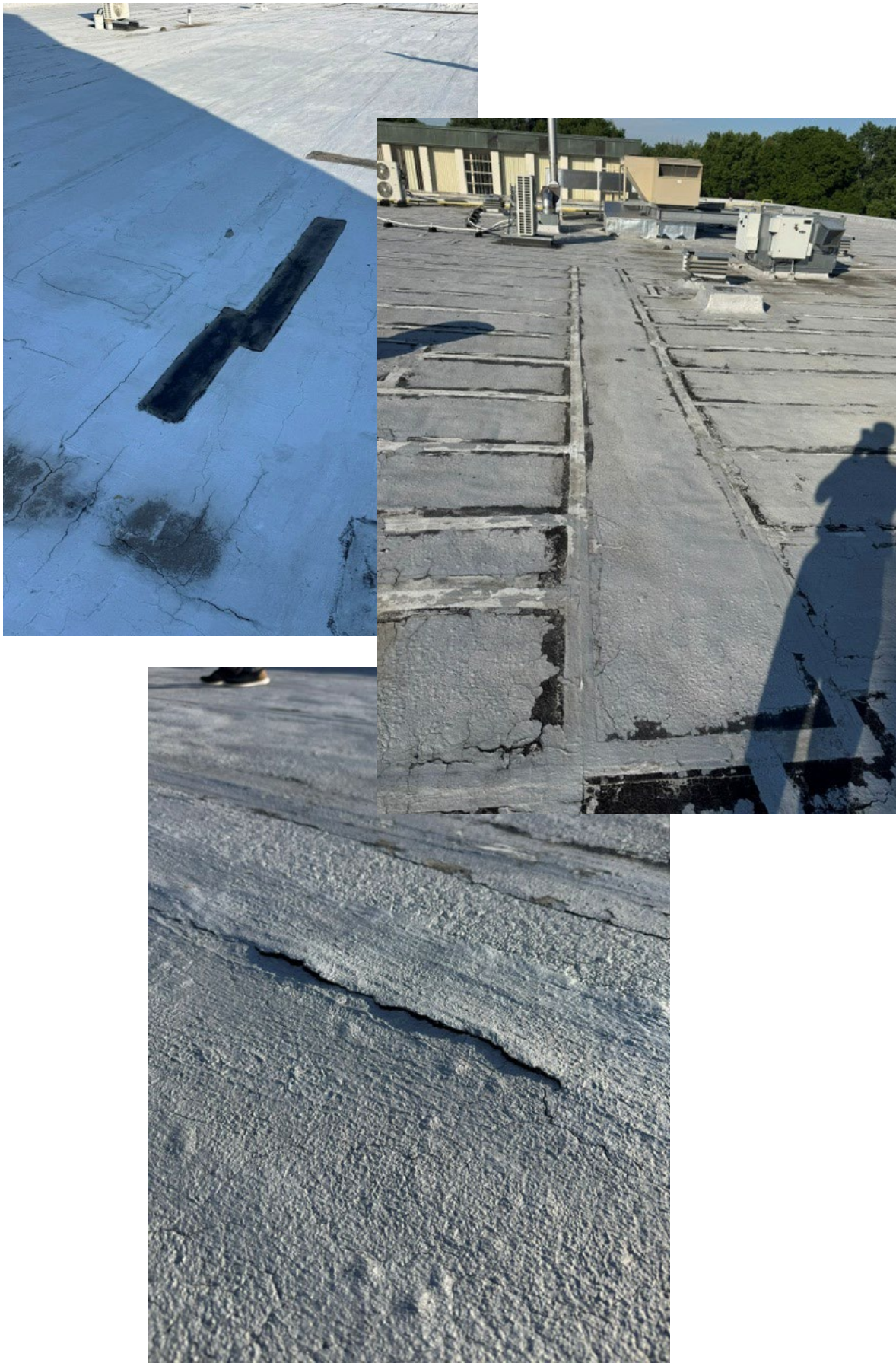
Northeast Middle School Roof
