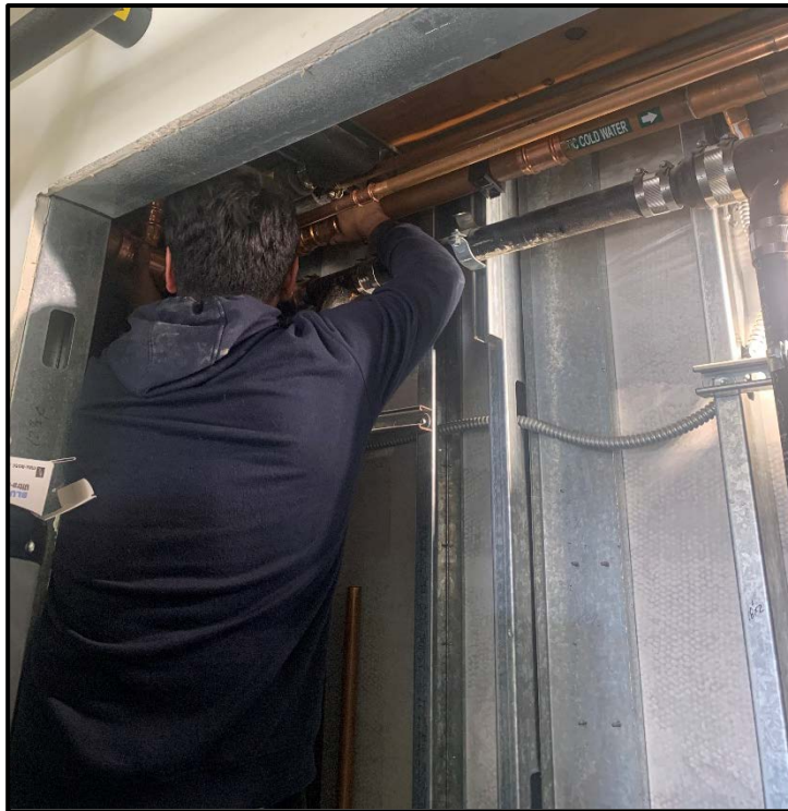
SMHS – John Daniloff Repairs a Water Leak in the Pool Equipment Room
