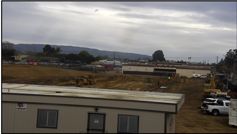
...Next you Put All the Dirt Back in the Hole and Compact it...
