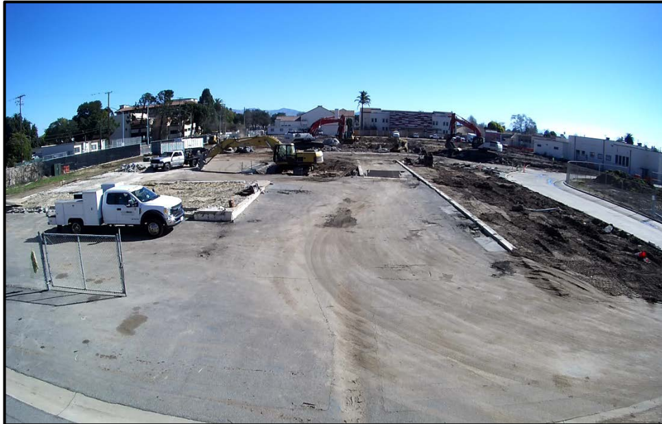
SMHS 50-Classroom Building – First you Demolish the Old Buildings...
