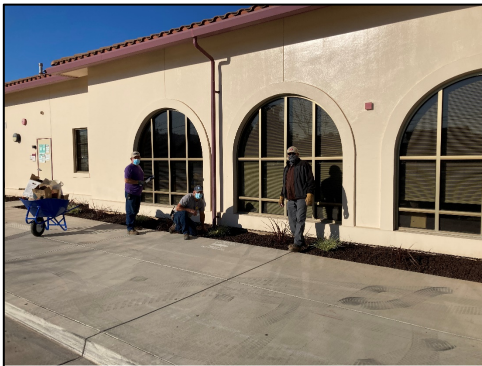
DHS – The Grounds Crew Puts the Finishing Touches on the Entry Planter
