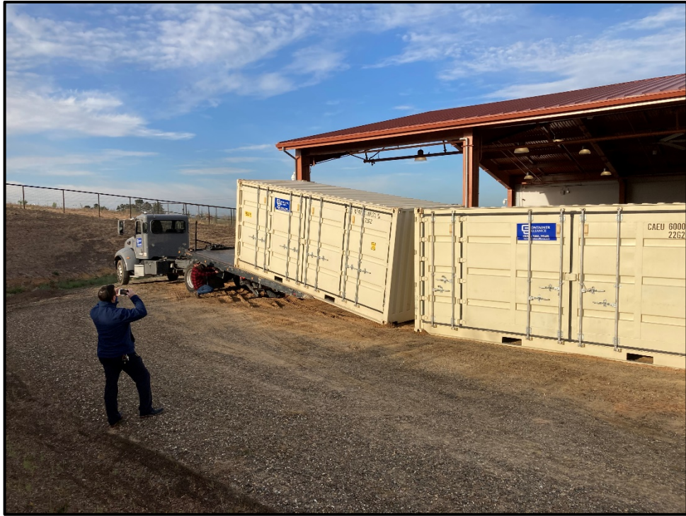
CTE Center – Paul Robinson Oversees Storage Unit Placement
