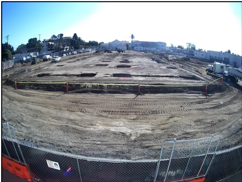
...and Finally, You Dig New Holes for the Footings!
