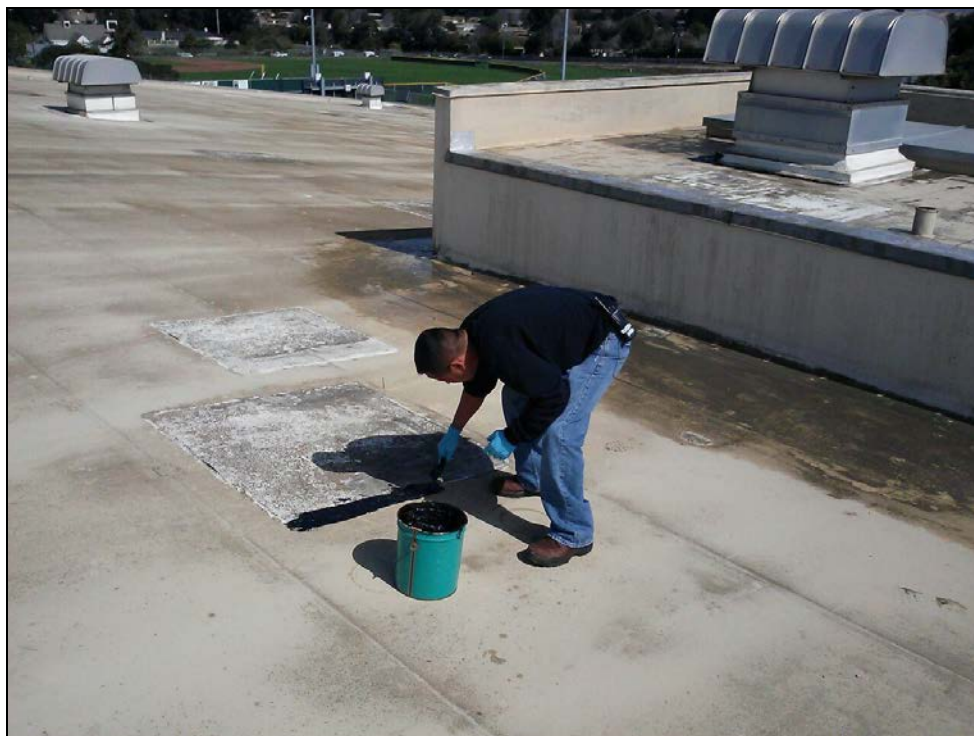
ERHS – Jimmy Salutan Makes Temporary Repairs to the Gymnasium Roof
