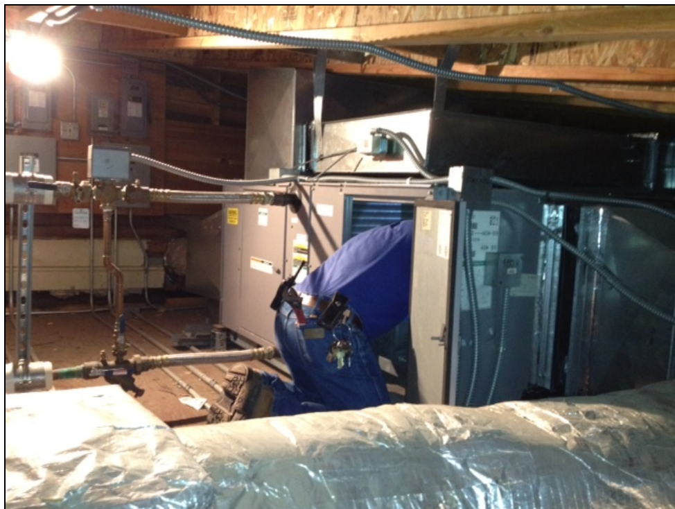
ERHS – Bernie Rayner Replaces Heater Filters in the Attic Crawl Space
