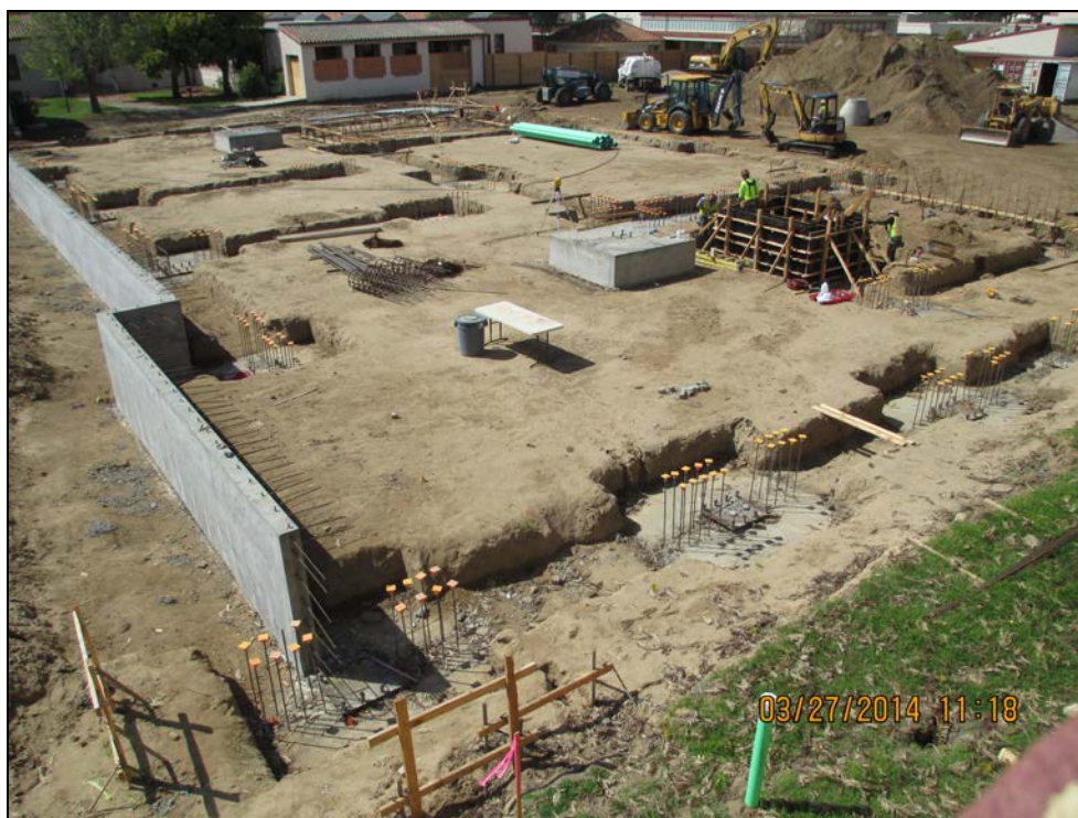
SMHS - 14 Classroom Building Elevator Pit Takes Shape
