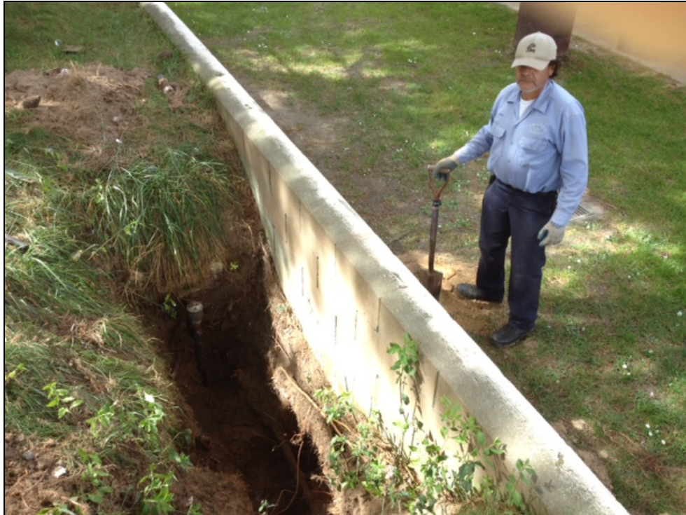
ERHS – Juan Rodriguez Uncovers an Irrigation Valve Buried Behind a Retaining Wall
