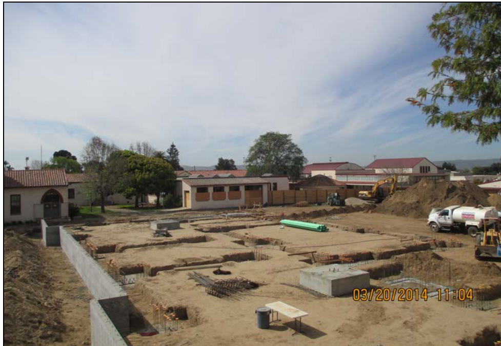
SMHS - 14 Classroom Building Concrete Reinforcing Bars & Elevator Footings
