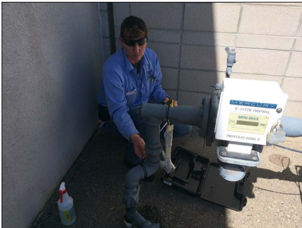
PVHS – Jennifer Abend Checks the Main Natural Gas Valve
