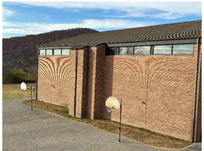
Exterior Brick & Concrete Block walls – sloped roof B
