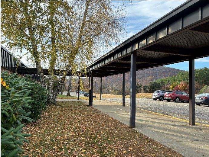
Can Canopy of North side of Building
