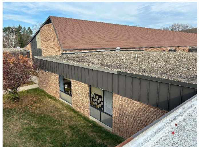
low slope roof 4 (note standing seam metal fascia panel)
