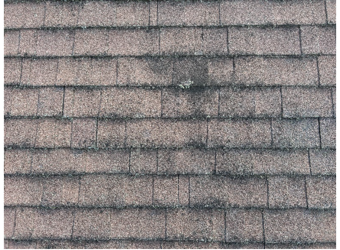
Typical condition of sloped asphalt shingle roofs
