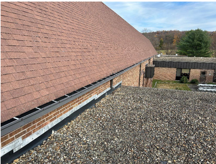
Exterior Brick & Concrete Block walls – sloped roof A
