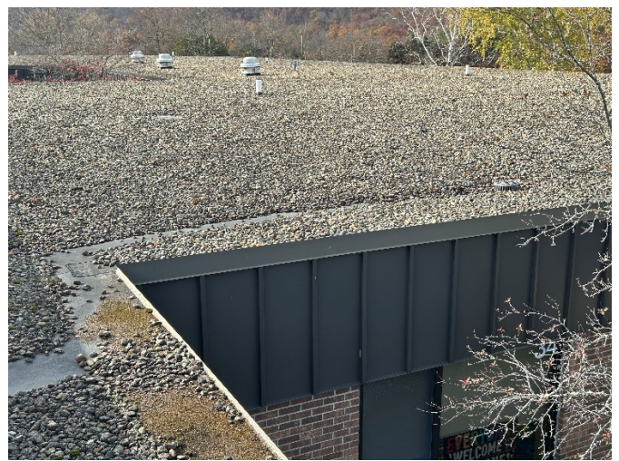
typical condition of low sloped ballasted membrane
