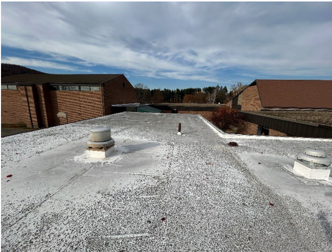
Roof f5, low slope single ply membrane roof
